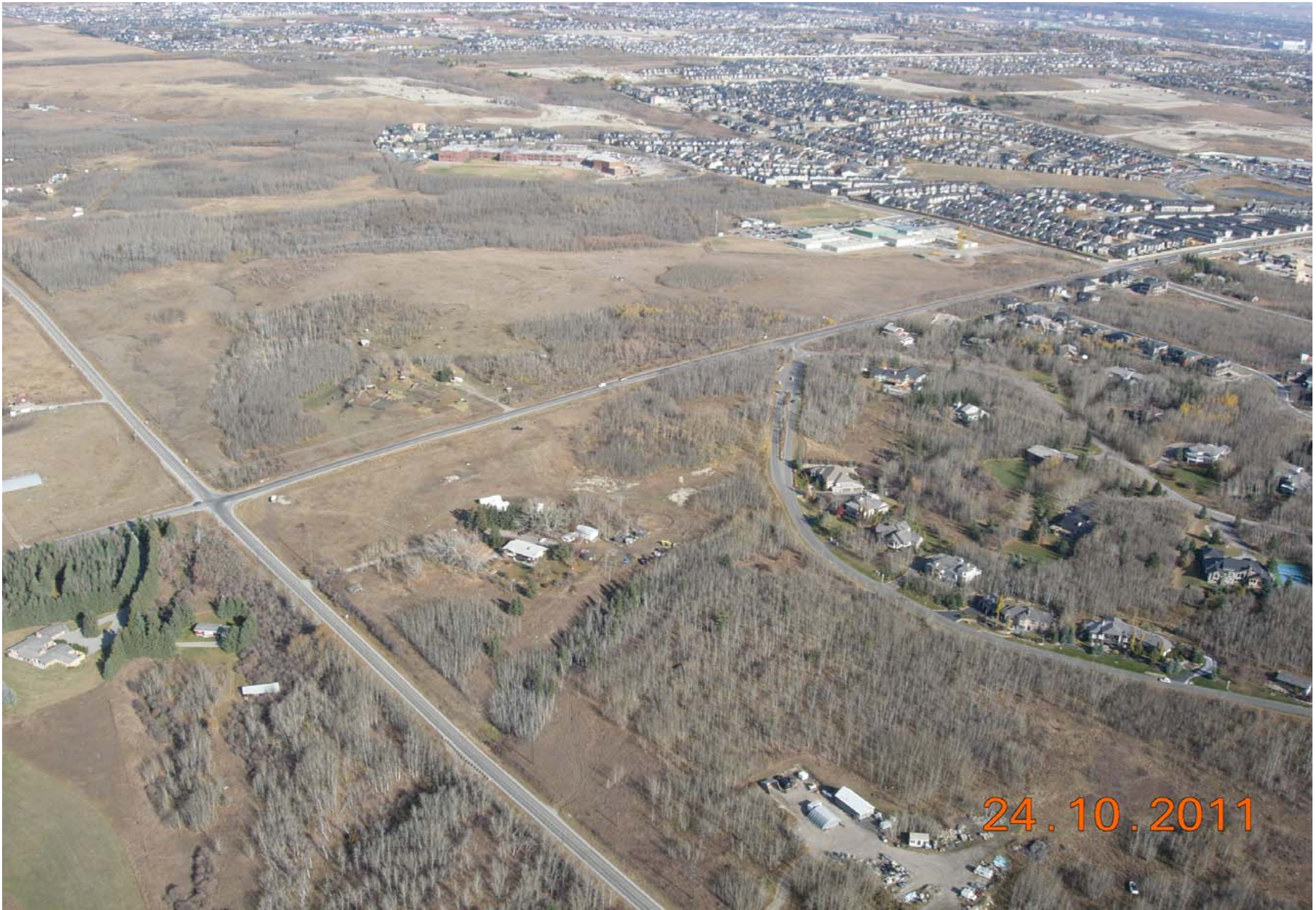
Stoney Trail / 17th Avenue SW Interchange Looking Northeast October 2011
