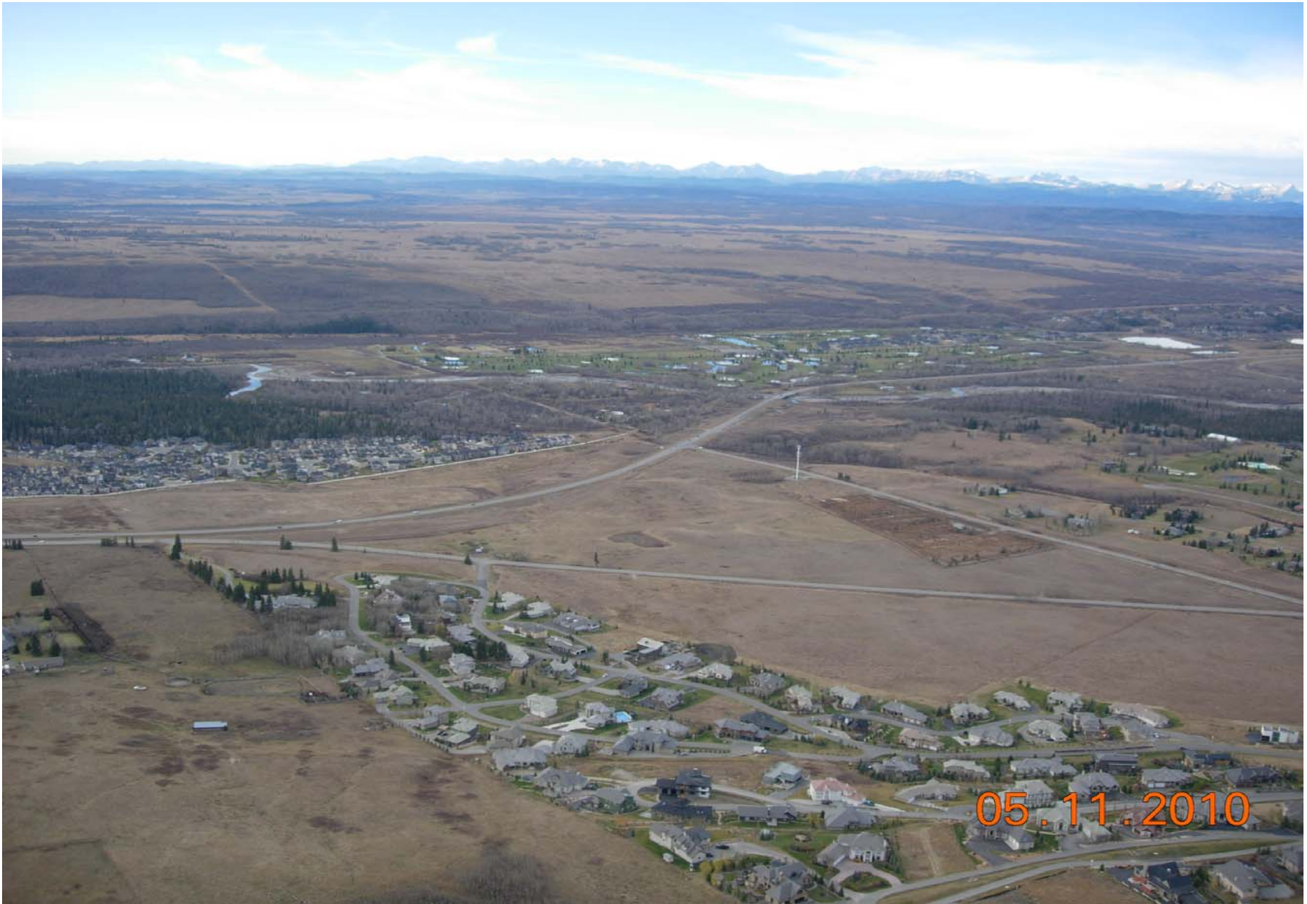
Stoney Trail / Glenmore Trail Interchange Looking Southwest November 2010
