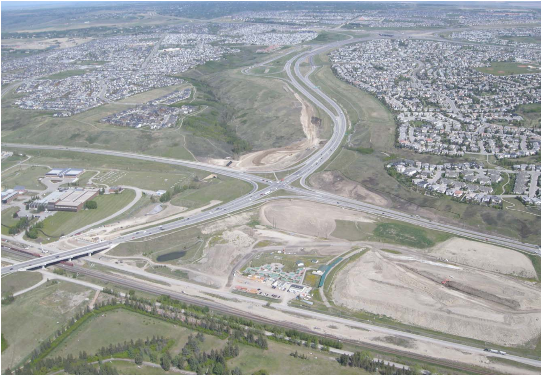
Stoney Trail / Nose Hill Drive Interchange Looking Northwest May 2012
