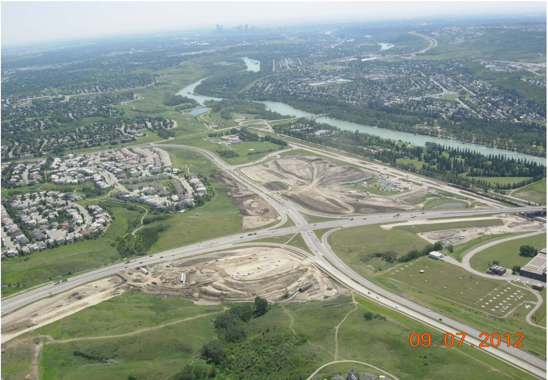
Stoney Trail / Nose Hill Drive Interchange Looking Southeast July 2012
