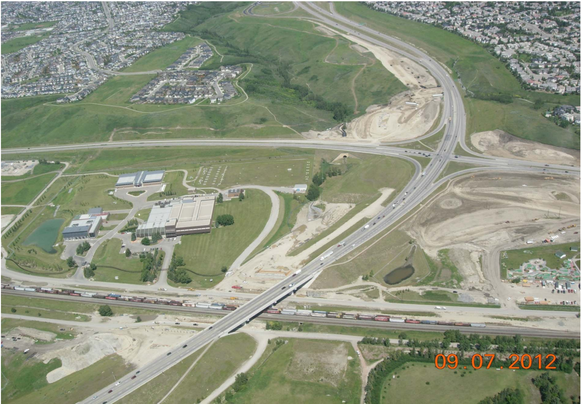
Stoney Trail / Nose Hill Drive Interchange Looking Northwest July 2012
