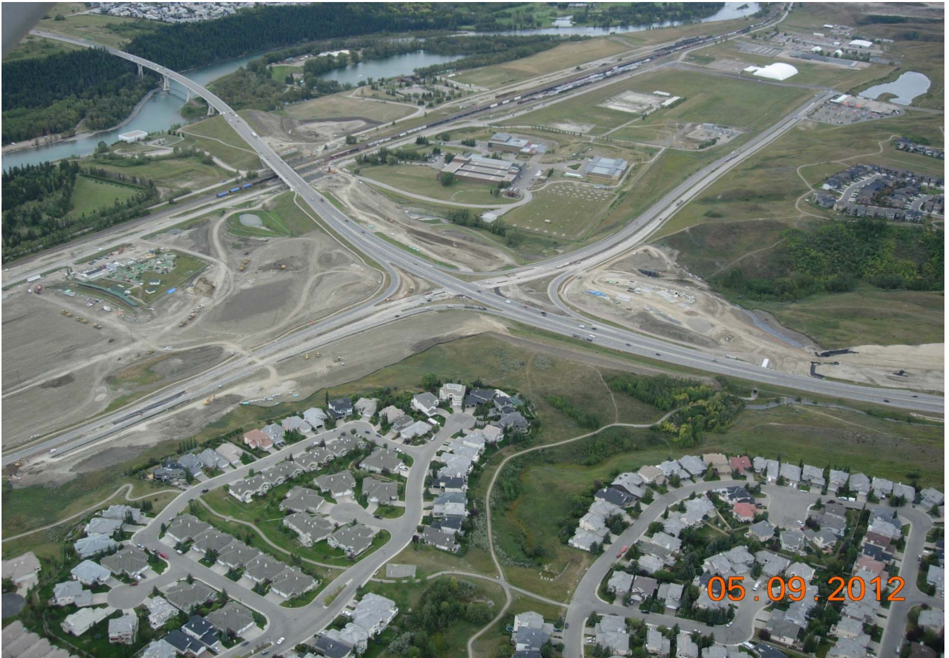
Stoney Trail / Nose Hill Drive Interchange Looking Southwest September 2012
