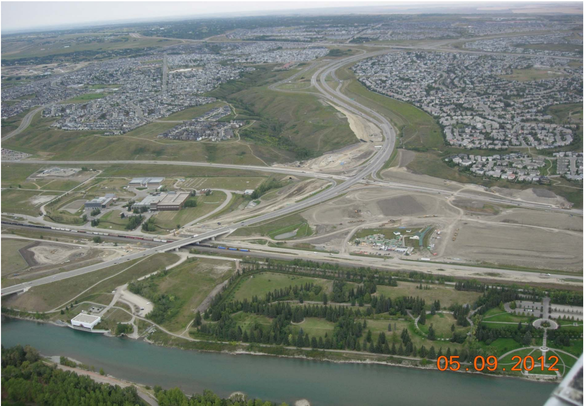
Stoney Trail / Nose Hill Drive Interchange Looking Northwest September 2012
