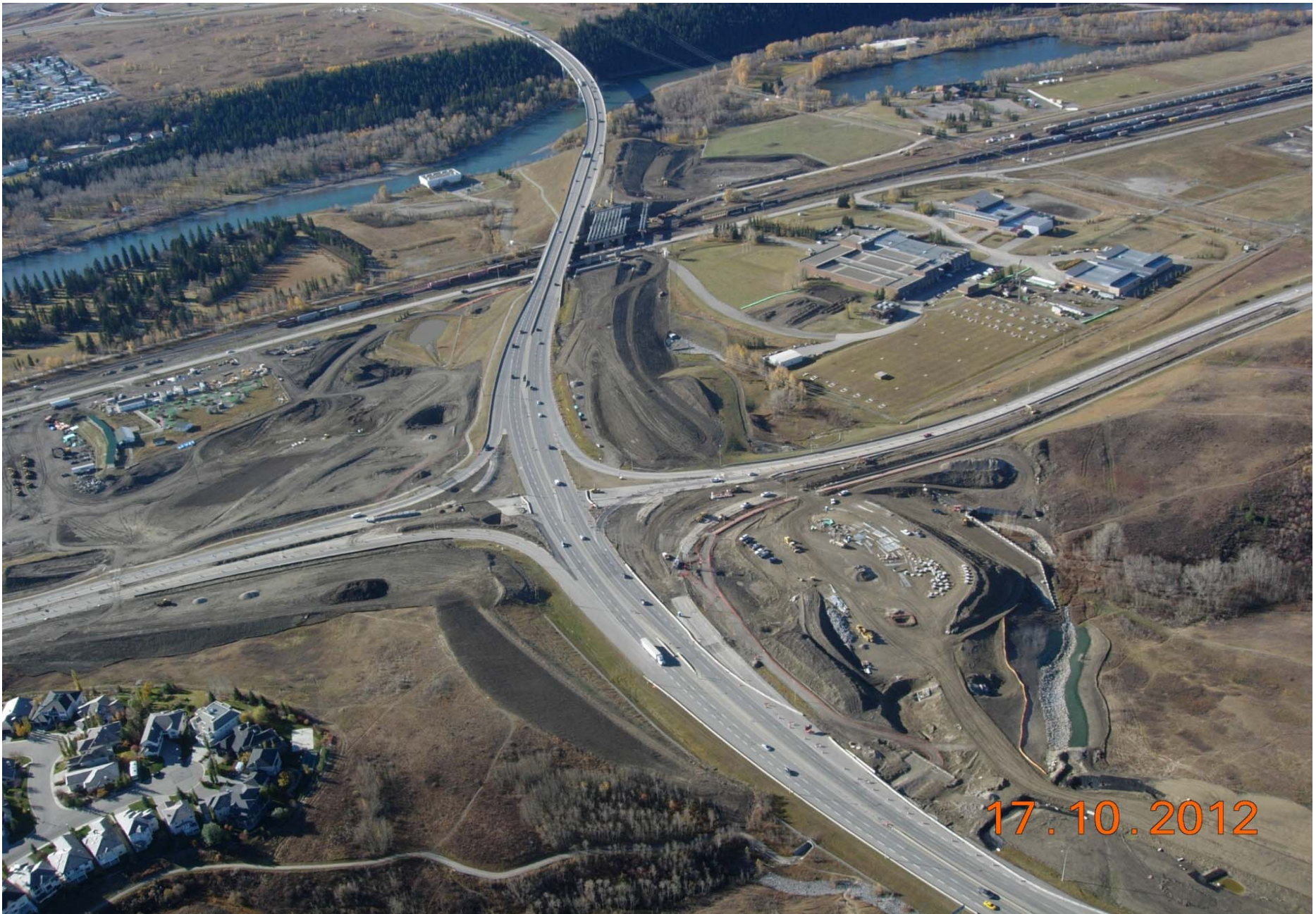
Stoney Trail / Nose Hill Drive Interchange Looking Southwest October 2012
