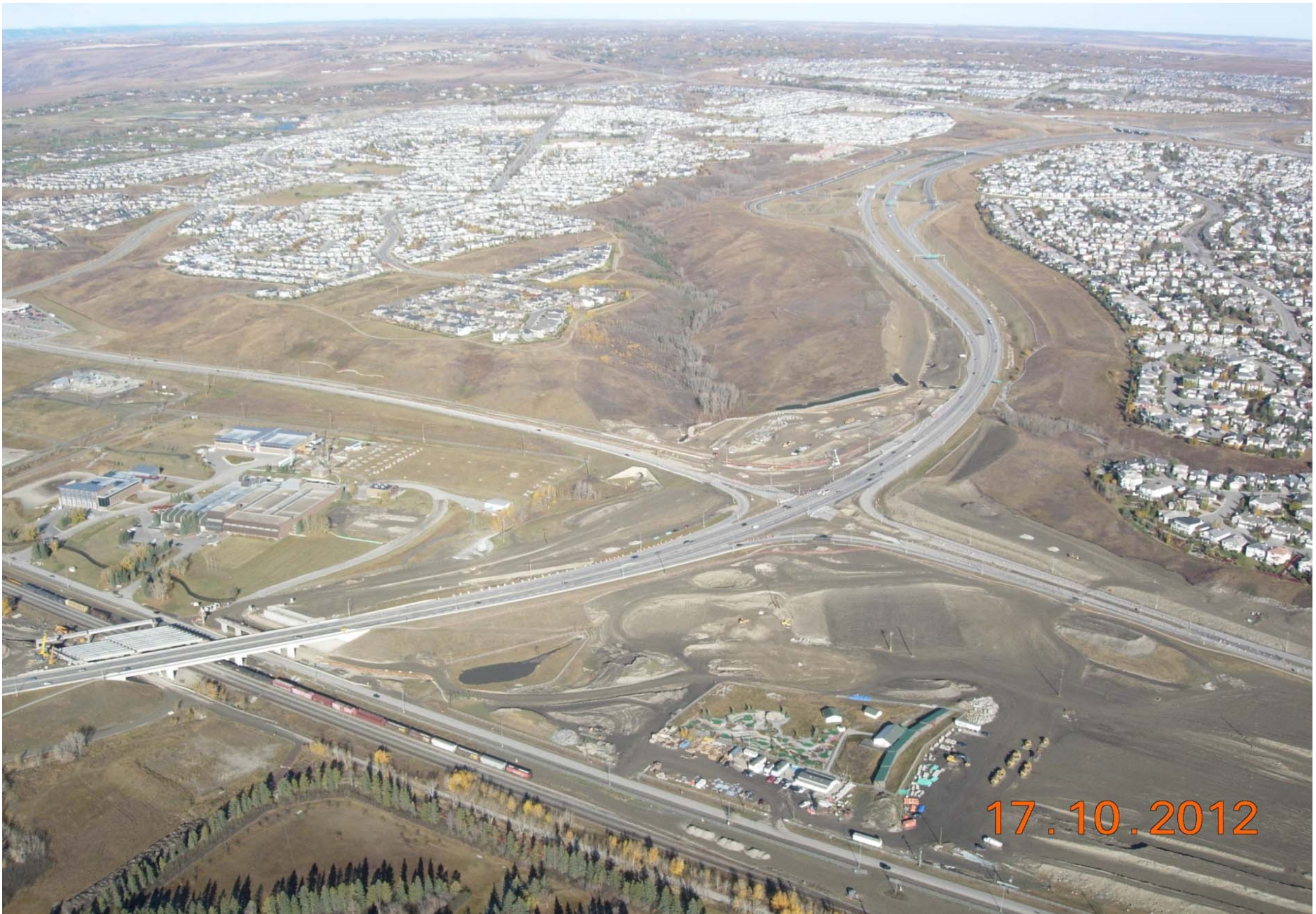
Stoney Trail / Nose Hill Drive Interchange Looking Northwest October 2012
