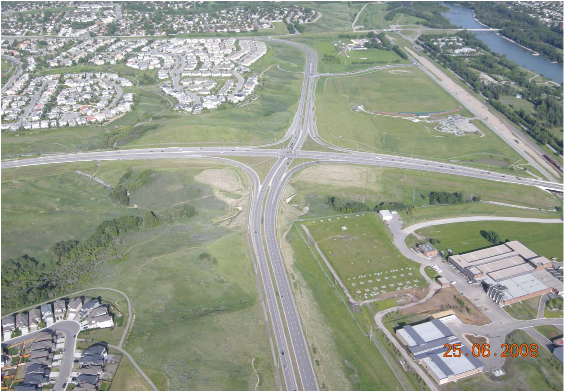
Stoney Trail / Nose Hill Drive Interchange Looking East June 2008
