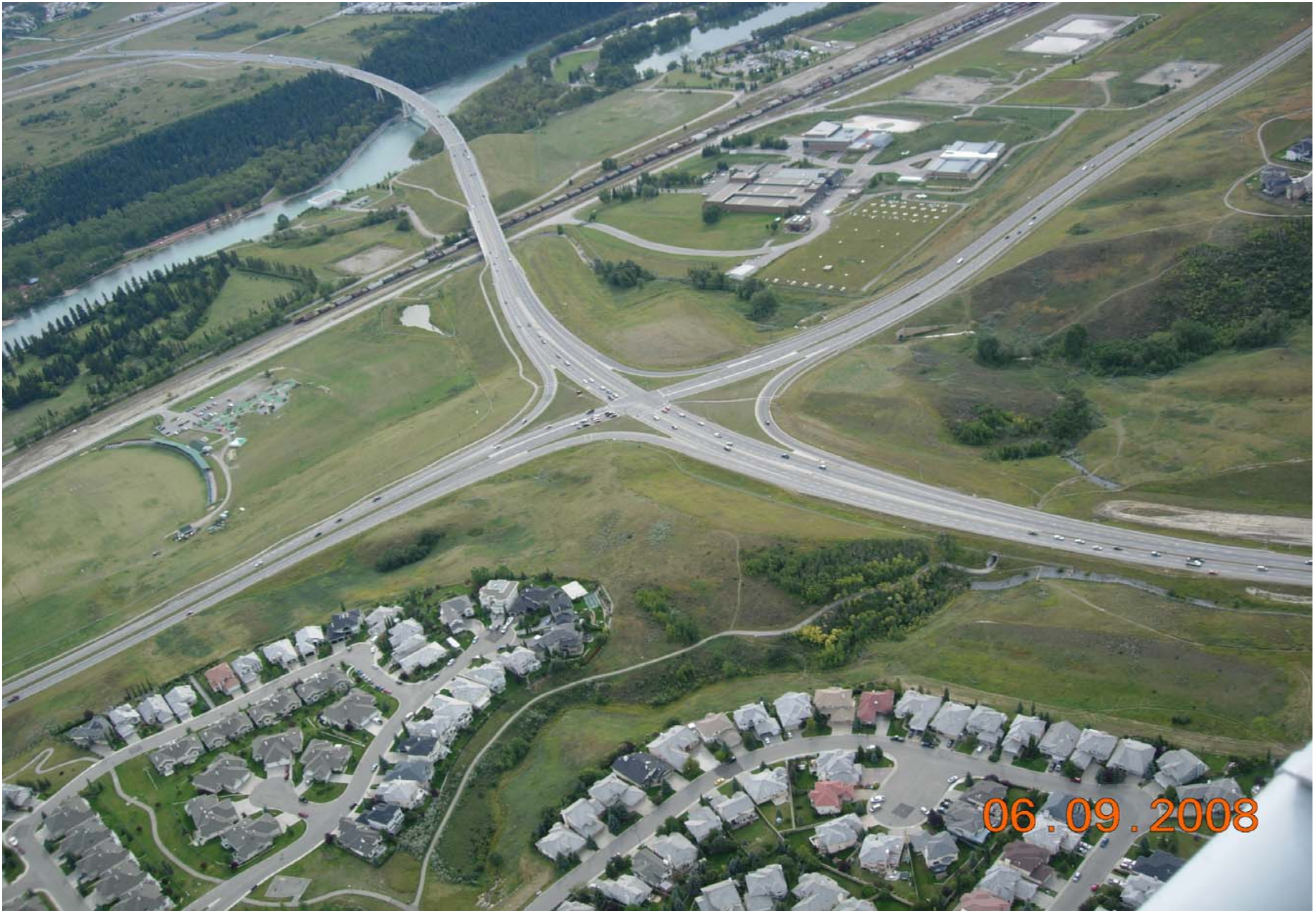
Stoney Trail / Nose Hill Drive Interchange Looking Southwest September 2008
