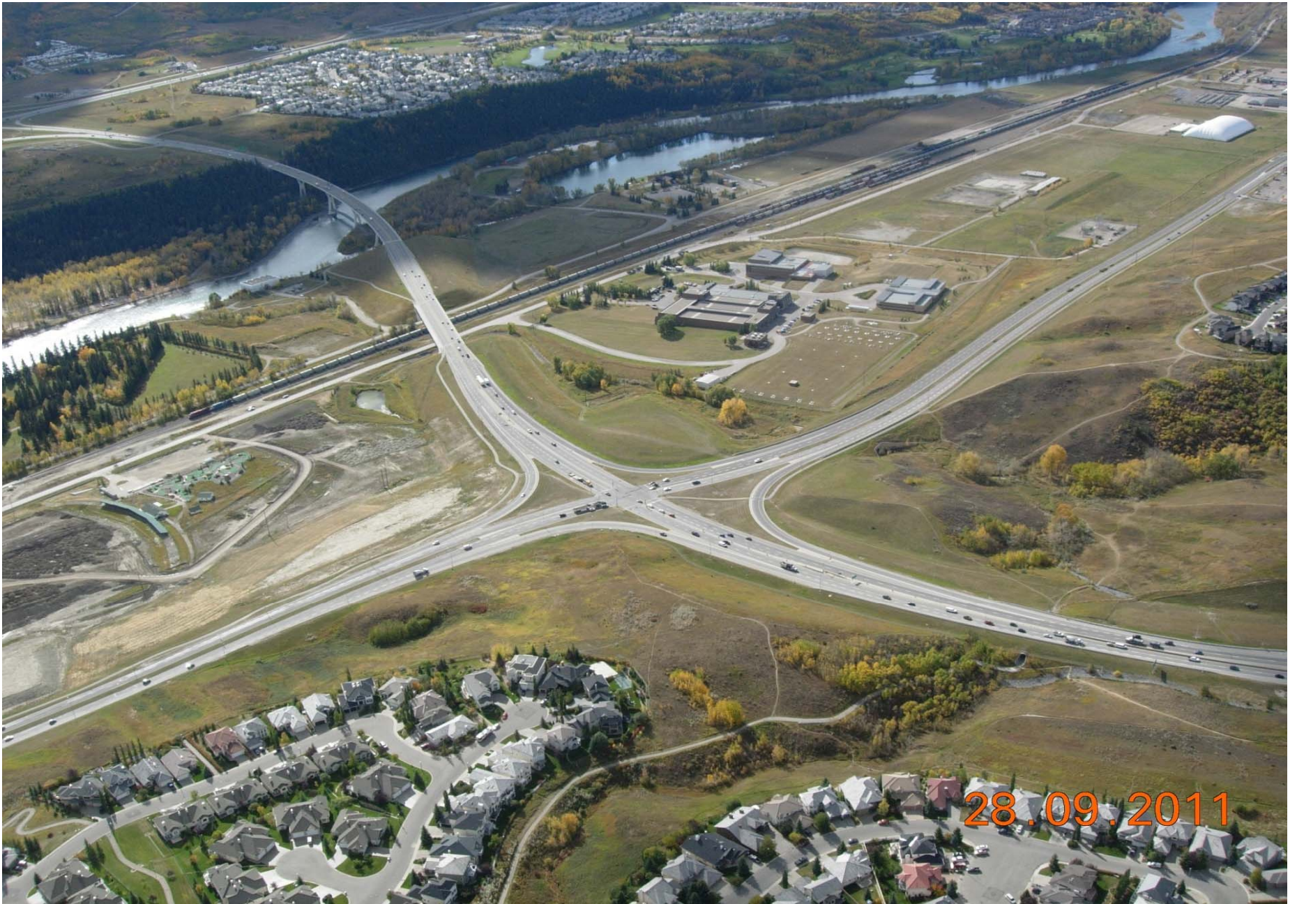
Stoney Trail / Nose Hill Drive Interchange Looking Southwest September 2011
