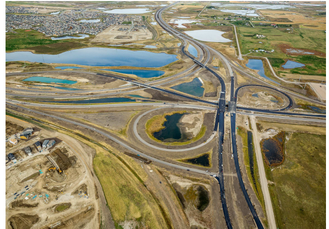
The connection at Stoney Trail and Highway 22X means motorists can go north or south along Calgary's east side.
