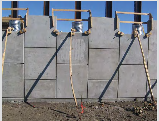
25.12 Adjustment of wall batter using turnbuckles.
