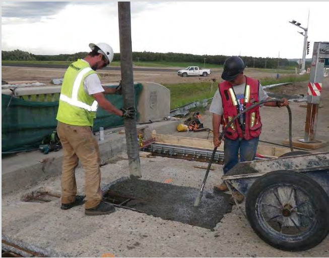
20.9 Concrete being placed into repair area.
