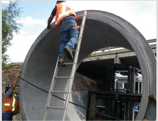
26.6 Gasket placed at spigot end of pipe.
