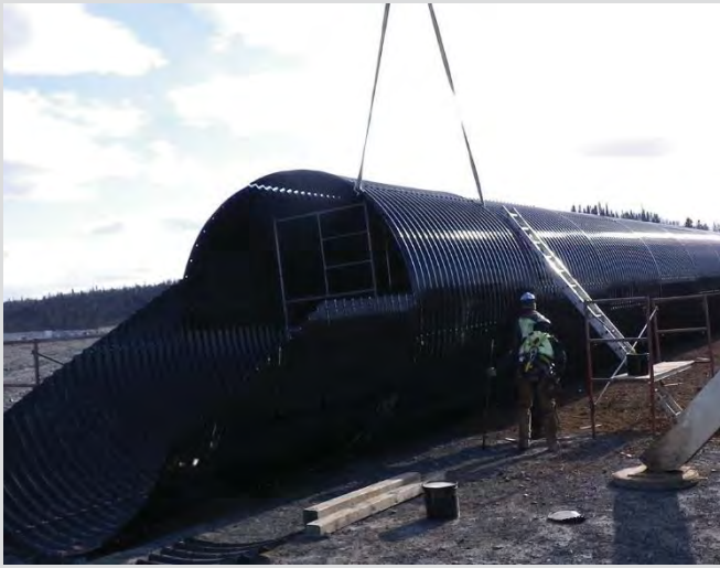
18.5 Assembling SPCSP culvert.
