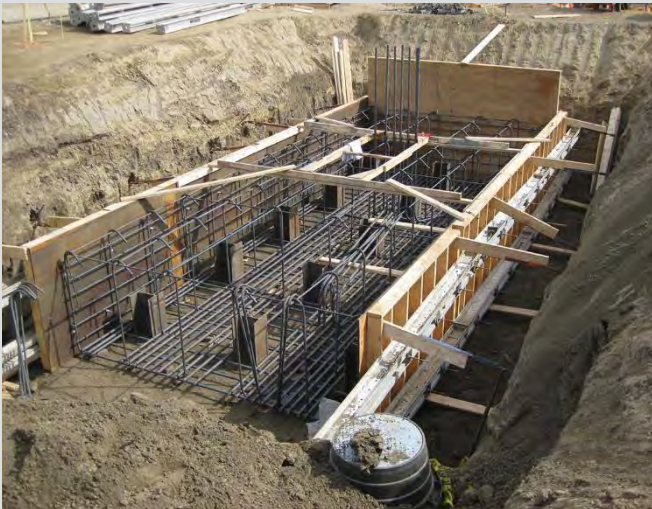
5.3 Pier pile cap formwork and plain reinforcing steel.
