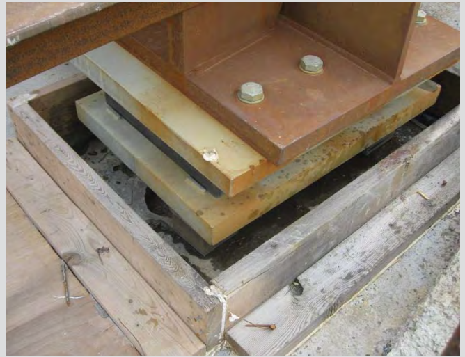
8.6 Block out for grout pad formed and ready for grout.
