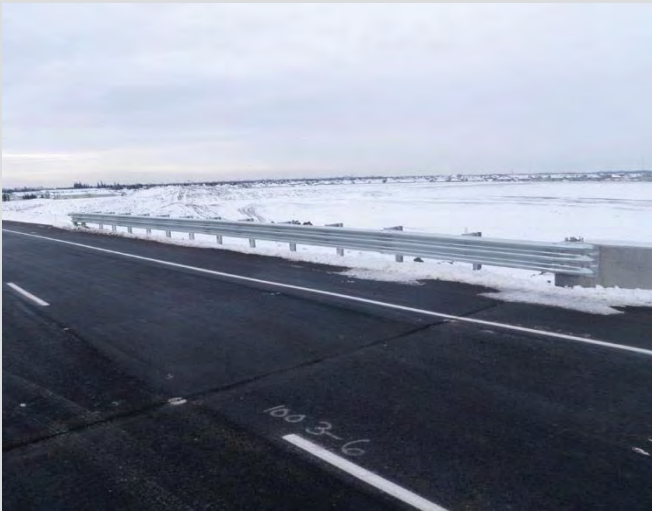
14.7 Guardrail and posts with end treatment.
