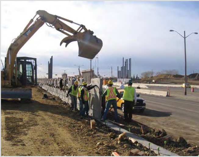
25.5 Installation of first course of panels.
