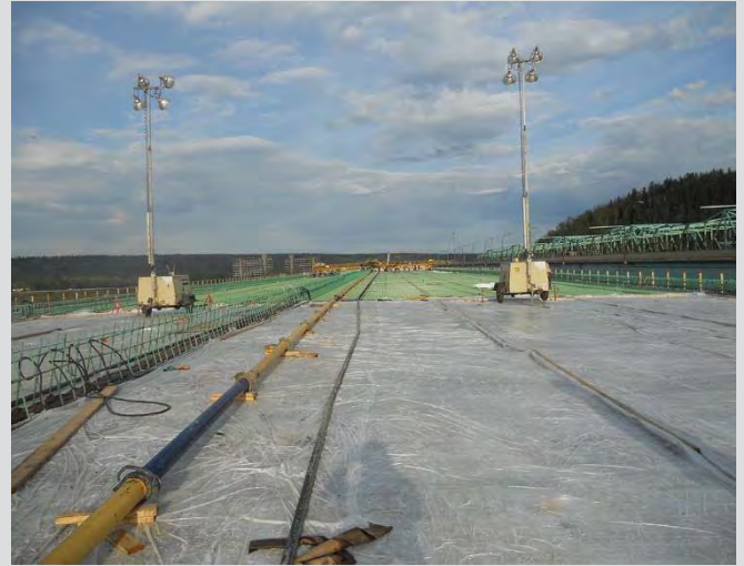
4.64 Line pump used to place deck concrete.
