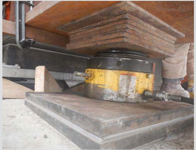
6.27 Pancake jack for final adjustment of bearing for temperature and elevation.
