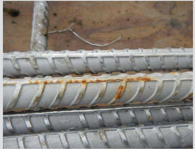
5.14 CRR showing iron contamination. Contamination is caused during fabrication but corrosion may begin at the project site.
