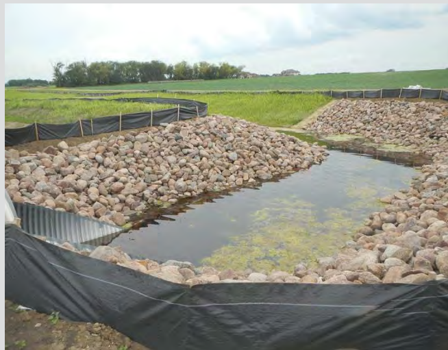
18.24 Completed culvert outlet.
