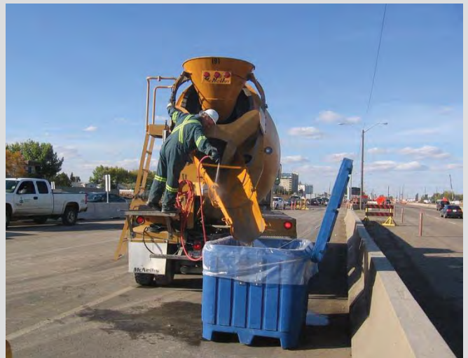
4.104 Concrete washout bin.
