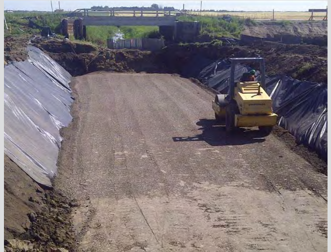
18.16 Backfilling of culvert bed.
