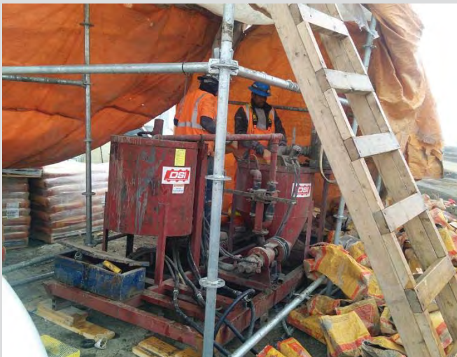
7.30 Portable grout mixer.
