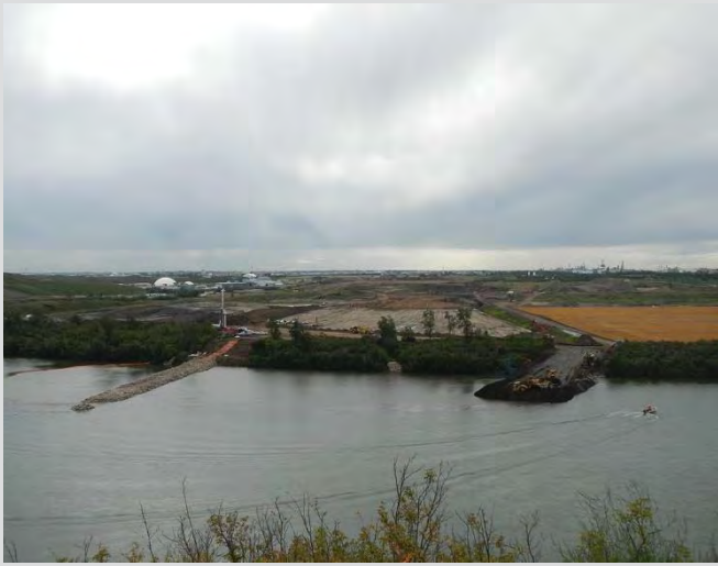
1.5 Installation of berm. Silt curtain downstream to control turbidity.
