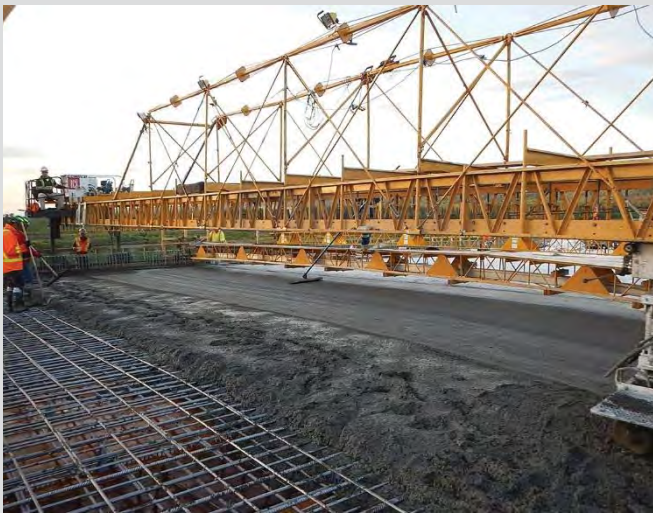
4.57 Deck concrete must be floated as soon as practical after screeding.
