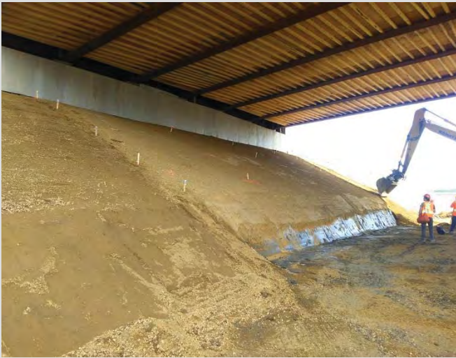
4.109 Excavation for toe cut-off wall
