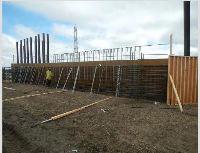
5.2 Abutment seat formwork and plain reinforcing steel.
