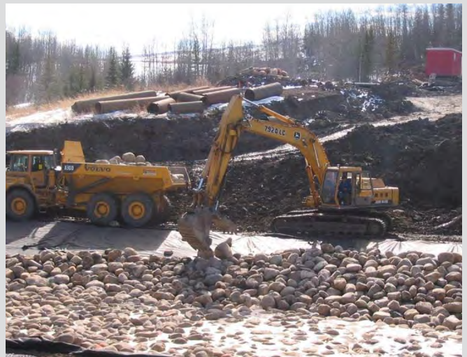
10.8 Riprap placement in creek bed by excavator with a bucket thumb.
