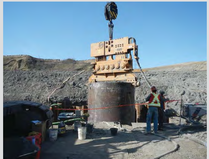
3.43 Vibratory hammer used to remove temporary drilling casing.
