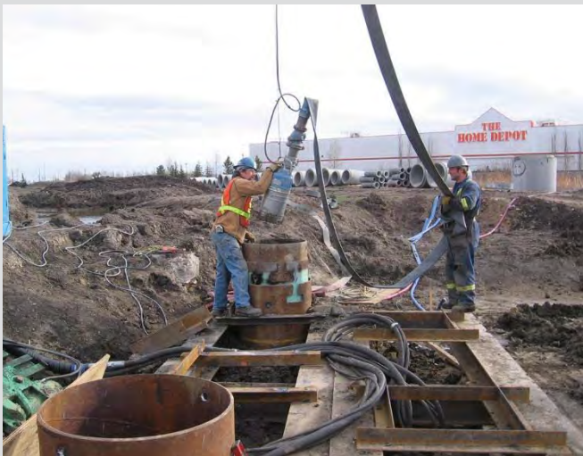
3.30 Water pump may be required to maintain a dry hole.
