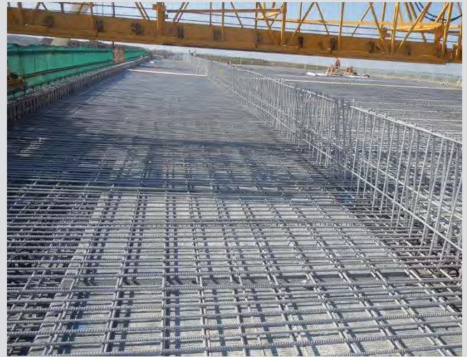
5.10 Deck and barrier CRR placed on precast concrete deck panels.
