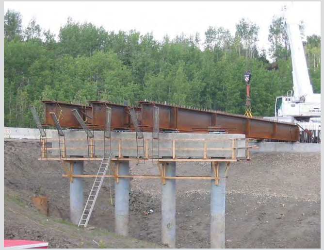
3.45 Galvanized pipe piles at exposed pier columns.
