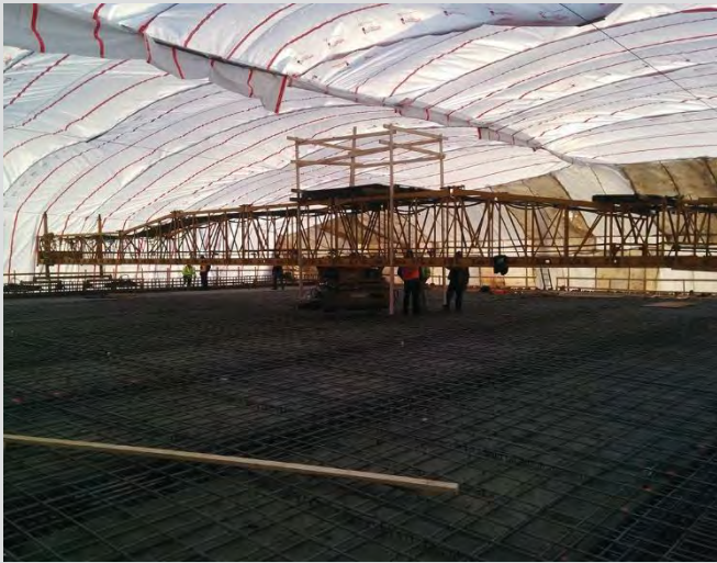
4.59 Full enclosure type heating and hoarding for cold weather deck pour.
