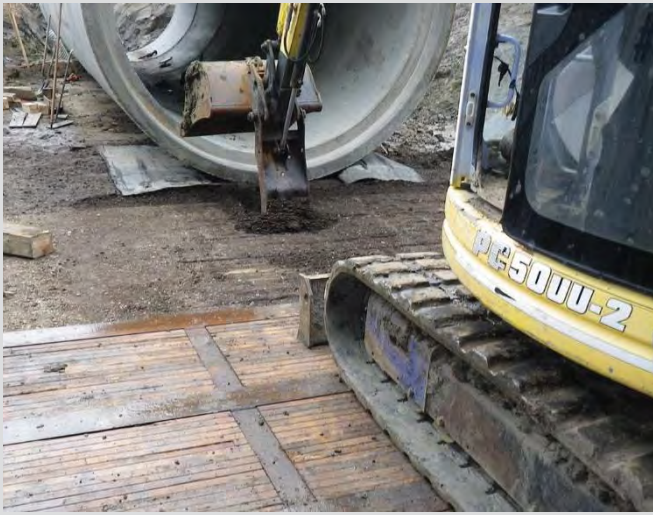
26.9 Loader loosening bedding material at bell.
