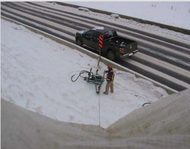
7.26 Winch used to pull strands through post tensioning ducts.
