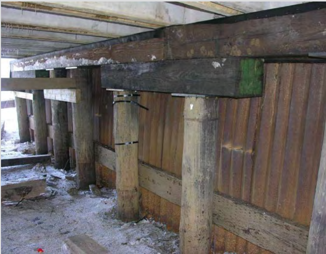
23.7 Treated timber pier cap with splice bearing on treated timber subcap.
