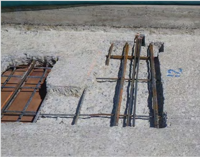
20.5 Full and partial depth repair areas prepared.
