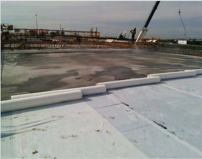
4.67 Crews applying pre-soaked curing fabric.
