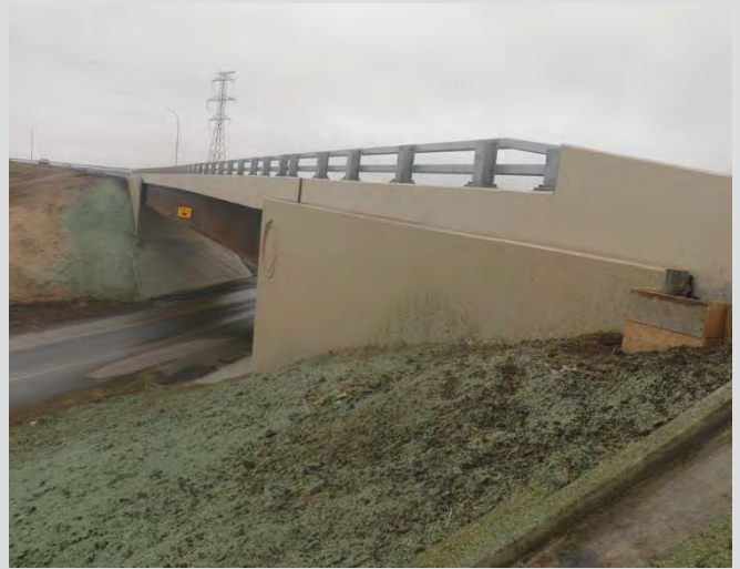
12.9 Completed PL-2 bridgerail.
