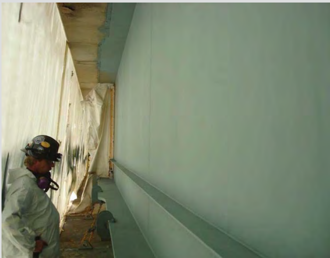
22.7 Primer applied to girder.
