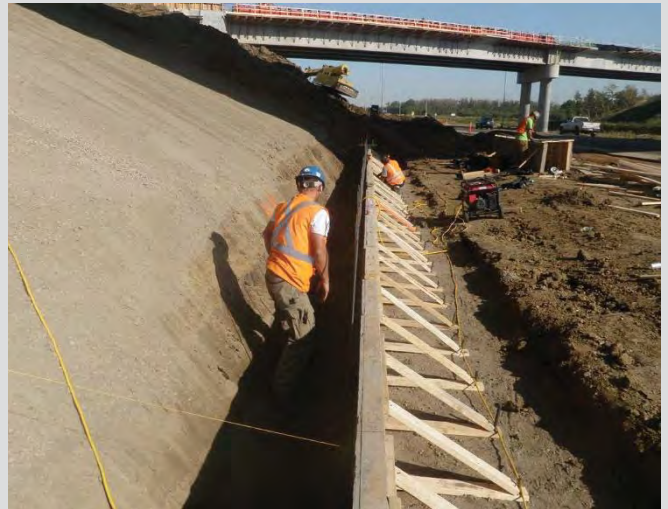
4.108 Toe cut-off wall formwork at base of concrete slope protection.
