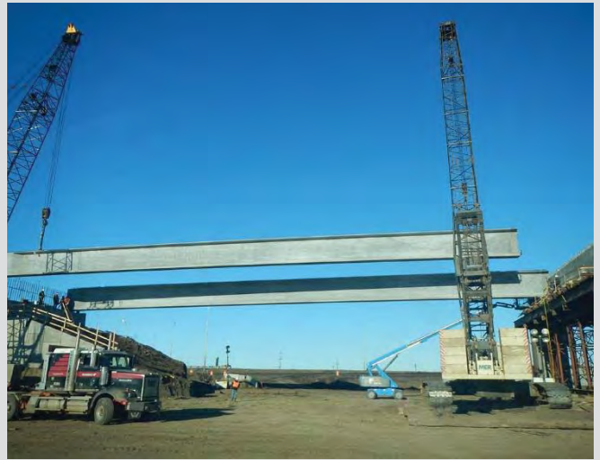
7.2 Lifting precast concrete girder into position with two cranes.
