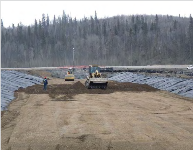
18.27 Backfilling at culvert bed.
