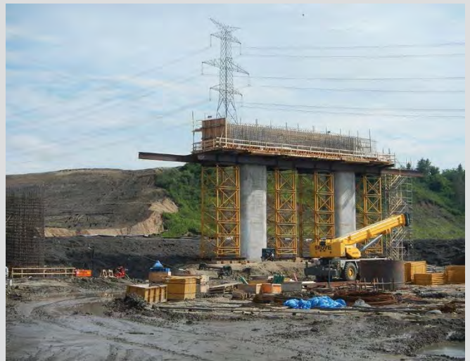
4.15 Pier cap shoring towers and scaffolding.
