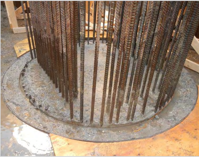
3.44 Construction joint at pile top.
