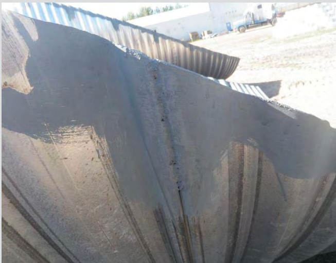
18.11 CSP bevel ends cut by fabricator. Coating repaired using zinc-rich paint
