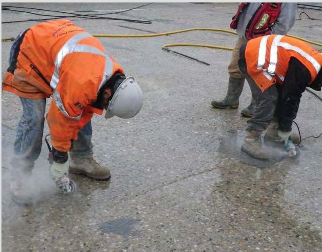
20.11 Workers routing cracks in preparation for epoxy.
