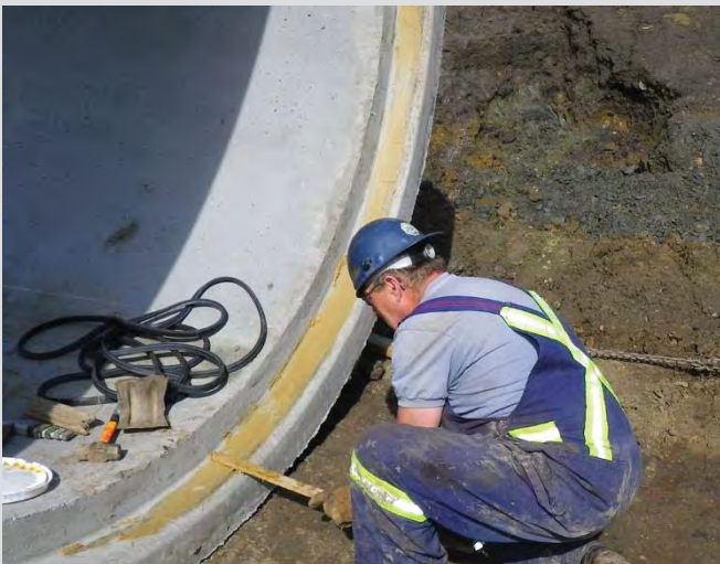
26.7 Placing gasket adhesive.
