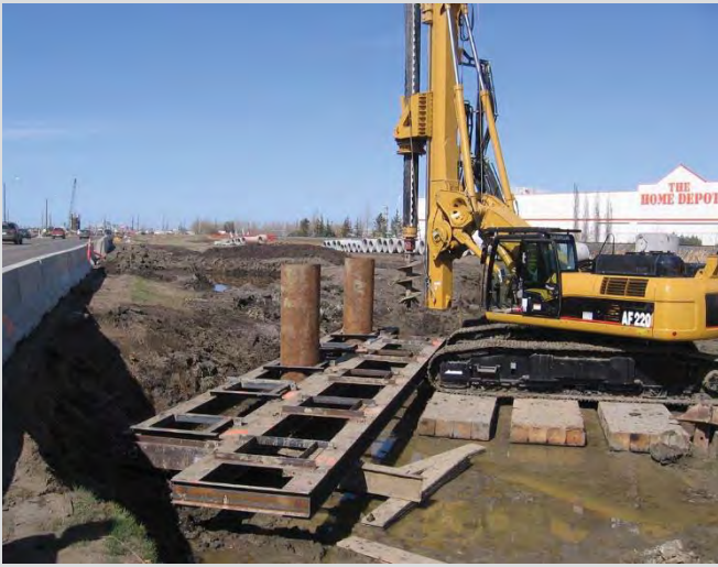
3.20 Drilling frame used to achieve pile location accuracy.
