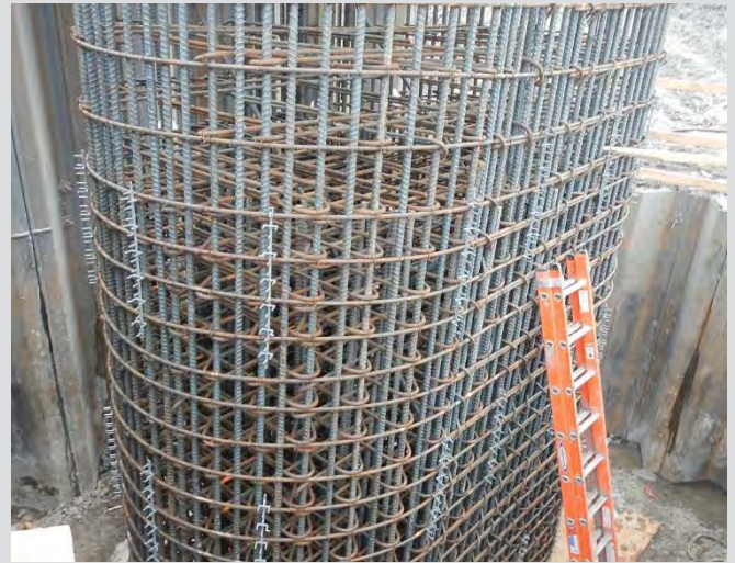
5.6 Pier column plain reinforcing steel.
