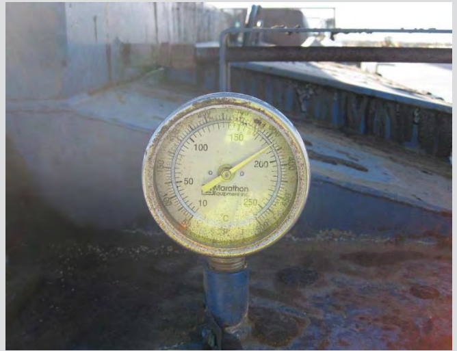
16.6 Asphalt membrane heating in kettle.
