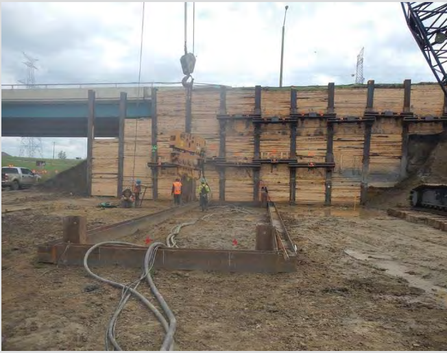
1.12 Steel H-beam frame set at perimeter of excavation.
