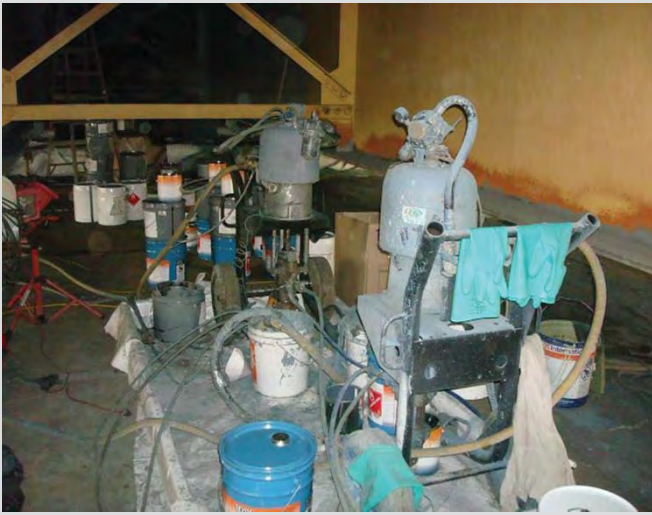
22.9 Typical paint setup.
