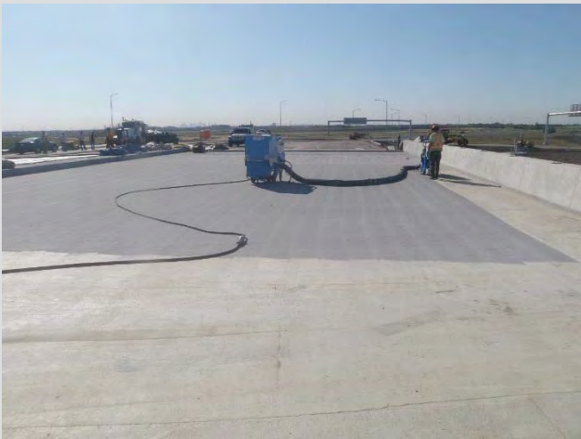
16.3 Surface preparation by shot-blasting.
