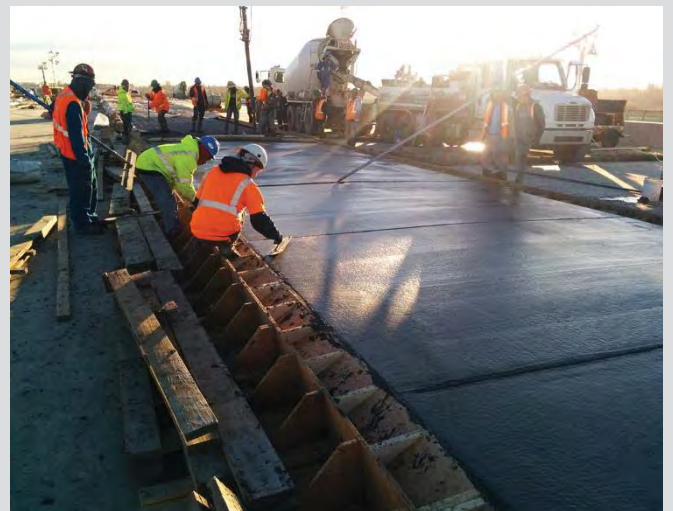
4.87 Crews tooling joints at 3.0 m spacing. Broom finish to be applied.
