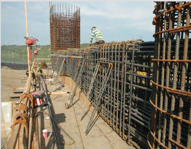
4.14 Pier strut with plain steel reinforcement.
