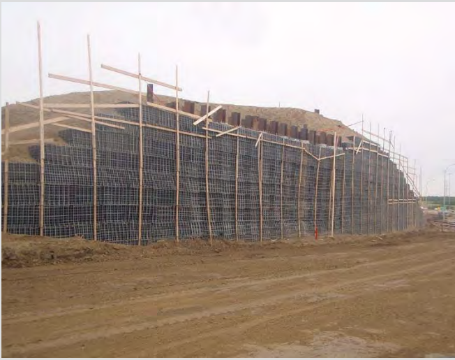
25.27 Wire wall completed at two stage wall.
