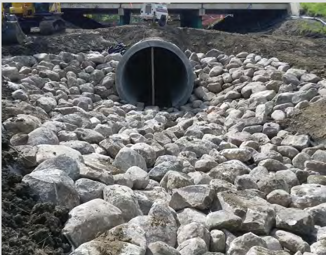
10.7 Riprap apron placed at RCP end.
