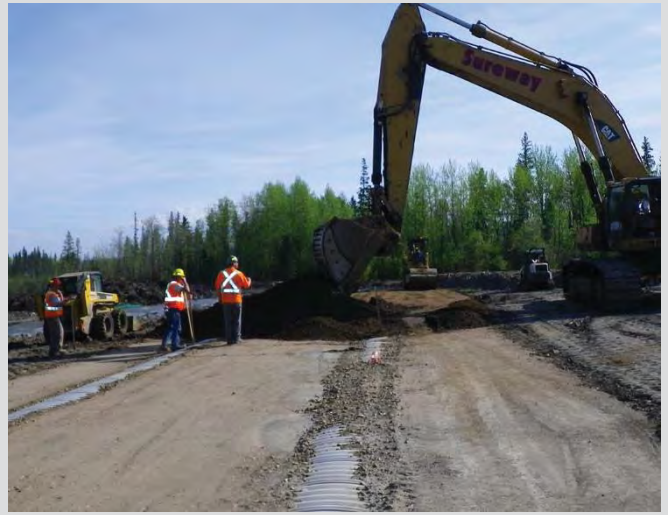
18.34 Completing backfill placement at crown of culverts.
