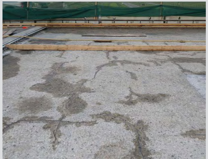
20.12 Cracks prepared for epoxy repair.
