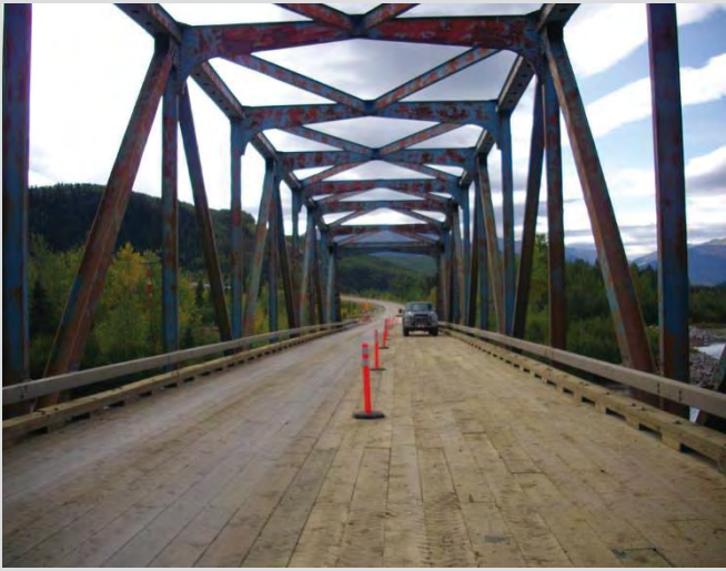
23.5 Completed strip deck.
