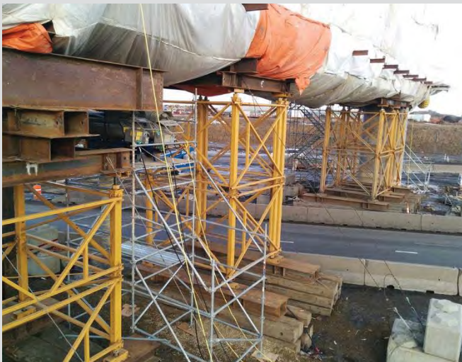
4.25 Scaffolding and shoring towers for straddlebent pier beam.
