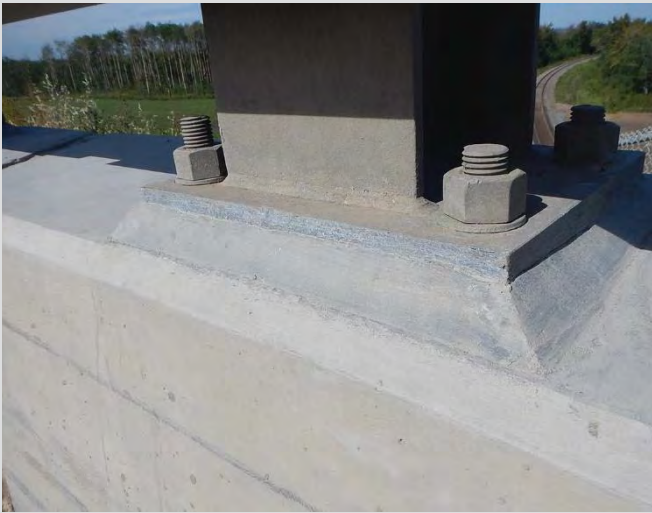
12.4 Completed bridgerail grout pad. Acceptable projection of bolts shown.
