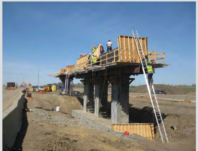
4.4 Pier cap formwork being erected.
