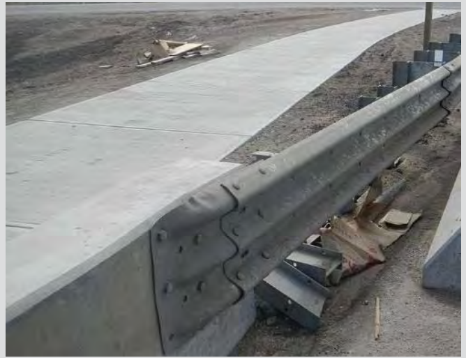
14.2 Guardrail to bridgerail transition.
