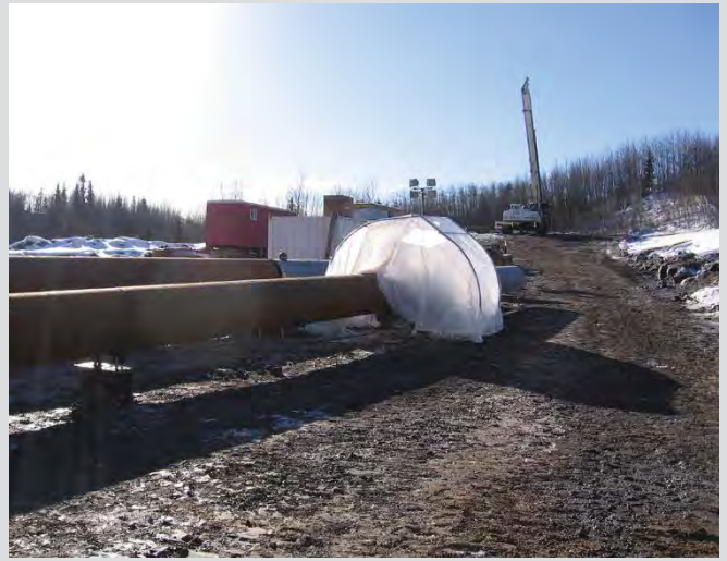
13.6 Hoarding setup for welding in windy or cold conditions.
