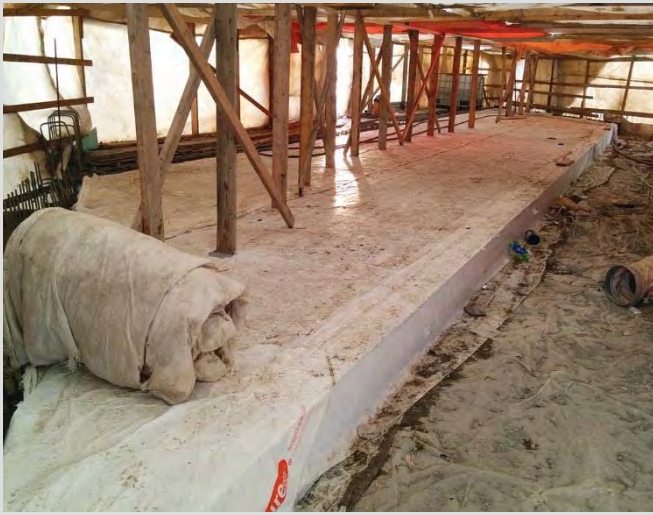
4.75 Heating and hoarding during winter curing.
