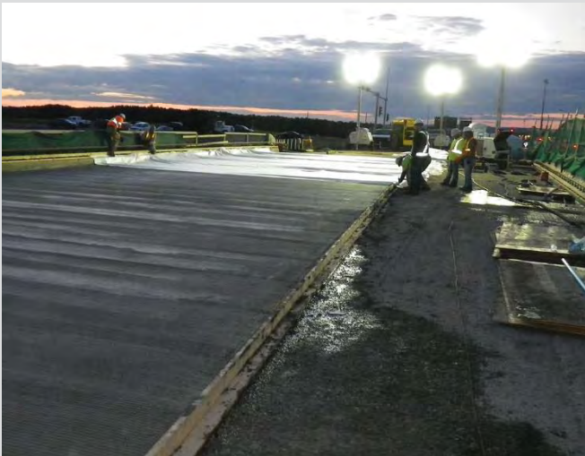
20.19 Overlay concrete placed and curing fabric being installed.
