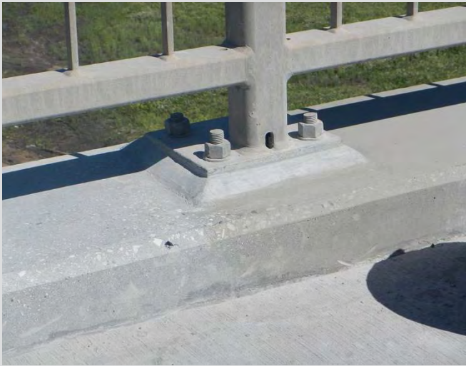
12.8 Completed pedestrian rail grout pad.
