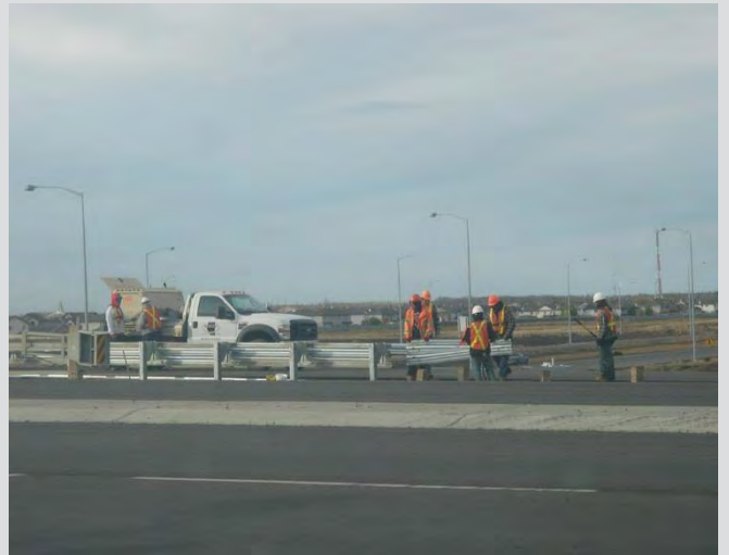
14.8 Installing guardrail to posts.
