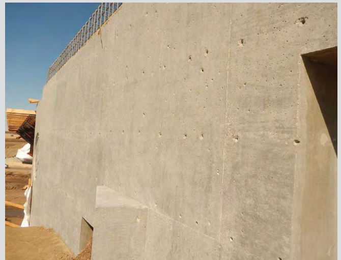
4.91 Wing wall after form stripping. Form tie holes to be patched.
