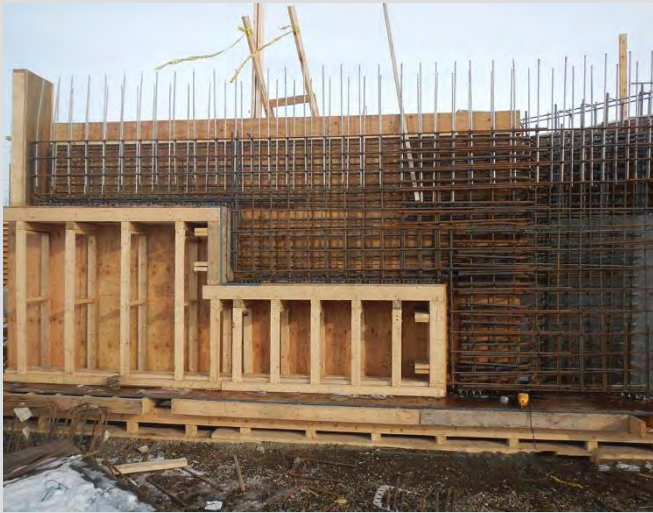
5.5 Wingwall reinforcing steel. CRR projecting for barriers.
