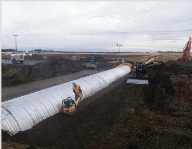
18.23 Compaction of granular backfill material.
