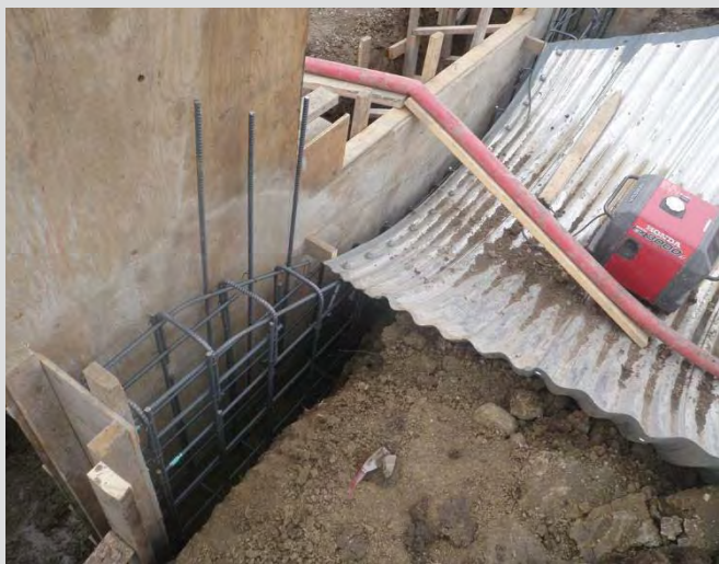
18.21 Formwork and reinforcing steel for cast-in-place cut-off wall.
