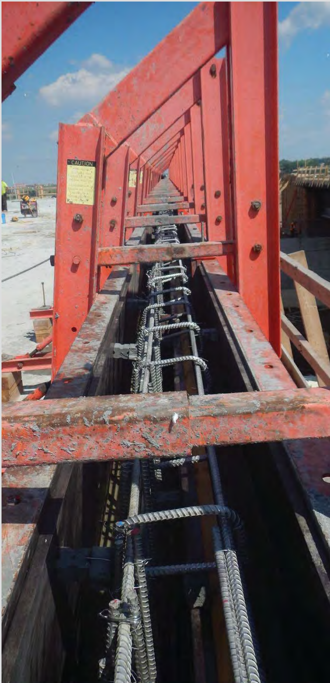
4.86 Re-usable steel forms for barriers.
