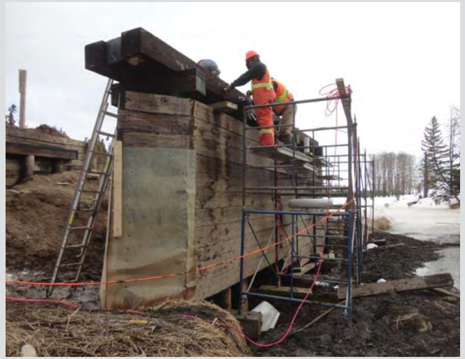
23.6 Treated timber pier cap replacement.
