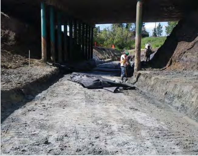
26.1 Excavation for bedding complete. Placing filter fabric prior to bedding material.
