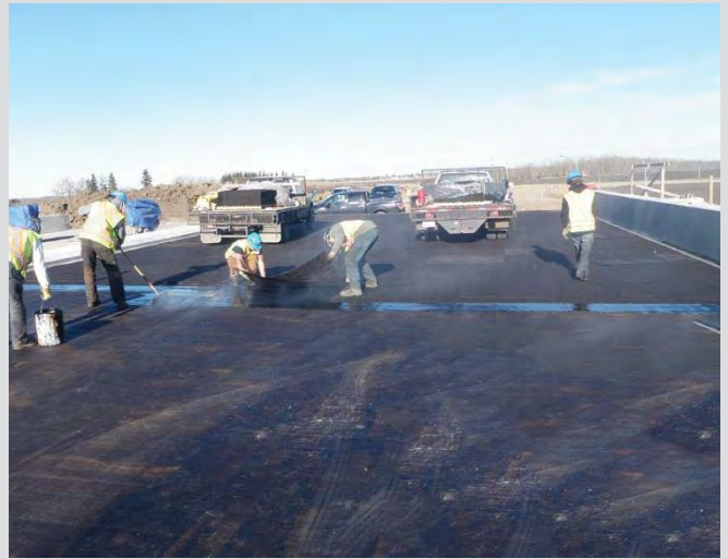
16.10 Protection board placed immediately after asphalt membrane has been placed.
