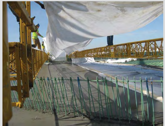
4.66 Placement of curing fabric from work bridges.
