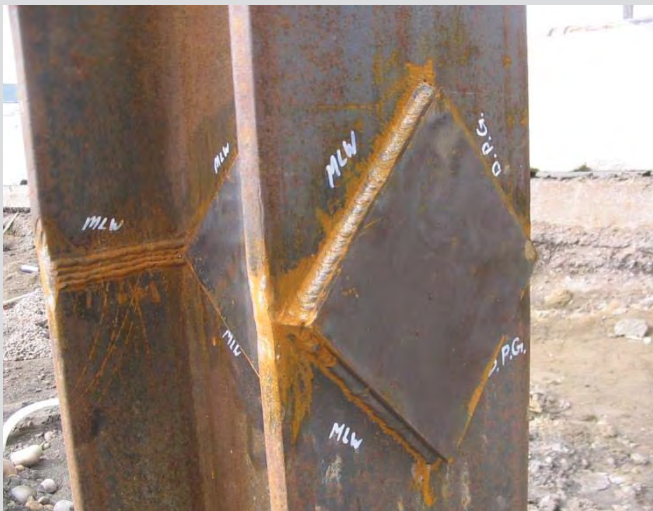
13.3 Completed H-pile splice plate detail.
