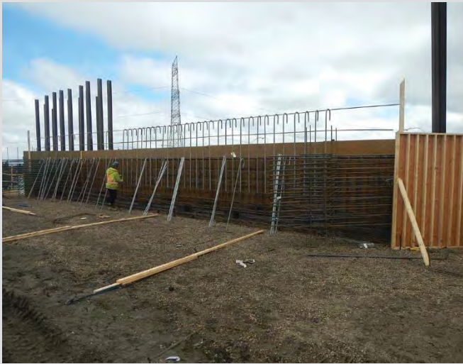
4.1 Abutment seat partial formwork and reinforcing steel.
