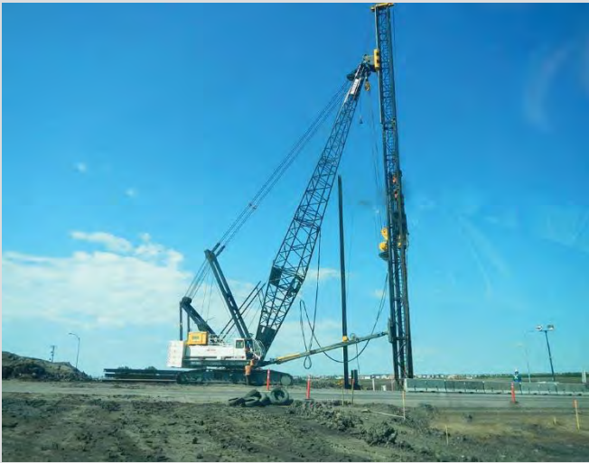
3.1 Diesel hammer and crane showing “fixed” box leads.
