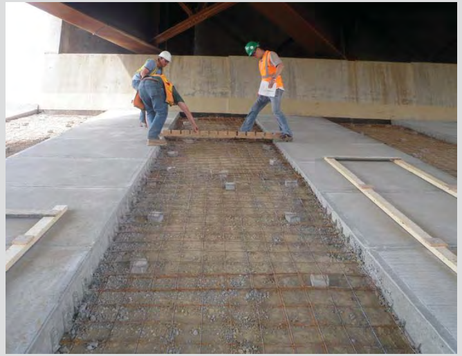
4.114 Checking cover and alignment.
