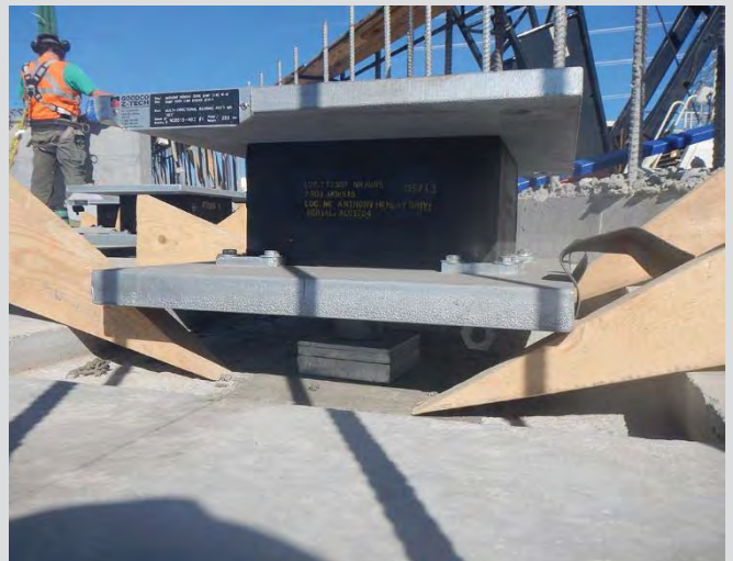
7.8 Setting elastomeric bearing with wooden wedges.
