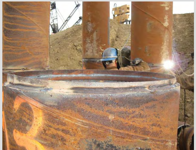
13.4 Splicing pipe pile. Bevelled edge with backup ring.
