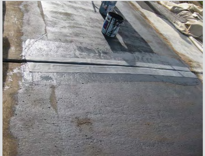
16.8 Membrane reinforcing fabric placed along construction joint.
