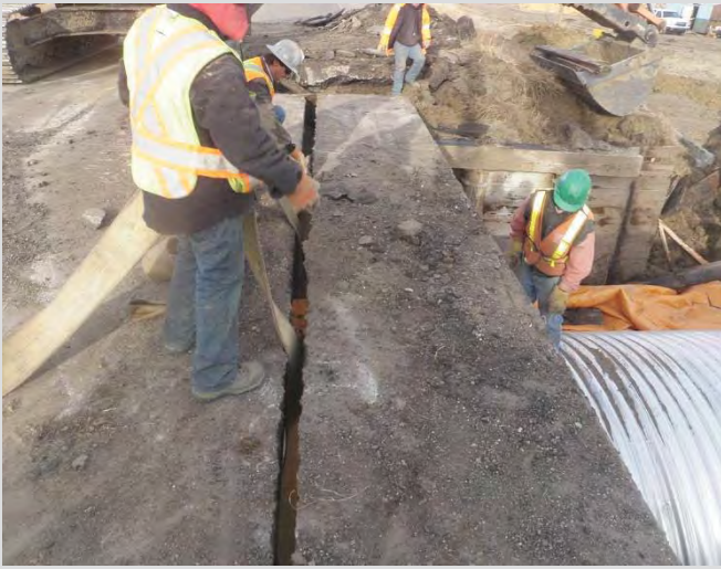
21.1 Concrete box girders salvaged. Girders lifted at their bearing points.
