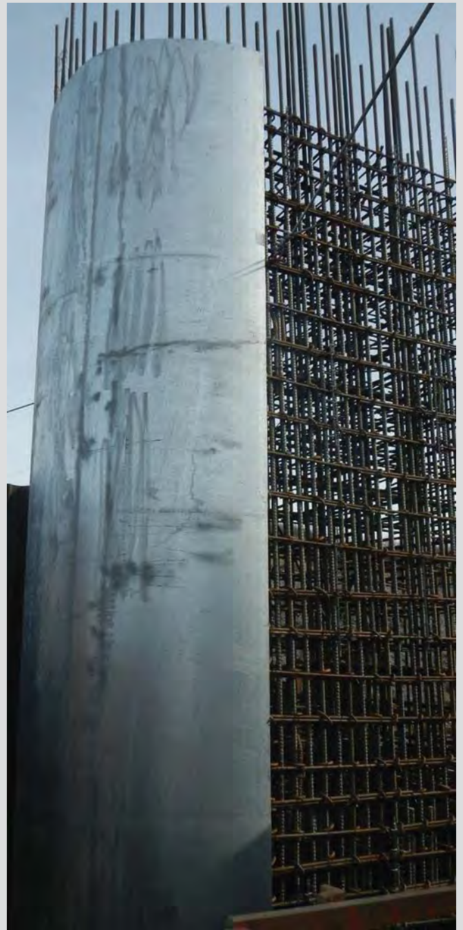
6.21 Galvanized nose plate for river pier protection.
