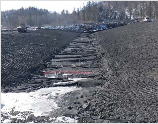
18.1 Culvert bed excavation completed and filter fabric placed.
