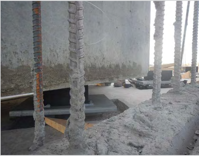
7.9 Concrete box girder on bearing.
