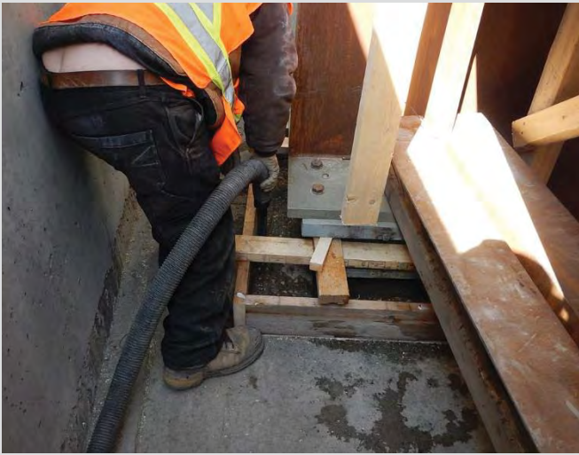
8.9 Clean-out prior to grouting.
