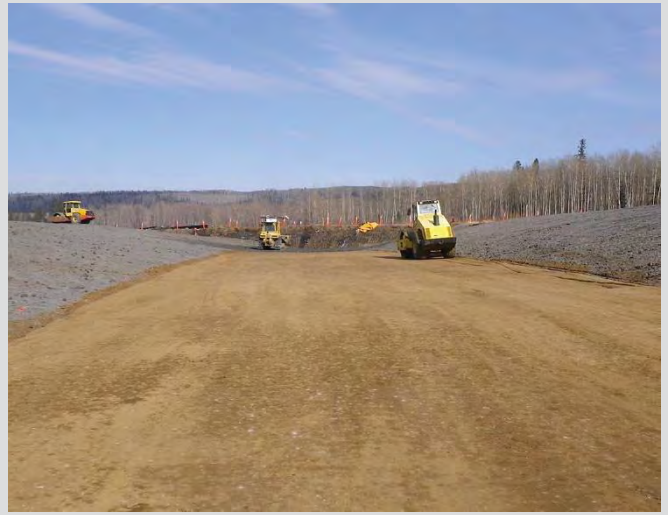
18.2 Compacting of culvert bedding material.
