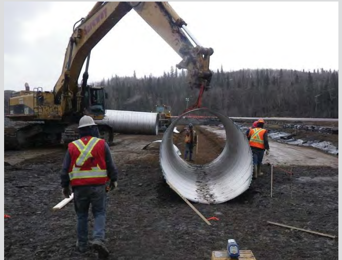
18.28 Installation of CSP structure at pre-shaped bed.
