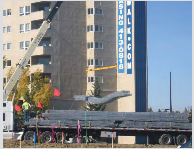
25.24 Correct handling using spreader bar.
