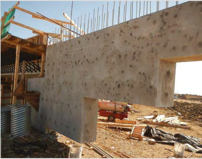
4.92 Outside face of wingwall showing patching of form tie holes.
