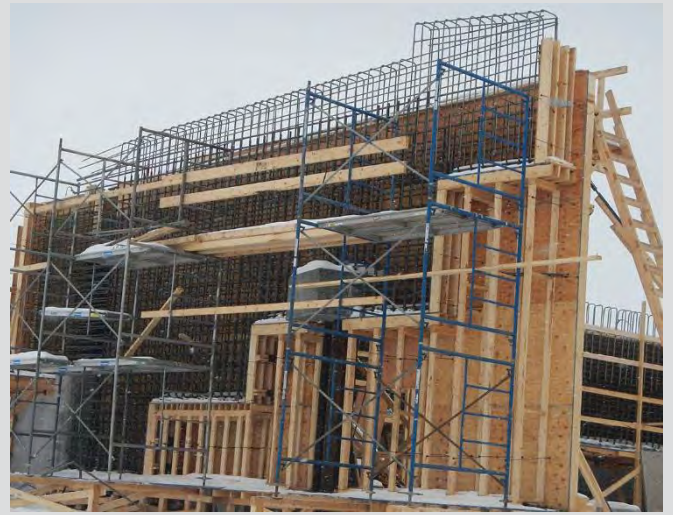
4.5 Partial wingwall formwork.
