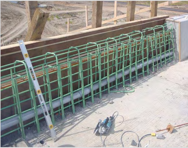
11.1 Duct for electrical conduit in barrier.
