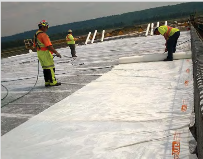
4.69 Placement of second layer of filter fabric after initial set.
