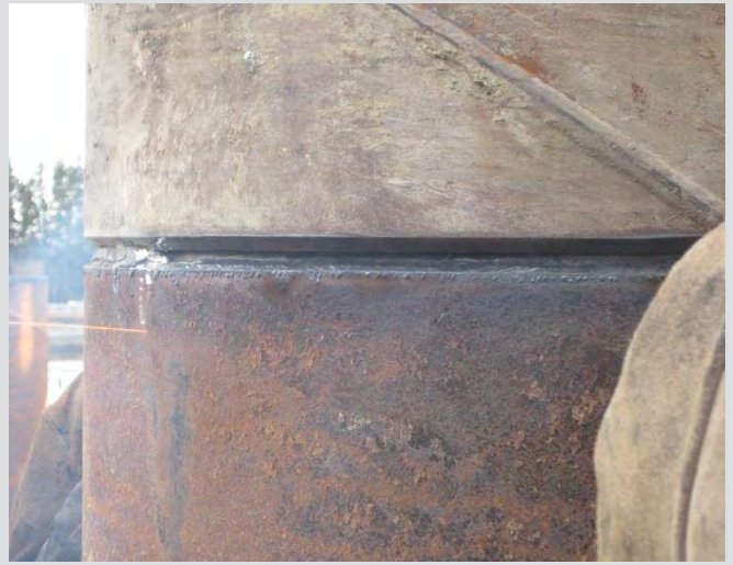
3.25 Splicing pipe pile shown after fit-up.
