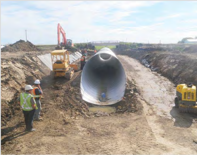
18.17 Backfill being placed at haunches.
