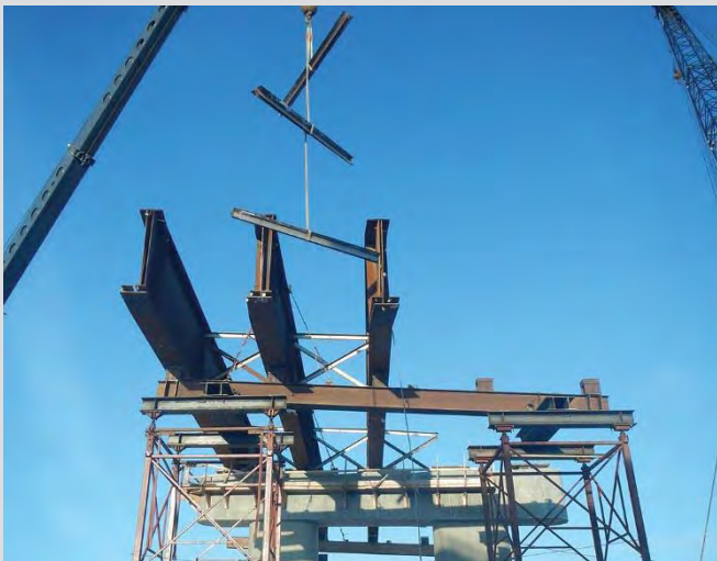
6.7 Steel diaphragm bracing installation with crane.
