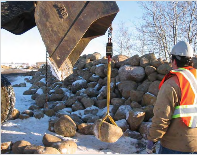
10.1 Load cell used to weigh heavy rock riprap at site.
