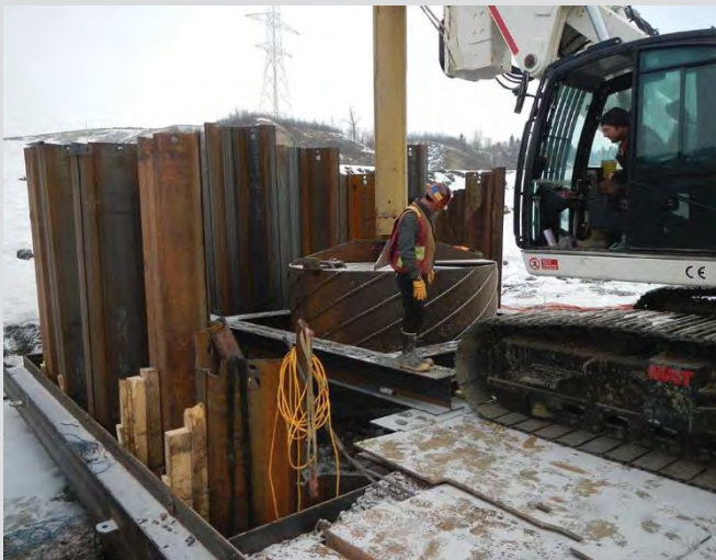
3.38 Large 3.0 m diameter pile. Muck bucket attached.
