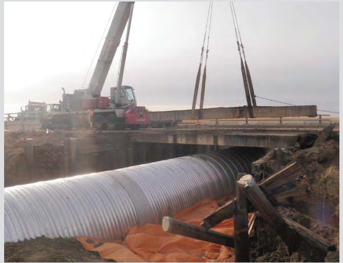
18.18 Removal of existing bridge structure.
