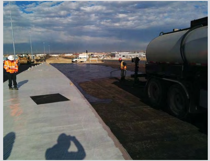
17.2 Application of tack coat by hand sprayer.
