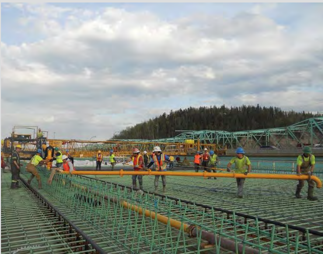
4.65 Line pump with adjustable swivel arm for accurate concrete placement.
