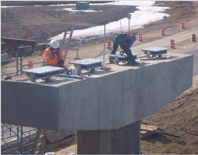
8.1 Placing bearings at pier cap.
