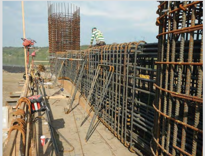
5.4 Pier strut consisting of plain reinforcing steel.
