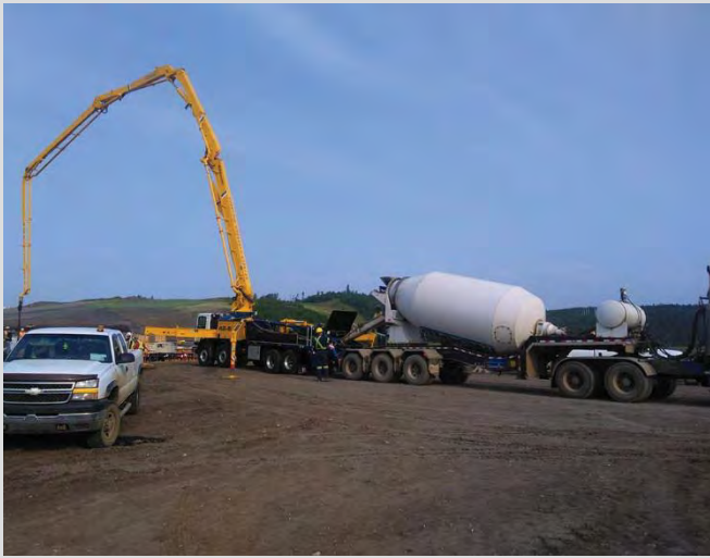
4.105 Typical trailer-type concrete mixer and concrete pump.
