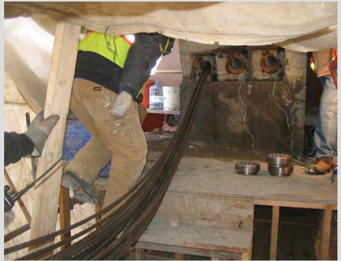
7.25 Tendons pulled through post-tensioning ducts.
