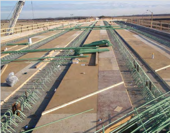
4.45 Deck formwork in place on concrete girders.
