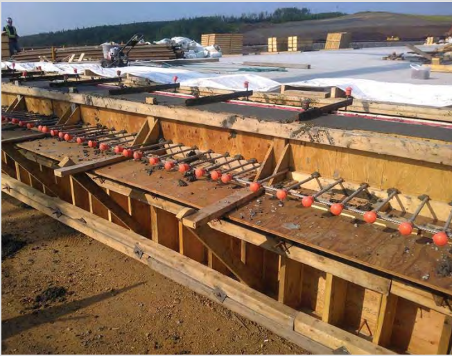
4.31 Backwall corbel formwork.
