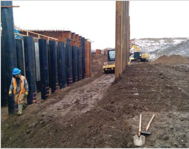
2.1 Compaction of backfill between abutment pipe piles and grade beam H-piling.
