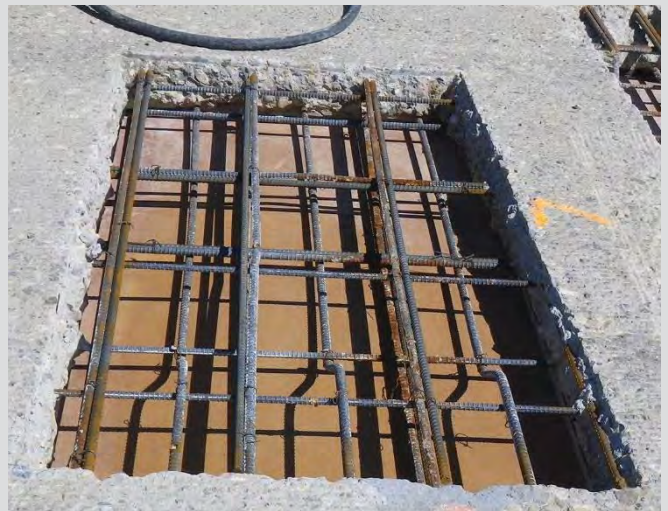
20.4 Full depth repair area prepared.
