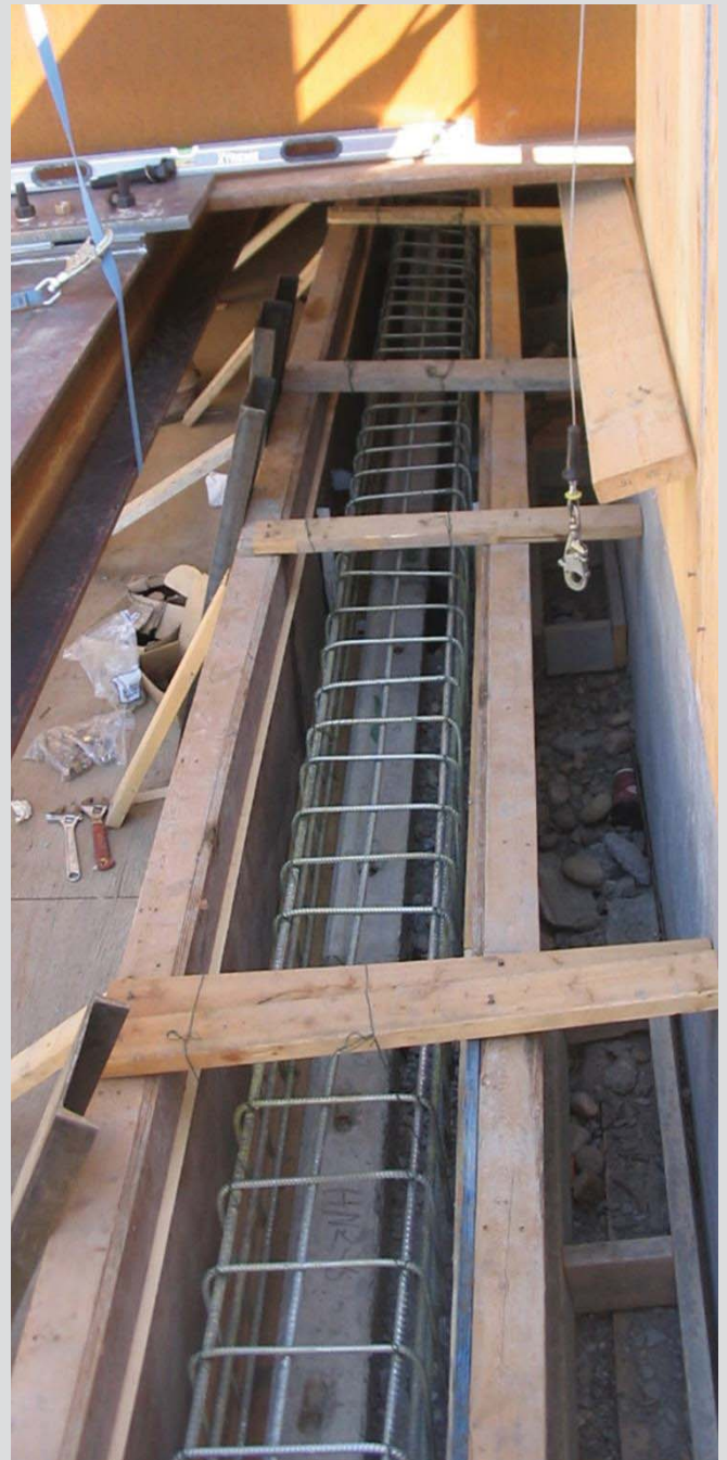
25.18 Cast-in-place coping cap.
