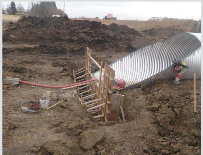
18.20 Formwork for cast-in-place collar cut-off wall.
