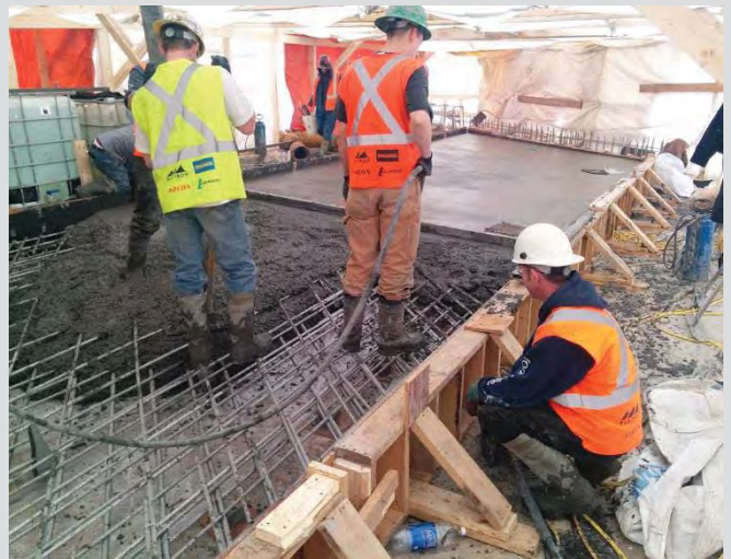
4.74 Placing approach slab concrete.
