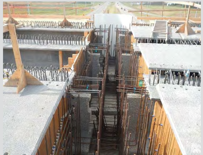
4.11 Pier diaphragm formwork and reinforcing steel.
