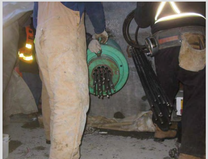
7.27 Jack used for post-tensioning. Tendon strand protruding beyond jack end.
