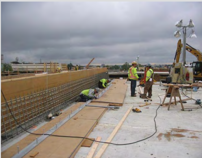
5.11 Crews tying barrier CRR.
