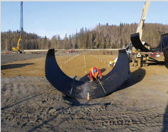
18.3 Assembling SPCSP culvert. Plates lifted into position with crane.
