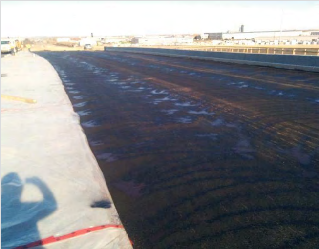
17.3 Application of tack coat by spray truck.
