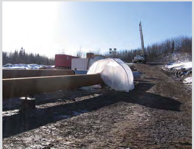
3.27 Hoarding for welding required during cold and windy conditions.
