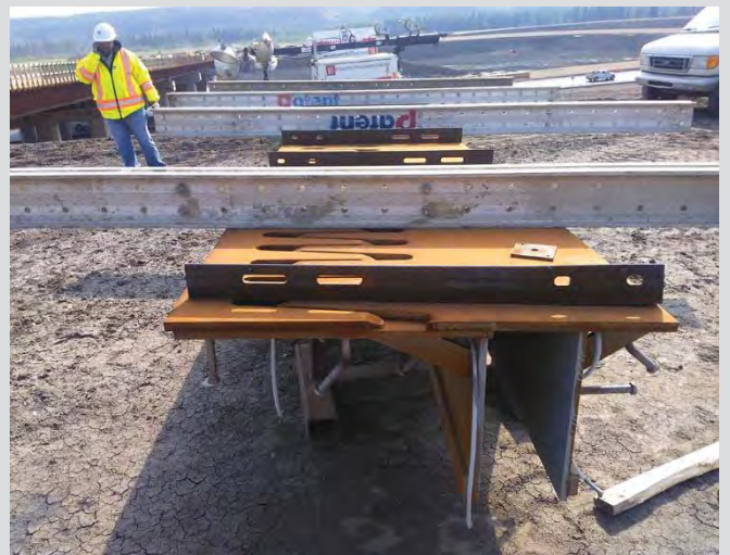
6.19 Finger type joint showing erection angles.
