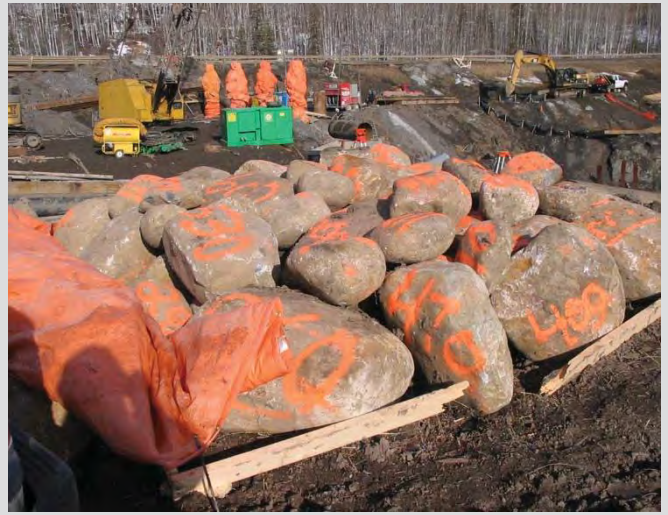
10.2 Heavy rock riprap sample with weights painted on each piece.
