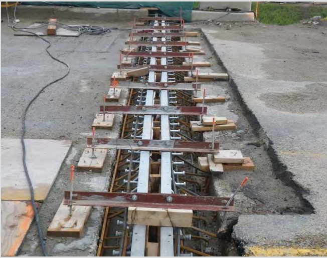
20.17 Type I strip seal deck joint ready for concrete placement.
