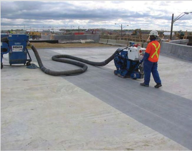
16.1 Deck surface preparation by shot-blasting.
