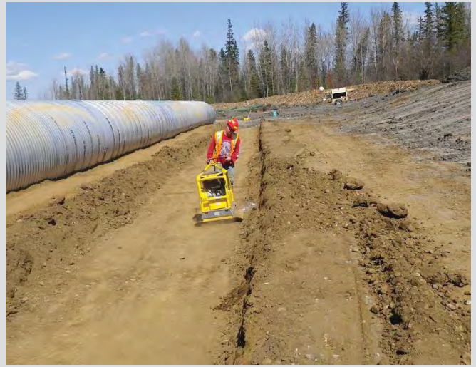
18.30 Pre-shaping and compacting bed material for second CSP structure.
