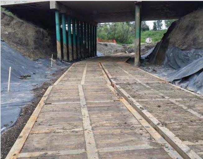
26.3 Rig mats placed to allow for ease of access to work.
