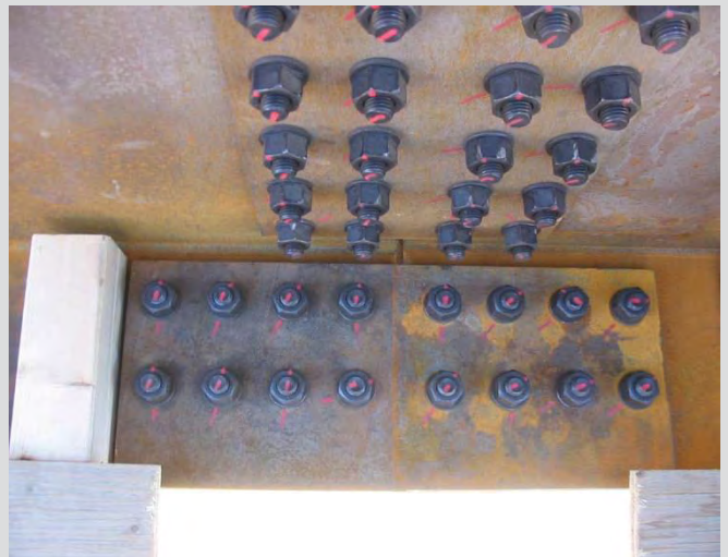
6.8 Splice plate detail. All bolts tightened by turn-of-nut method.
