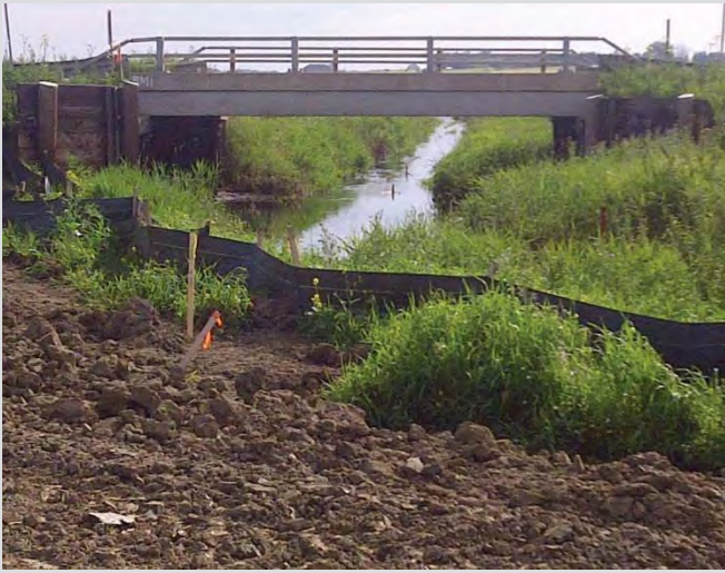
18.13 Temporary watercourse diversion.
