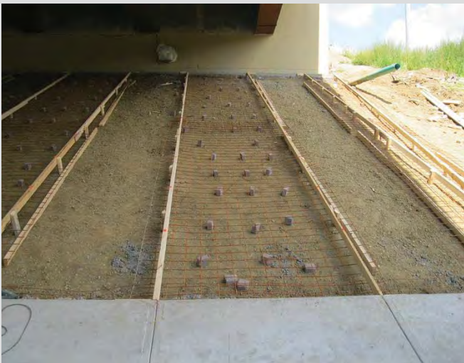
4.111 Forming vertical courses. Reinforcing mesh chaired using masonry bricks.
