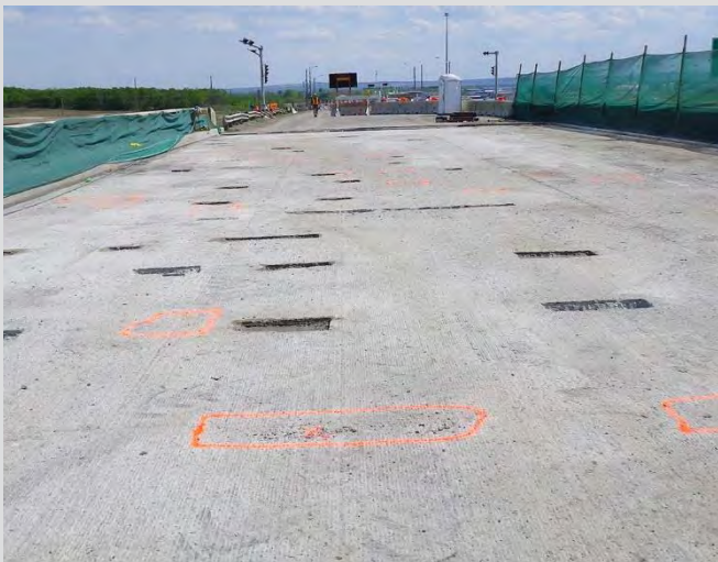
20.3 Partial or full depth repair areas prepared.
