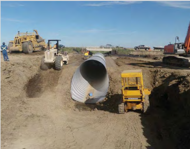
2.11 Placing backfill evenly on both sides of culvert in 150 mm lifts.
