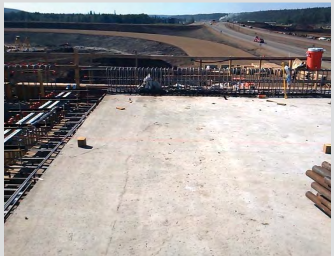
6.16 Strip seal type joint temporarily supported.
