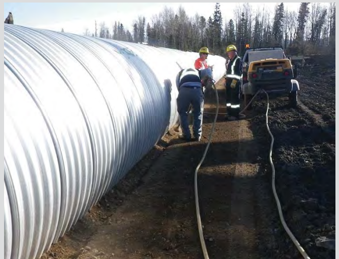
18.32 Backfilling and compacting haunch area.
