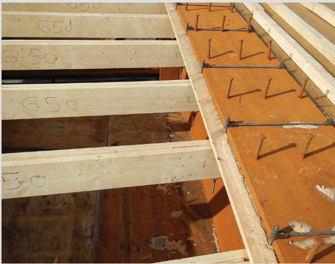
4.35 Timber ledger beams are typically hung from hanger rods.
