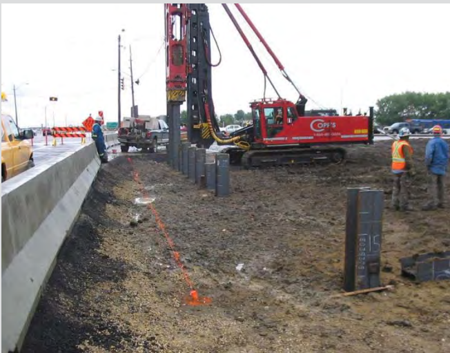
3.3 Hydraulic pile driving hammer. Pile offset line marked with paint.
