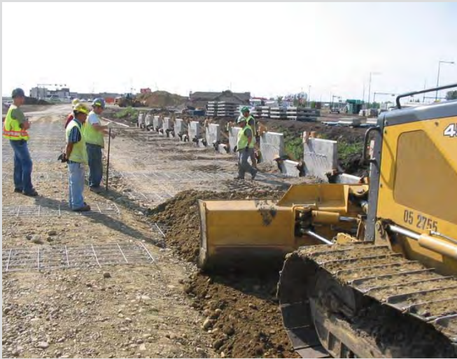
25.9 Hydraulic excavator pushing backfill material over soil reinforcement.
