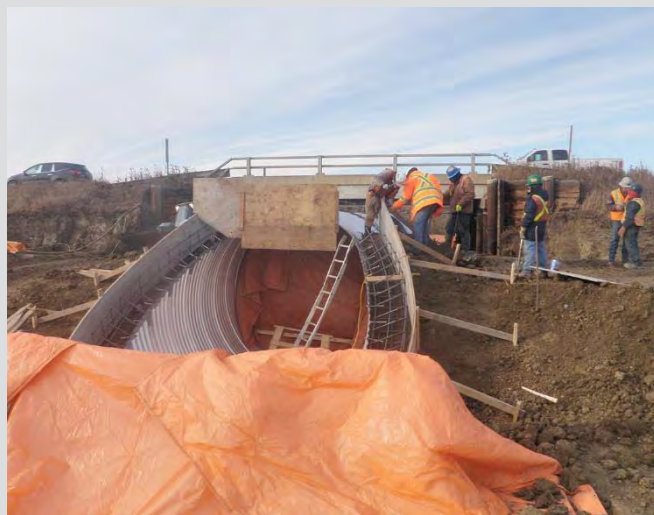
18.22 Concrete placement for collar.
