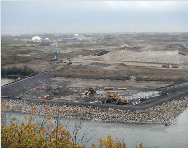
1.9 River berm construction complete. Sides armored with riprap and filter fabric.
