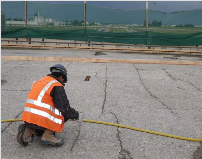
20.13 Cracks being filled with gravity flow epoxy.
