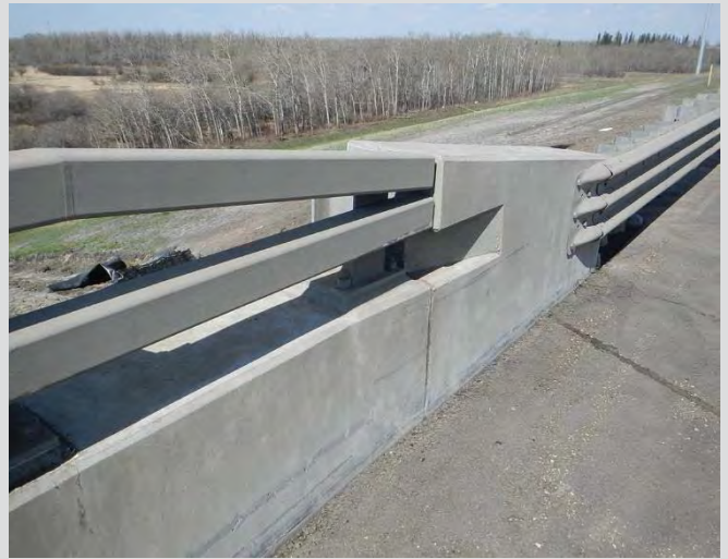
12.5 Bridgerail to guardrail transition.
