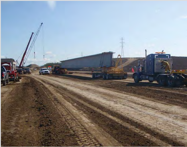
7.1 Precast concrete NU girder delivered to site.
