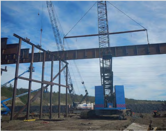
6.5 Erecting girder between piers. Spreader bar used to erect girder.
