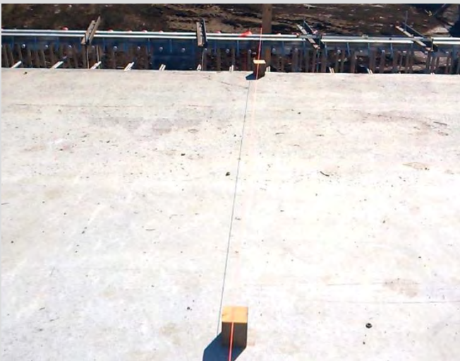
6.15 Checking joint alignment with stringlines and instrument.
