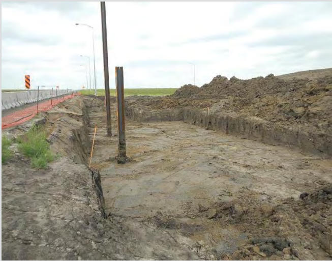
25.1 Ground improvement excavation. Soil was removed since it was not competent.
