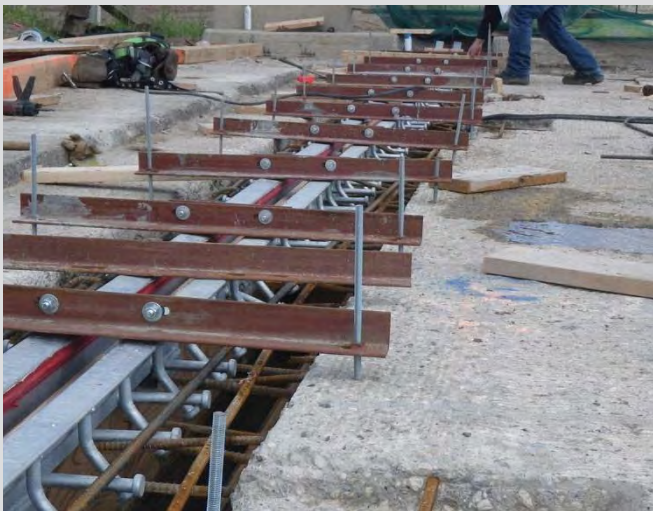
20.15 Deck joint set into position using erection angles.
