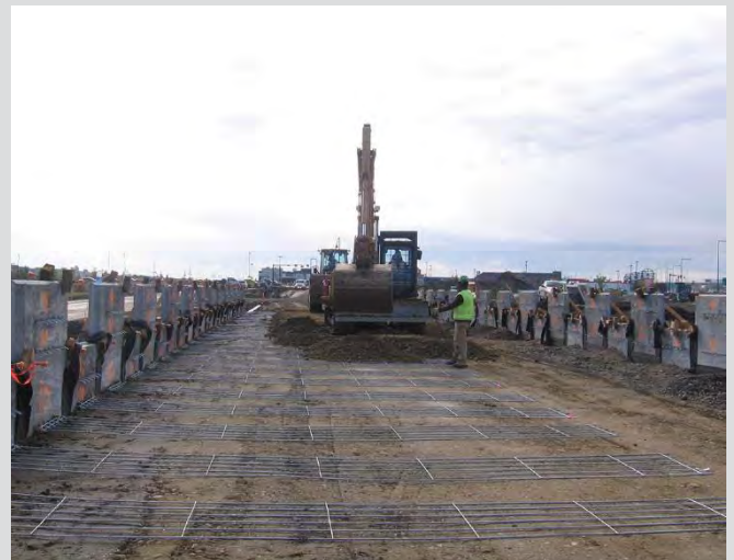
25.8 Hydraulic excavator pushing backfill material over soil reinforcement.
