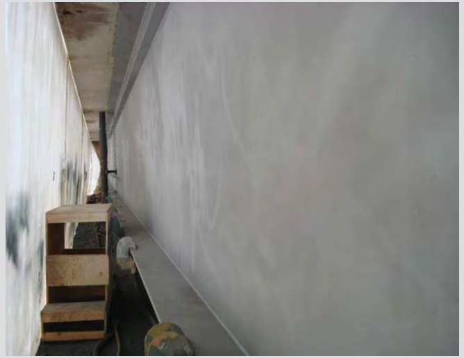
22.6 Girder after sandblasting.
