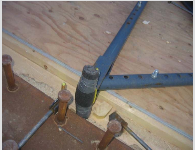
4.44 Softener wrapped around bracket end to prevent girder web damage.
