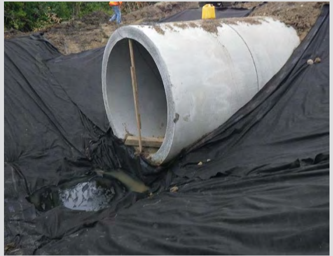
10.6 Filter fabric placed around end of RCP.
