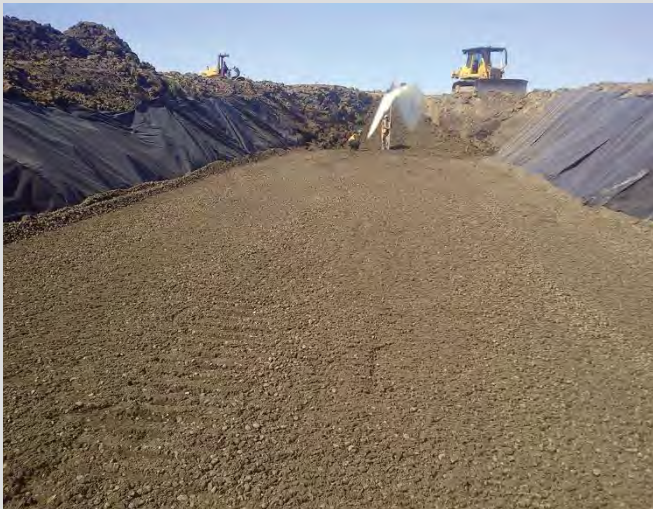
2.7 Culvert foundation material in loose state, spread by dozer.
