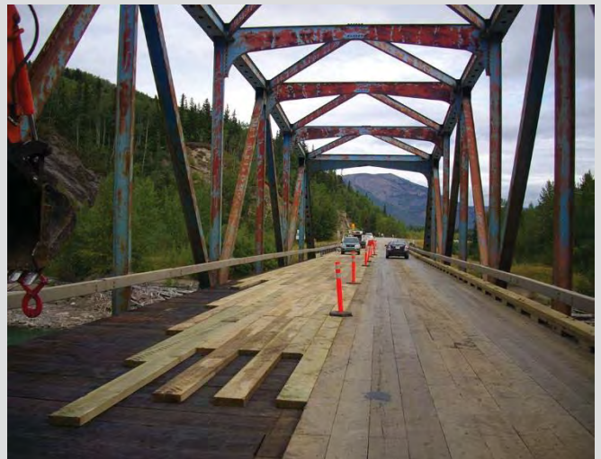
23.4 Strip deck replacement ongoing, boards staggered.
