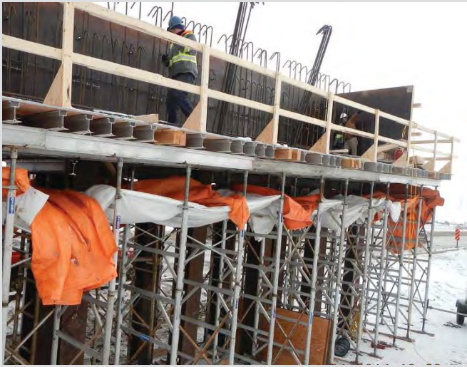
4.12 Elevated construction. Shoring towers used to construct abutment seat.
