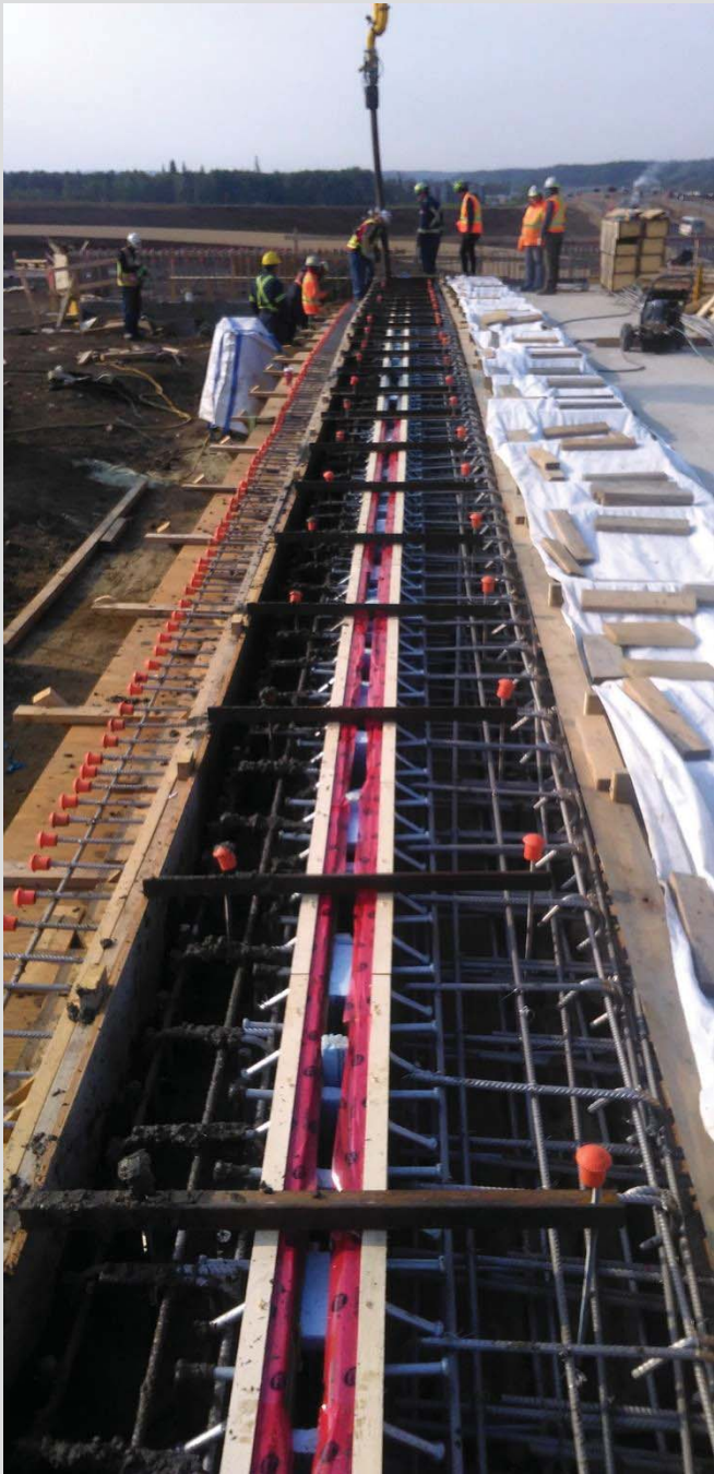
6.18 Casting abutment side of strip seal deck joint.
