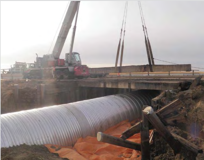
21.3 Concrete box girder salvage.
