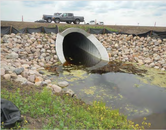
18.25 Completed collar and heavy rock riprap.
