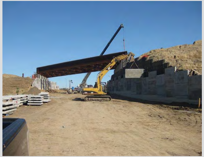
25.28 Installation of 2 nd stage panels after settlement has occurred at Stage 1.
