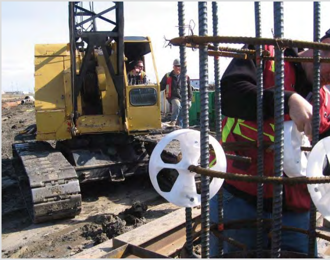
3.32 Wheel spacers are used to maintain required cover for pile cages.
