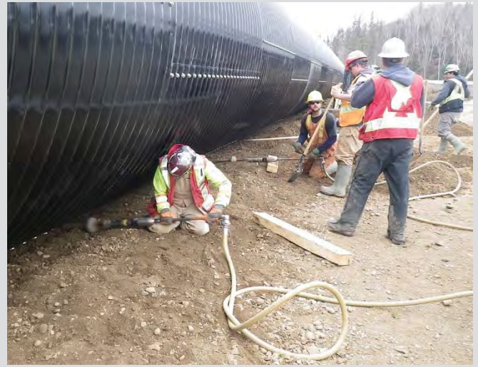
18.6 Compacting haunch area using air tampers (pogo sticks).
