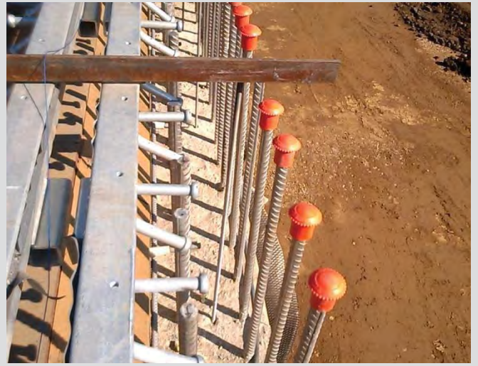
6.17 Abutment side coil rod supports shown.
