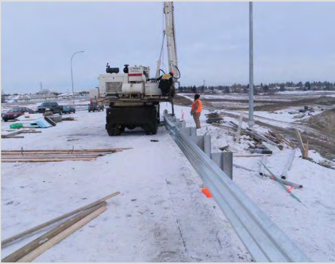
14.9 Post installation drilling.
