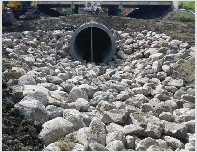
26.14 Completed placement of heavy rock riprap.
