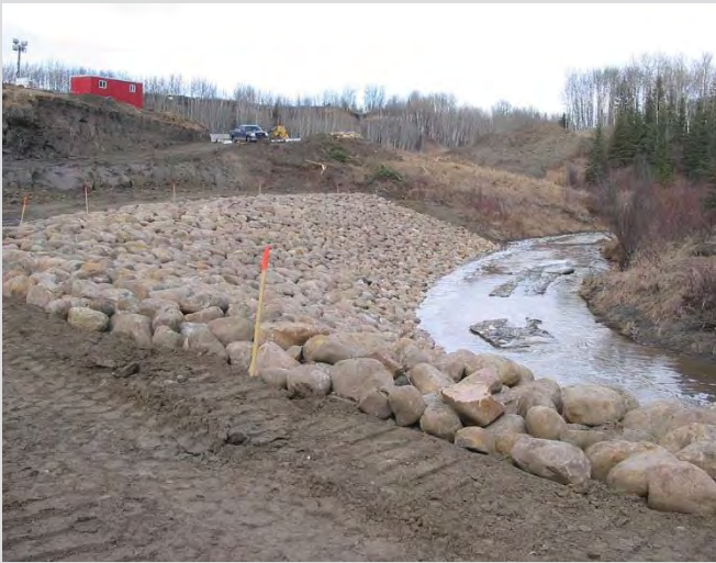
10.9 Completed installation of heavy rock riprap as channel armouring.
