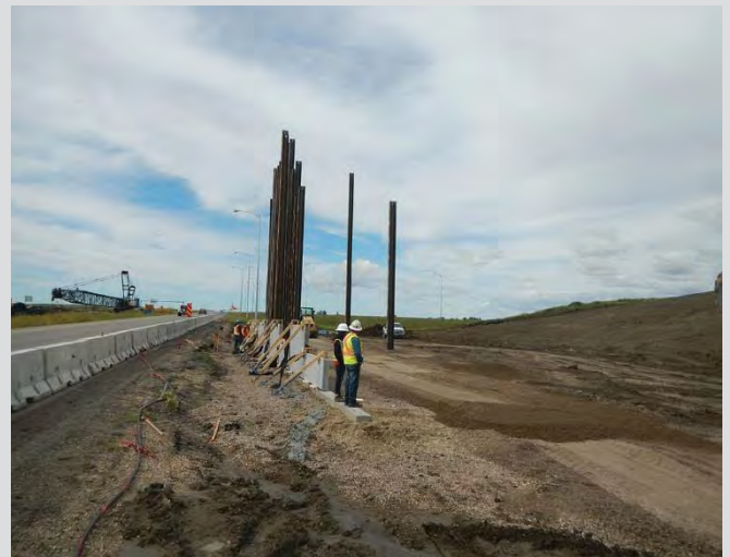
25.4 Installation of first row of precast panels on the levelling pad.
