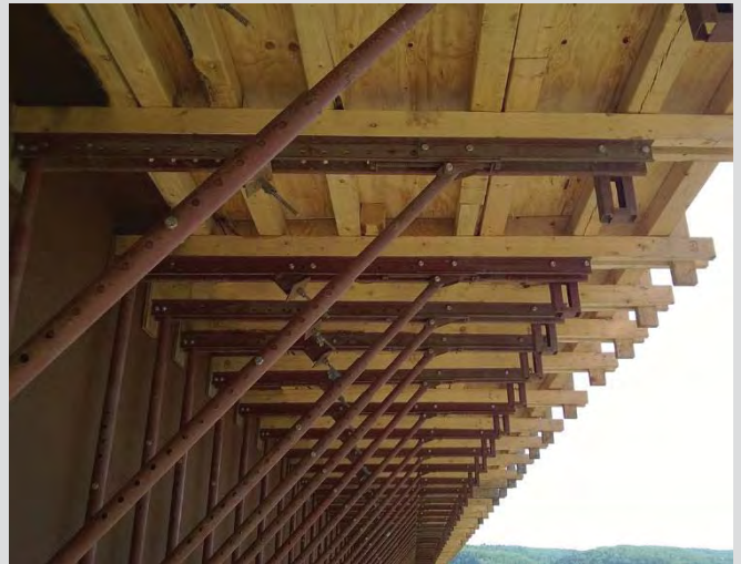
4.42 Typical deck overhang formwork, also showing hanger rods.
