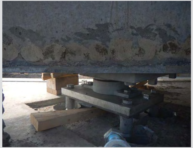
7.10 Concrete box girder on pot bearing.
