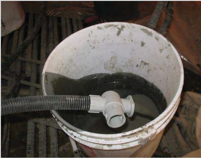
7.36 Grout sampled for testing.
