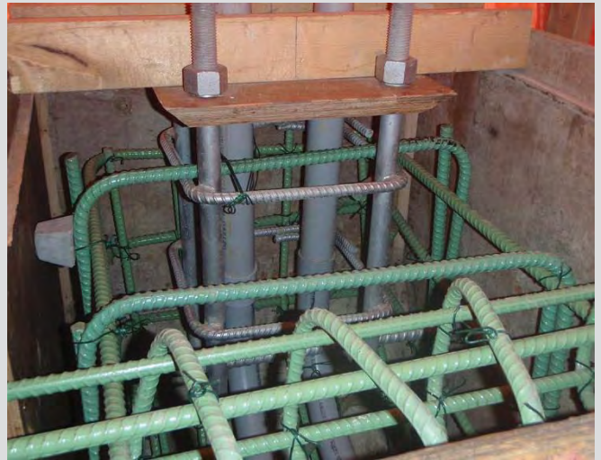
11.4 Ducts in barrier for overhead lighting.
