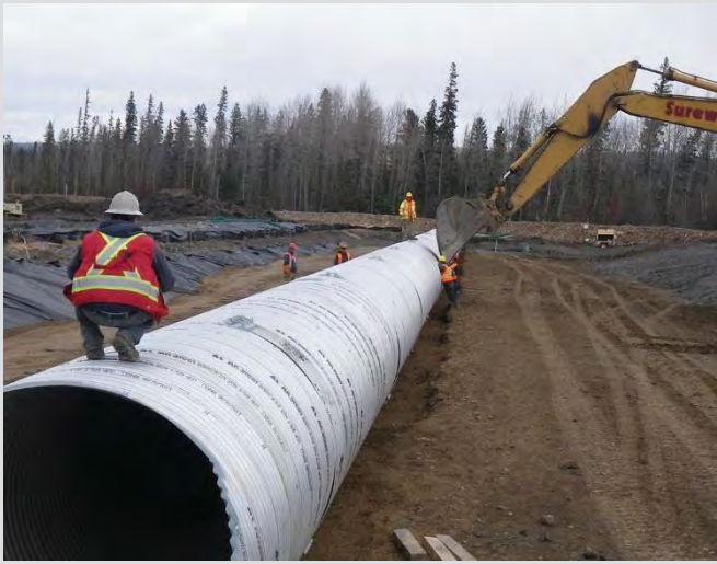
18.29 Installation of CSP structure. Backfilling and compaction at haunches.
