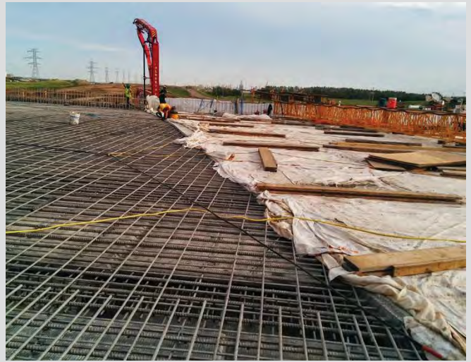
4.72 Curing material placed. Dunnage used to hold wet cure in place.
