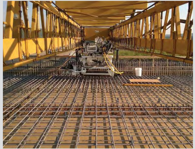
4.48 Finishing machine rail and chain system for carriage shown.
