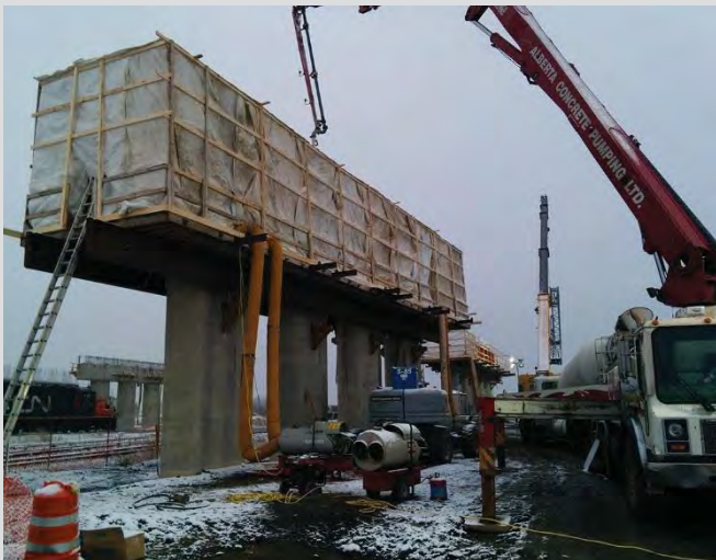
4.29 Cold weather concreting. Hoarding for pier cap pour.
