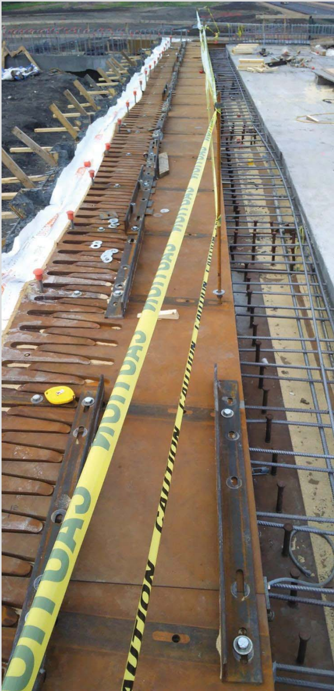
6.20 Finger type joint showing deck-side block-out.
