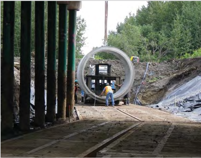
26.5 Placing first section of RCP.
