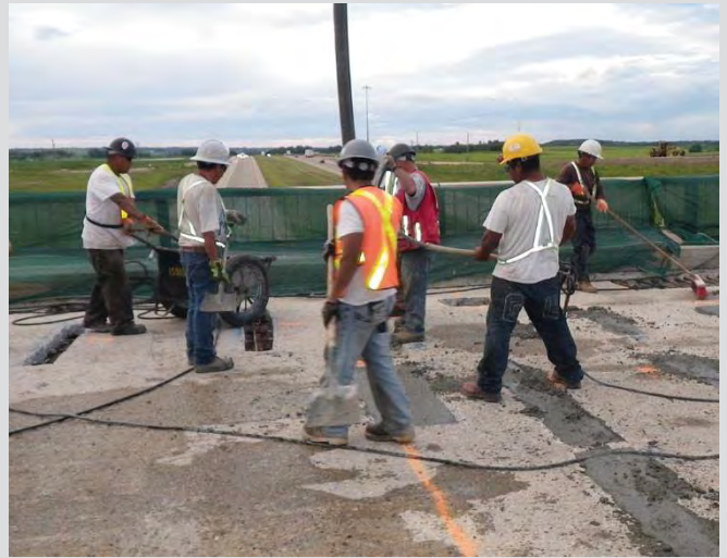
20.10 Concrete being placed into repair area.
