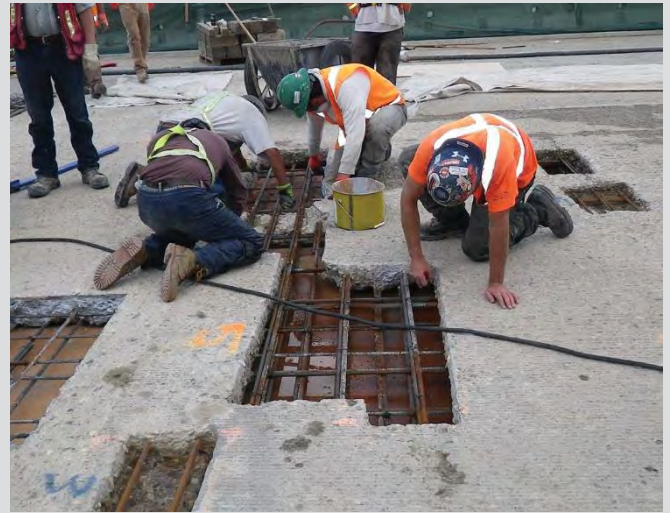
20.6 Crew preparing repair areas.
