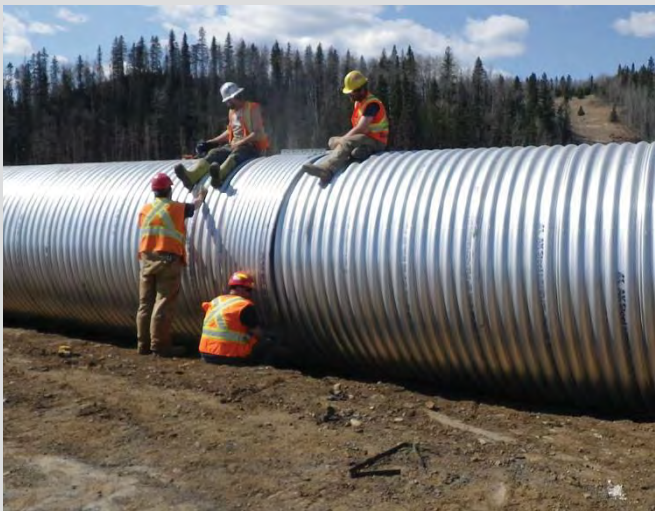
18.31 Installing CSP couplers.
