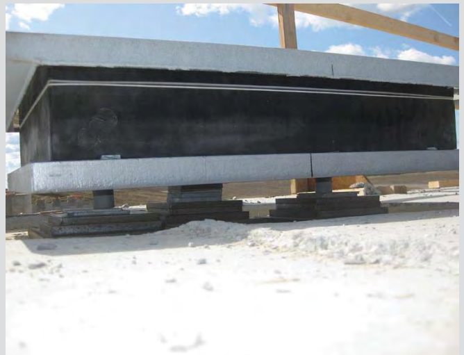
8.8 Bearing set to elevation.
