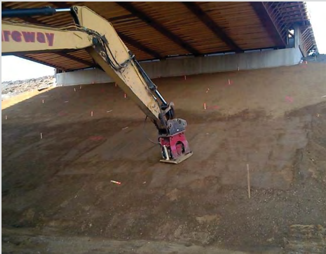
4.107 Headslope compaction with hydraulic excavator.
