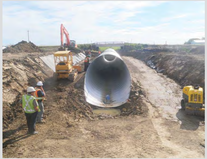
2.10 Backfill placed at culvert haunches.
