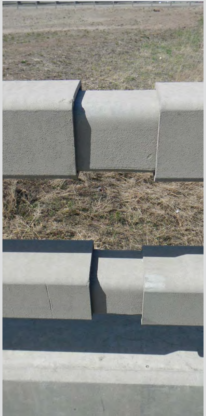
12.3 Expansion joint sleeves between rail sections.
