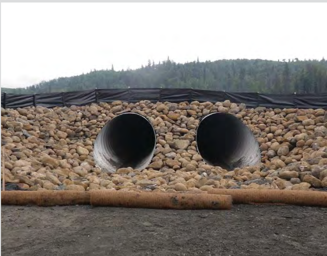
18.35 Completed culvert outlet.
