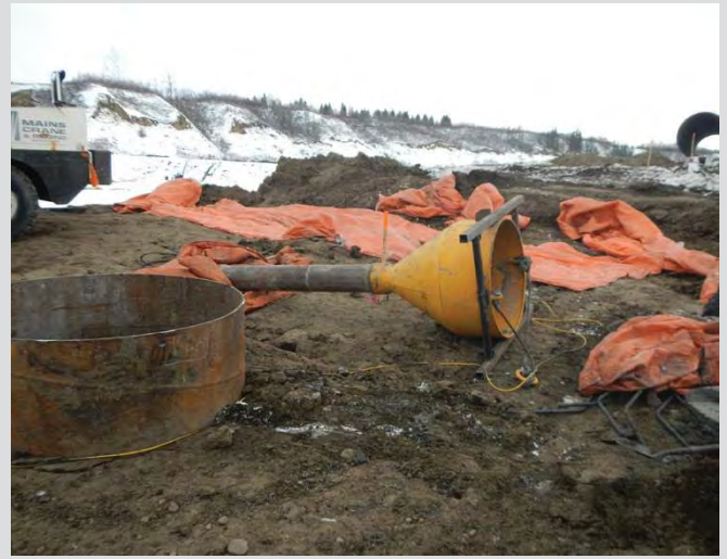
3.33 Concrete hopper for discharging concrete through pile cage.
