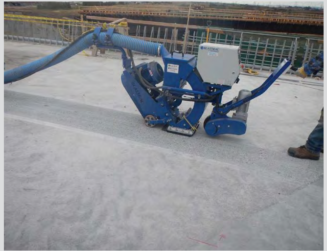
16.2 Deck surface preparation by shot-blasting.
