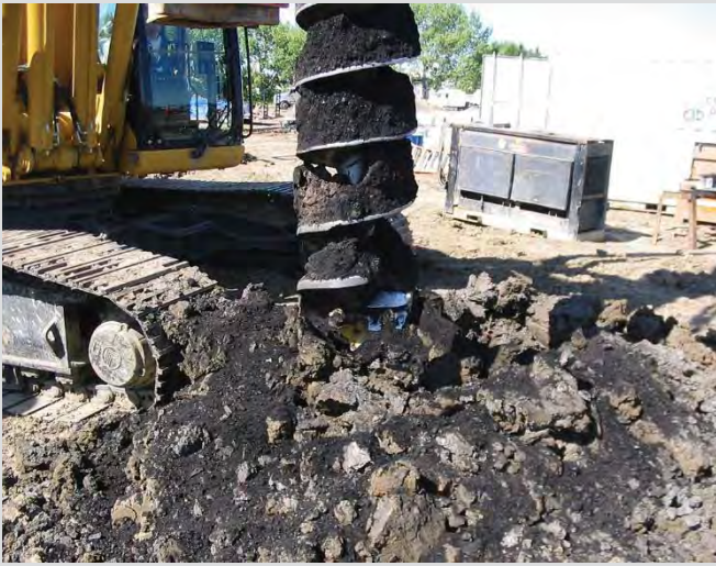
3.13 Piling rig with auger and soil tailings.
