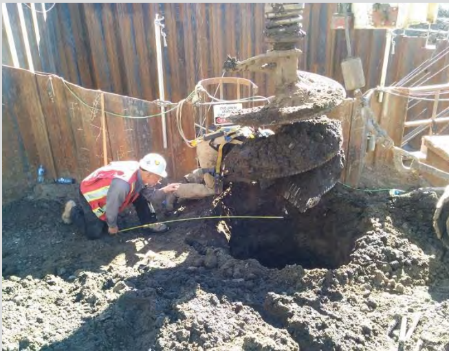
3.18 Drilling auger and tailings. Offset measurement used to confirm pile location.
