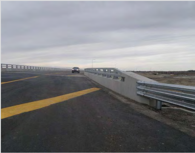
14.1 Guardrail to bridgerail transition.
