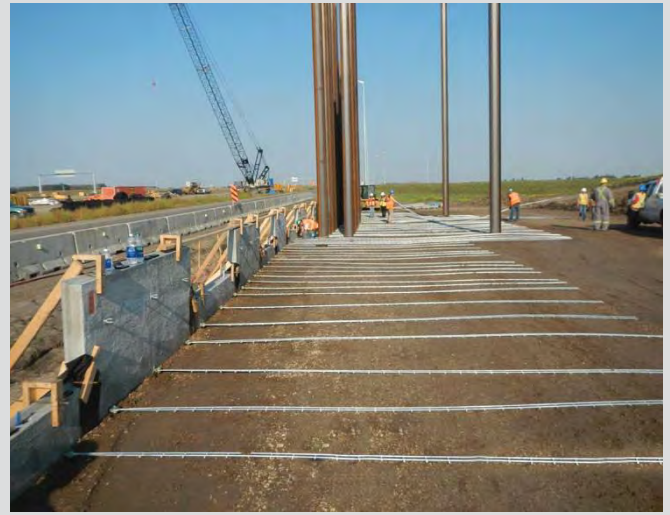
25.6 Installation of soil reinforcement.
