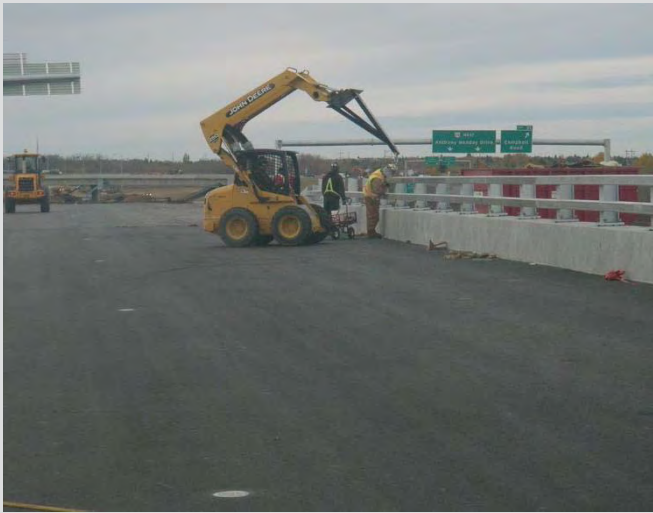
12.1 Installation of bridgerail. Bolting railing to posts.
