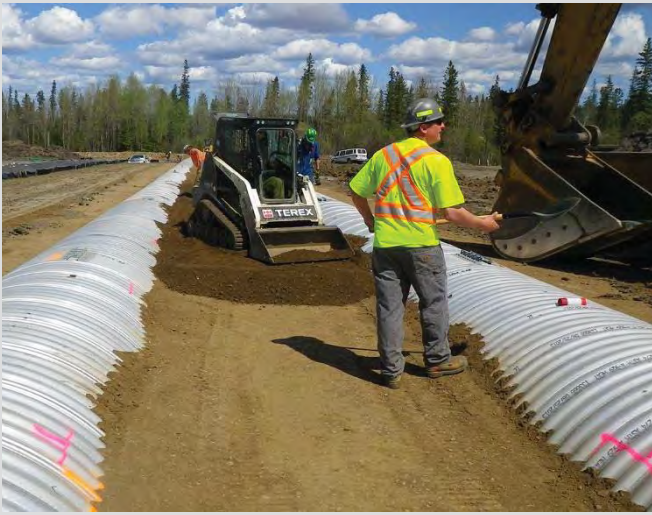
18.33 Small equipment spreading granular backfill material between culverts.
