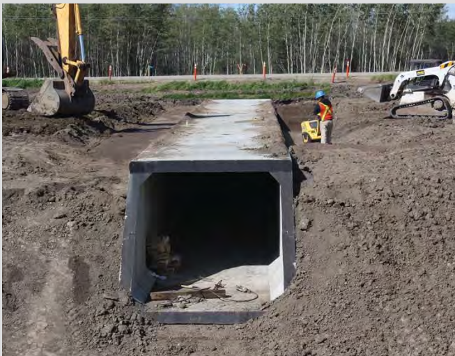
26.19 PCB culvert backfilling operation.
