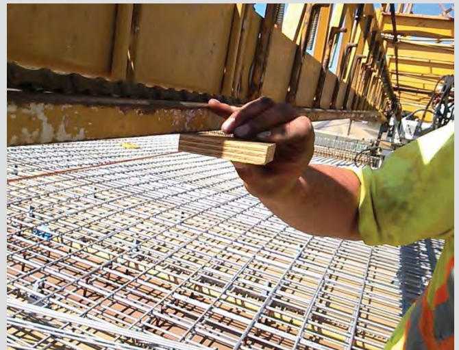
4.50 Carriage rails checked for cross-fall after adjustment.
