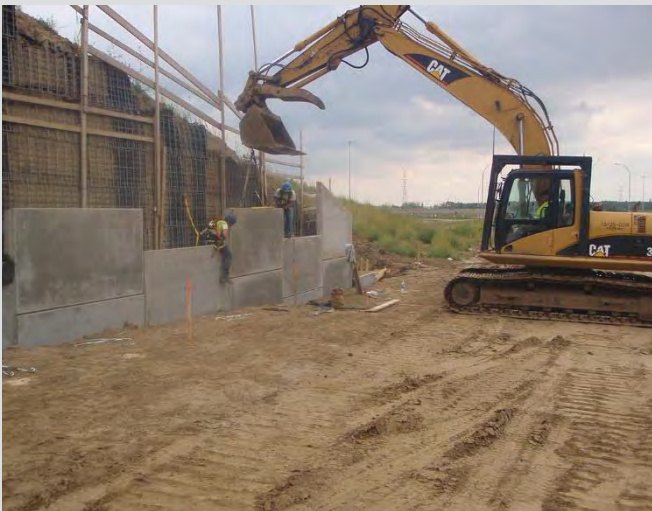
25.29 Installation of 2 nd stage panels.
