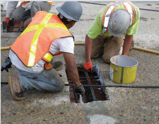
20.7 Bonding agent applied to full depth repair area.
