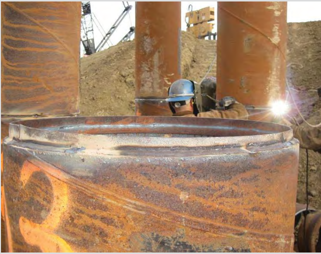
3.24 Splicing pipe pile. Bevelled edge with backing plate shown.
