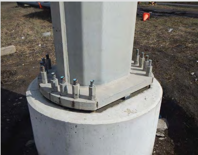
24.7 Sign structure base prior to grouting.
