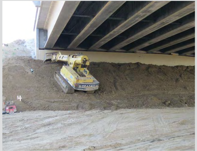
4.106 Preparation of headslope with telescoping boom excavator.
