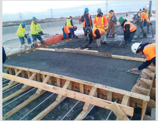
4.85 Median pour. Wooden strike off board built to maintain desired profile.
