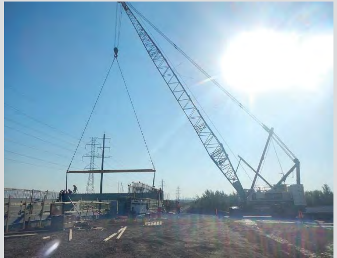
7.12 Erecting concrete box girders from approach fill.
