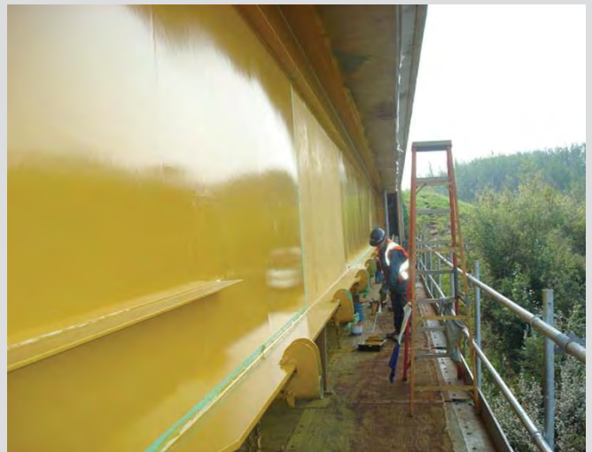
22.8 Applying finish coat of paint.
