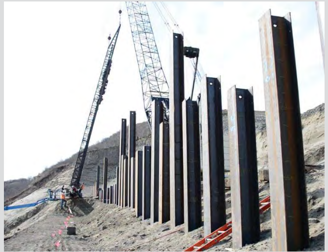
3.2 Diesel hammer and crane showing “hanging” leads.
