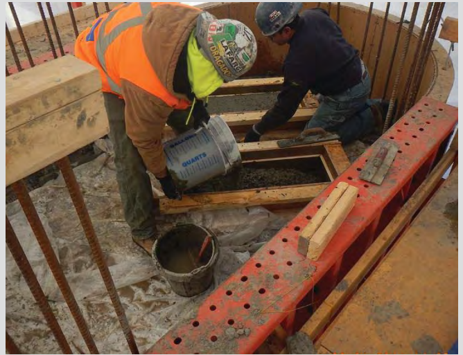
8.13 Bearing plinths for girders cast into pier diaphragm.
