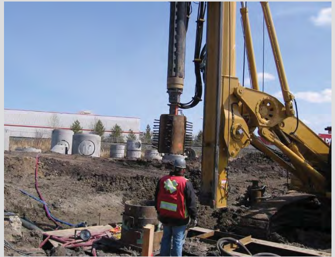
3.29 Wire brush clean up bucket attachment.
