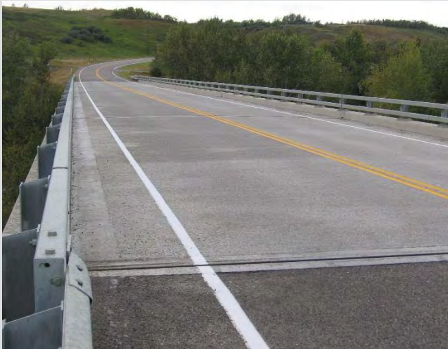
19.3 Shoulder and centreline paint lines.
