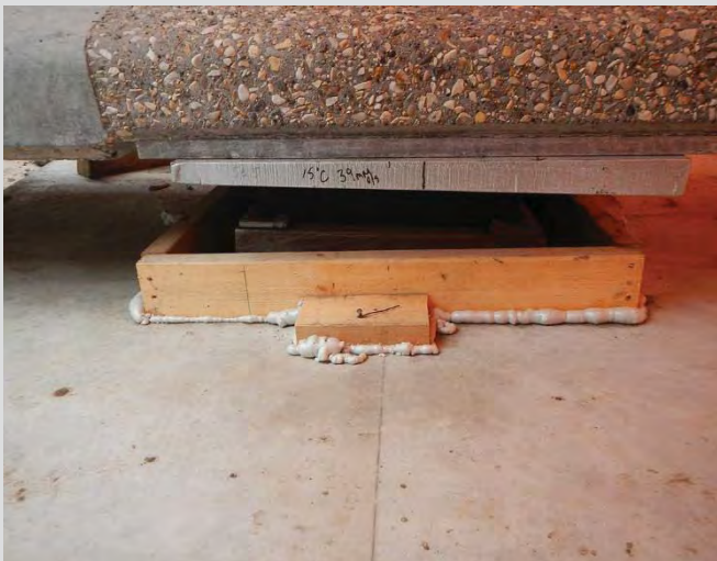
8.21 Bearing pad form work for grouting.
