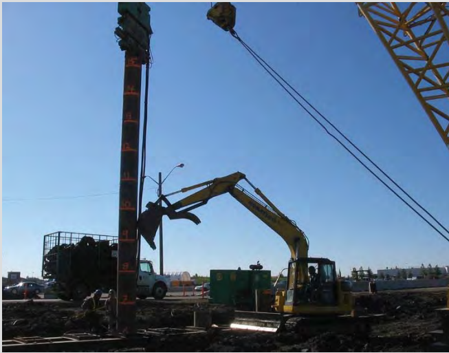
3.28 Vibratory hammer used to advance drilling casing.
