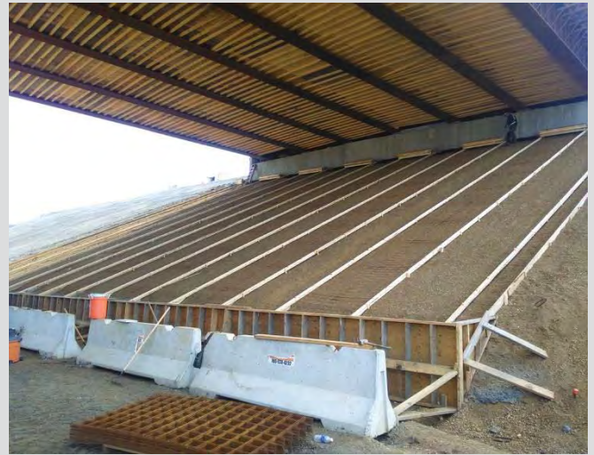
4.110 Forming of vertical concrete slope protection courses.
