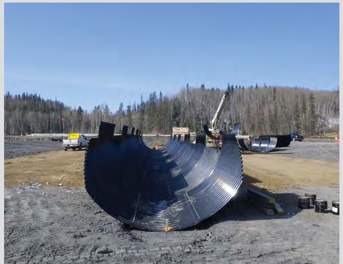
18.4 Assembling SPCSP culvert.
