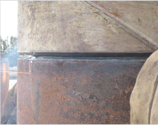
13.5 Pipe pile splice ready for field welding.
