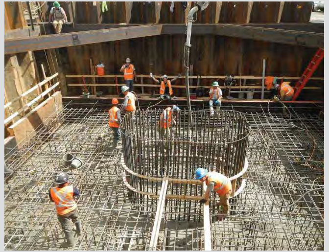
4.20 Pile cap ready for concrete placement.
