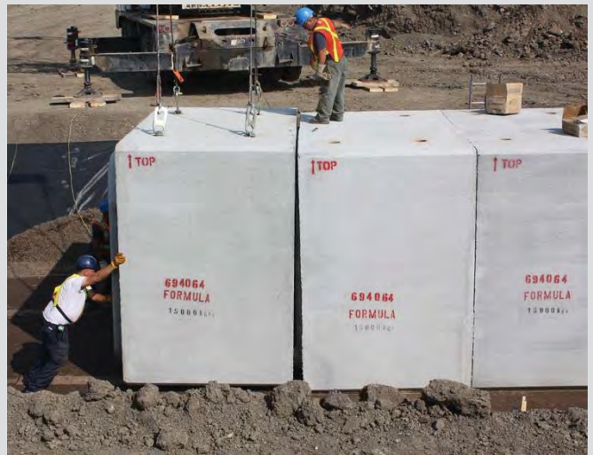
26.16 Erection of PCB unit.
