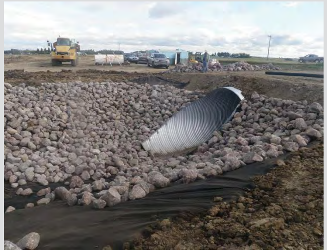
10.4 Riprap placed at the end of culvert level.
