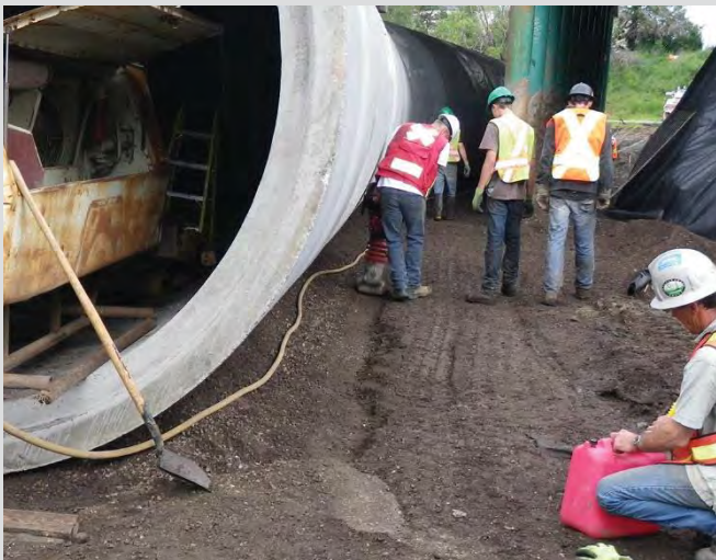
26.11 Compacting haunch area with a rammer.
