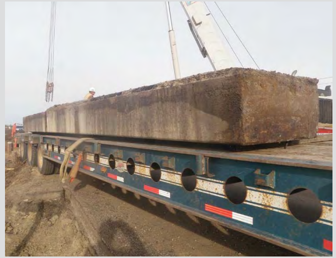
21.2 Concrete box girders salvaged. Girders lifted at their bearing points.
