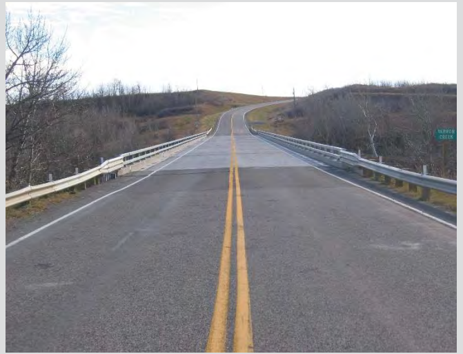
19.2 Shoulder and centreline paint lines.
