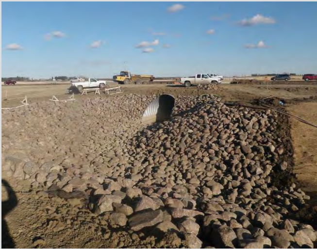
10.5 Heavy rock riprap at culvert level.
