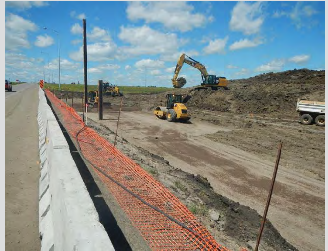
25.2 Ground improvement excavation. Soil was removed since it was not competent.
