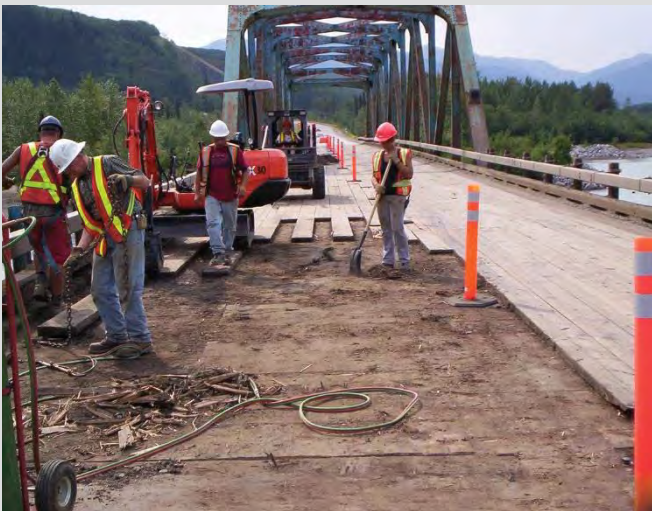
23.3 Strip deck replacement ongoing.
