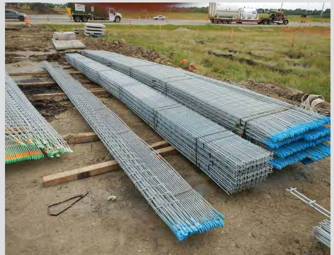
25.26 Soil reinforcement stored on timber blocks. Colour system used to identify reinforcement gauge.
