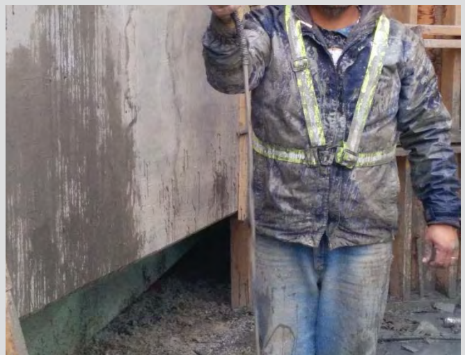
7.35 Once grout flow is confirmed at all vents, caps are closed.
