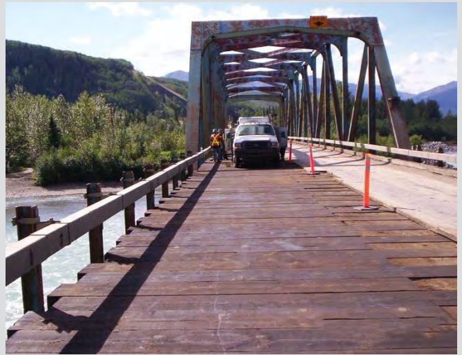
23.2 Strip deck partially removed.
