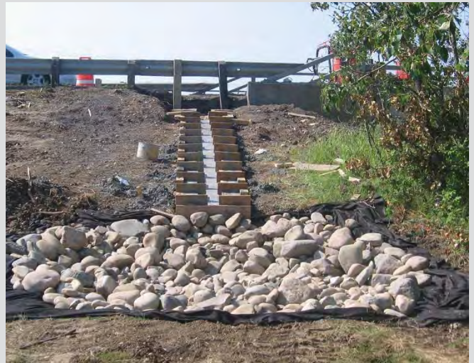
9.4 Drain trough with riprap terminal protection.
