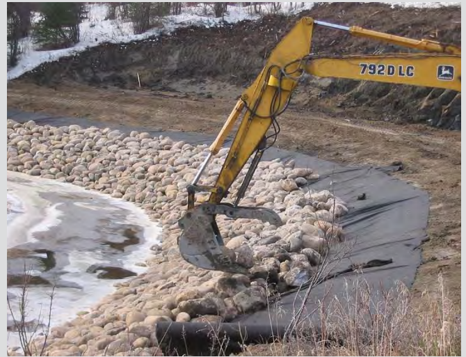
10.10 Placement of heavy rock riprap, starting from base and working upwards.
