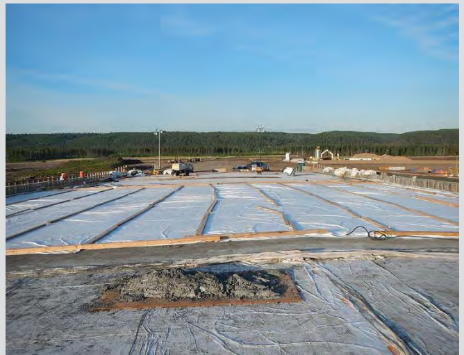
4.70 Dunnage is used to secure filter fabric.
