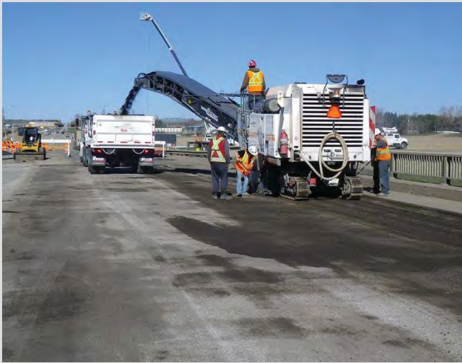
20.1 ACP milling operation.
