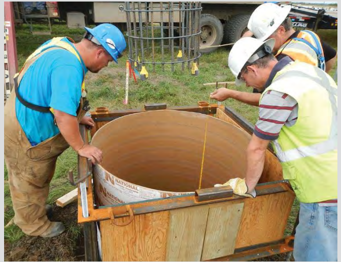
24.2 Checking depth of pile.
