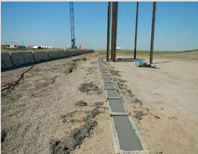
25.3 Levelling pad poured.
