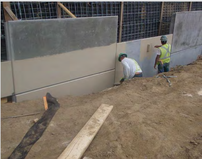
4.94 Applying pigmented sealer to MSE wall fascia panels below grade.
