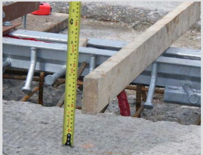
20.16 Checking deck joint elevation.
