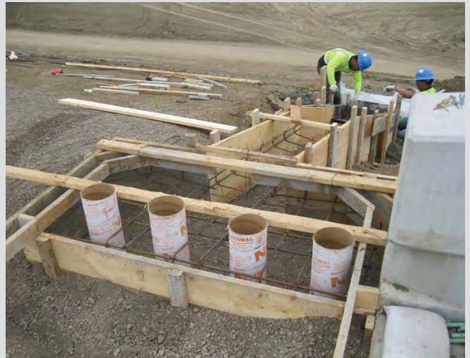
14.4 Guardrail transition post holes in concrete drain trough take off.
