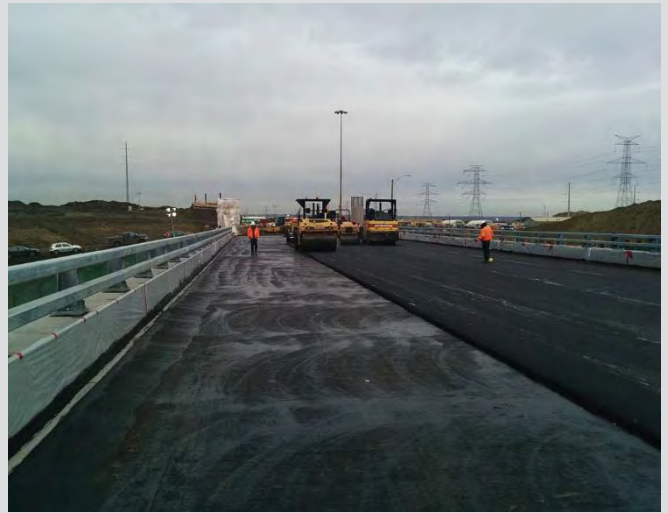
17.6 Large smooth drum and rubber tired rollers used to compact ACP.
