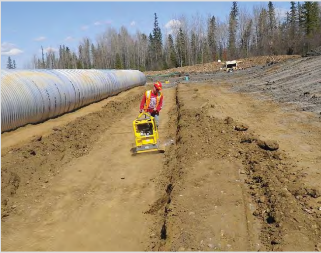
2.9 Compaction of bedding.
