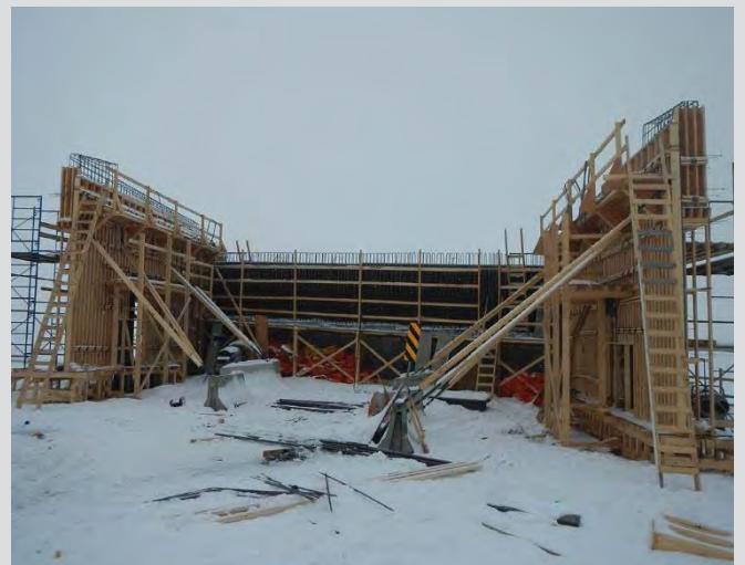
4.7 Partial wingwall and backwall formwork.
