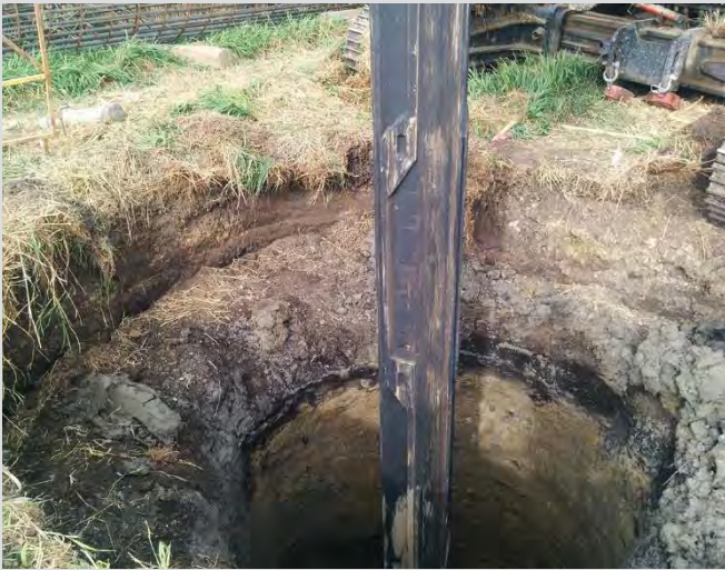
24.1 Drilling foundation pile.
