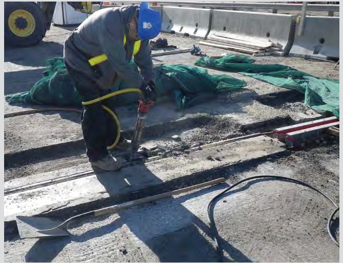
20.14 Existing deck joint removal using pneumatic hammer.
