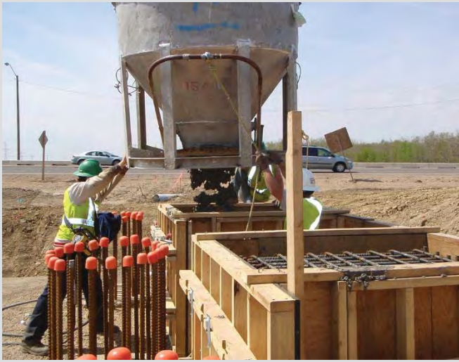
4.23 Concrete placement using crane and bucket. Freefall of concrete minimized.
