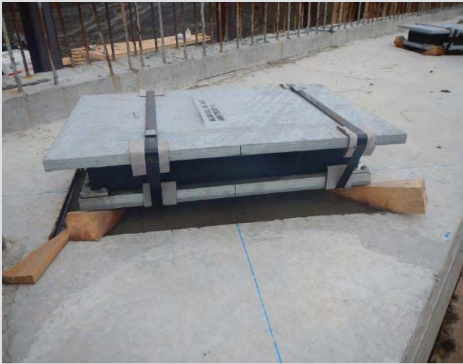
8.5 Bearing assembly centred and blocked in position.
