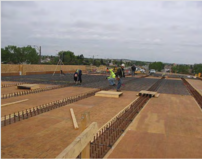
5.9 Crews tying and placing first mat of deck reinforcing steel.
