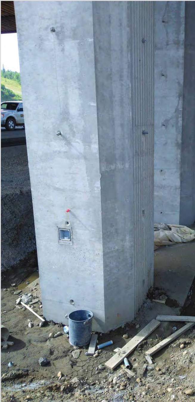
4.6 Mudslab shown at pier columns.
