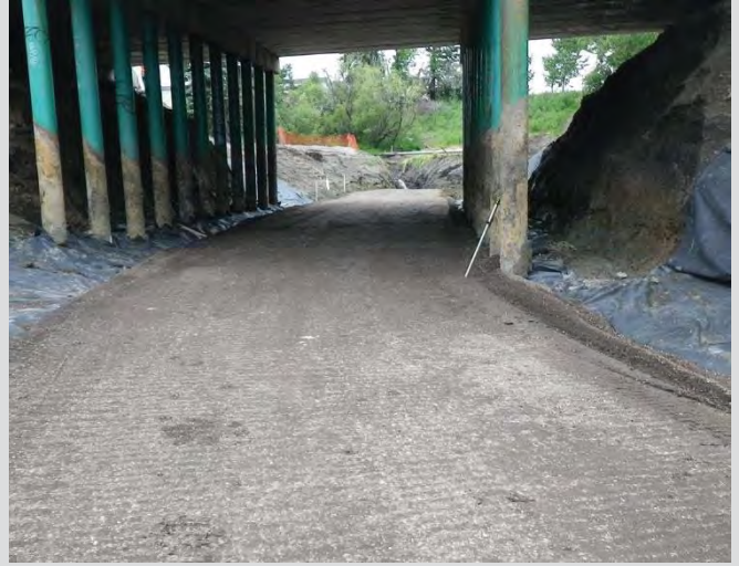
26.2 Bedding material placed and compacted.
