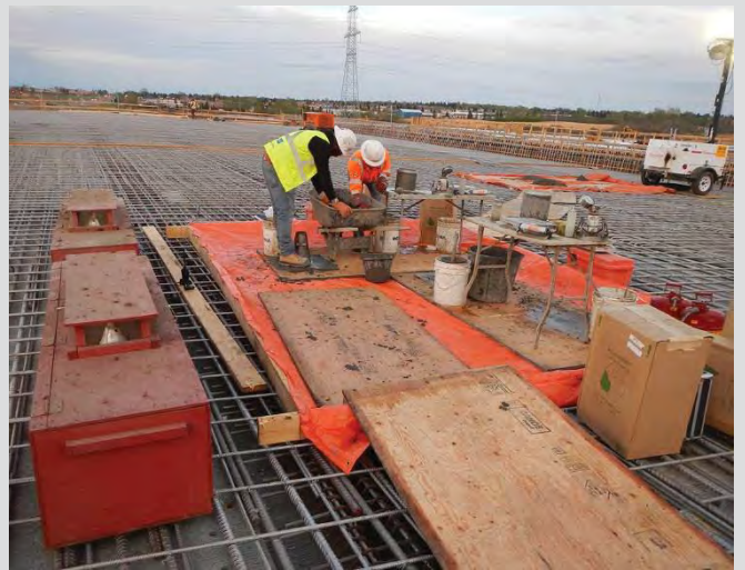
4.58 Concrete testing station set up on deck.
