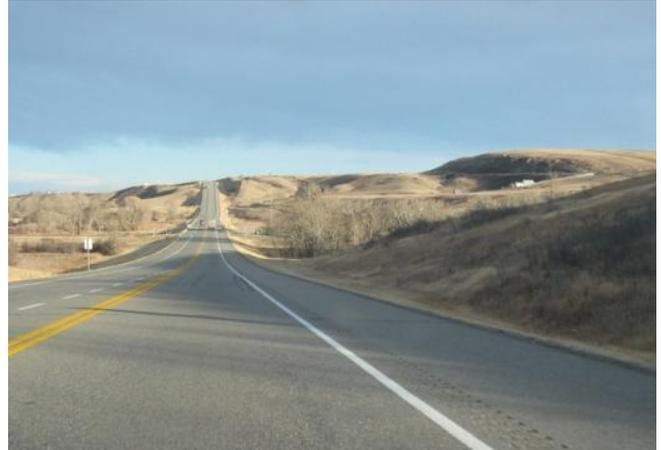
**Pincher Creek:** Rural application of wide paved shoulder with shoulder rumble strips.
