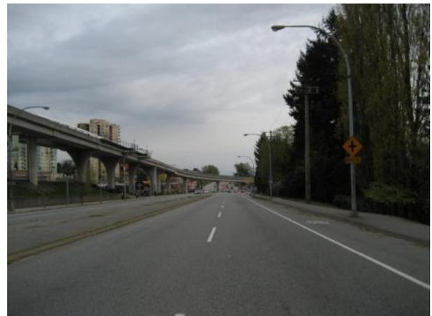
**Lougheed Highway, Vancouver:** Urban application where fixed objects are frangible (breakaway posts and small caliper trees) and separated from the travel lane by a bicycle lane and sidewalk.
