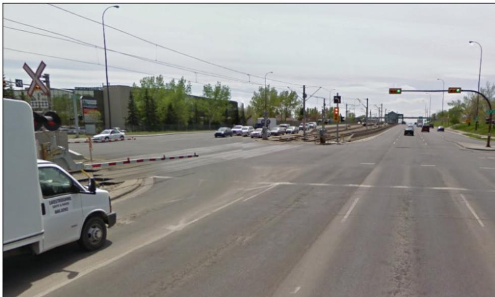
FIGURE 3.27 SINGLE LEFT-TURN LANE WITH PROTECTED-ONLY PHASING
