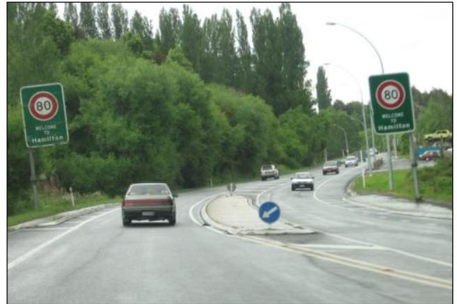
FIGURE 3.3 PHYSICAL ROAD NARROWING USING RAISED MEDIAN (NEW ZEALAND)
