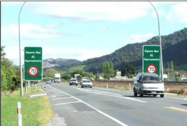
FIGURE 3.2 VISUAL ROAD NARROWING THROUGH HATCHING AND PAINTED MEDIANS (NEW ZEALAND)
