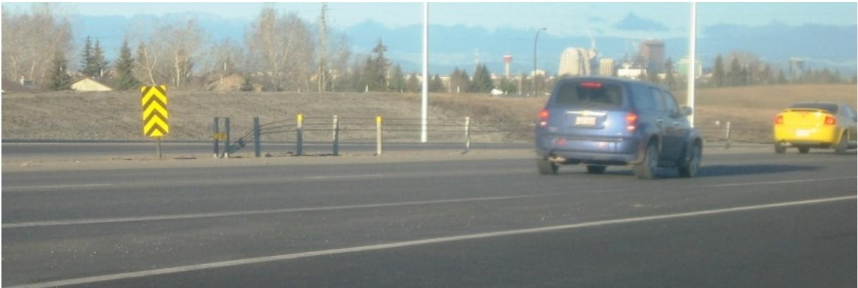
**FIGURE 3.30 CABLE BARRIER USED TO DISCOURAGE UNSAFE LANE CHANGES
