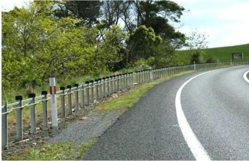
**FIGURE 3.28 EXAMPLE OF ROADSIDE CABLE BARRIER IN NEW ZEALAND**
