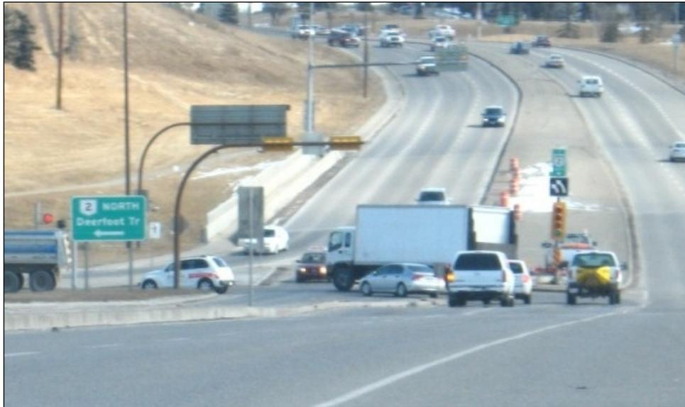
FIGURE 3.26 DUAL LEFT-TURN LANE WITH A PROTECTED-ONLY LEFT-TURN PHASE
