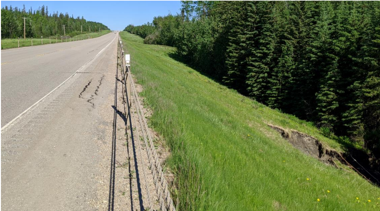
Photo No. 1 – Looking at WBL landslide; note the presence of open tension cracks on the highway shoulder; main head scarp crack of landslide is about 5.6 m from the edge of pavement
