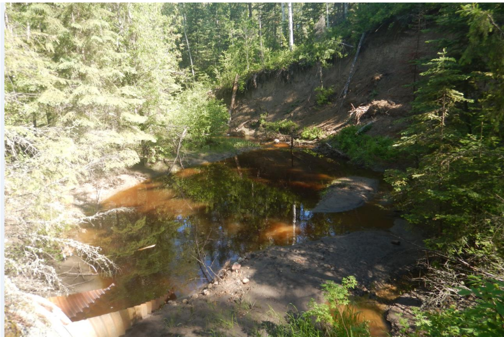
Photo No. 4. Looking northwest at the CSP culvert outlet; note silt accumulation as well as fallen trees near the culvert outlet
