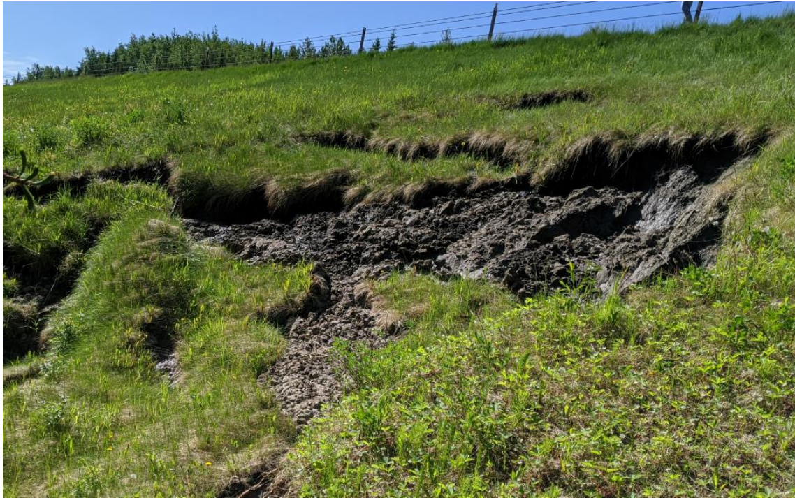
Photo No. 3 – Looking southeast at the landslide’s head scarp and eastern flank; note the presence of multiple tension cracks within the slope downslope of the highway location
