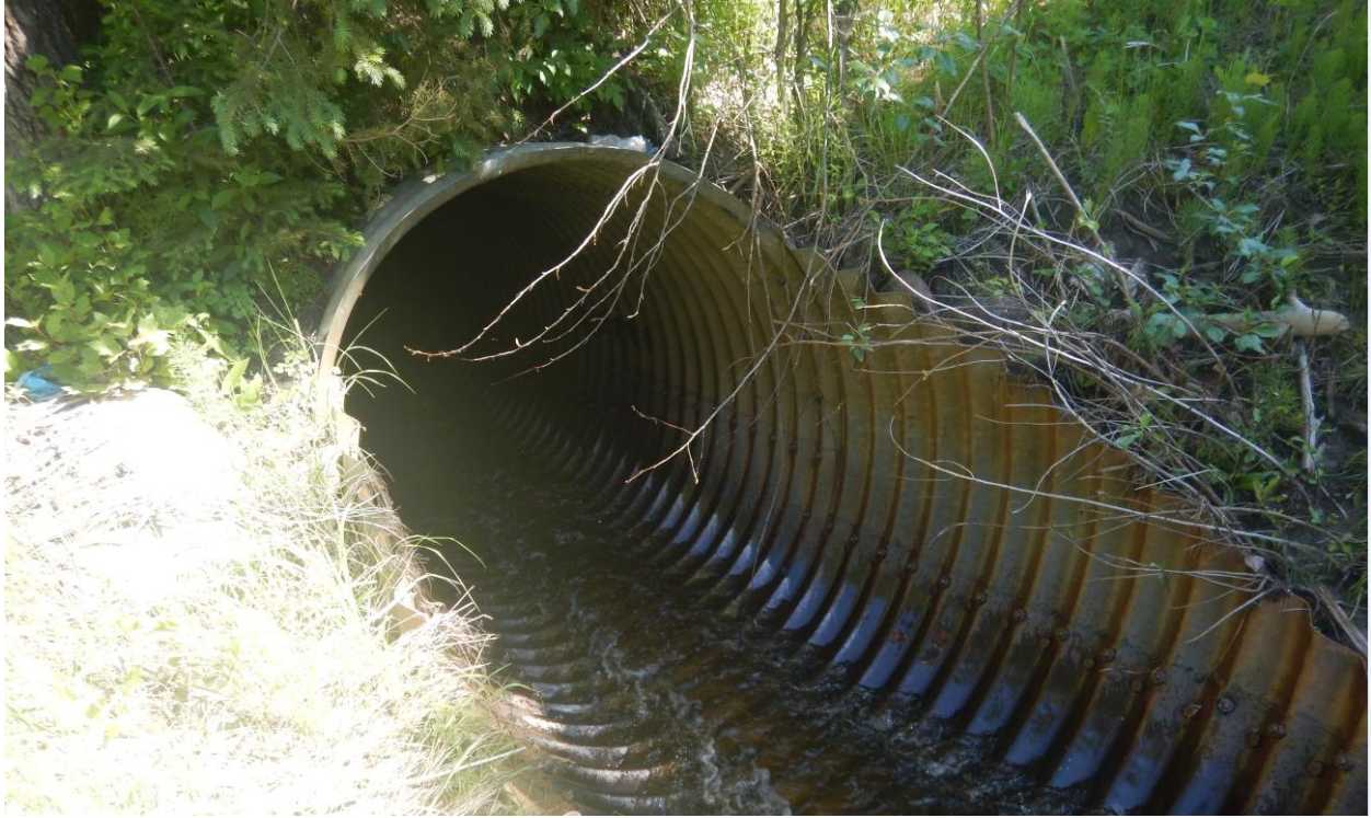
Photo No. 7 – Looking at CSP Culvert Inlet (1.9 m diameter); scattered riprap was noted at inlet location
