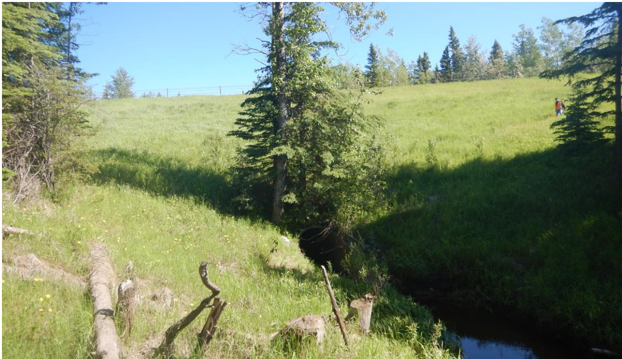
Photo No. 8. Looking north at the south side slope of the highway embankment
