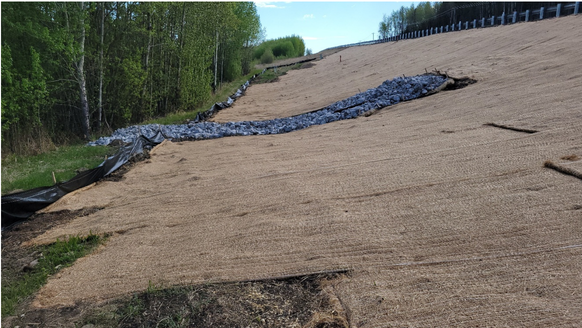
Photo 6. Looking east at the regraded downslope area. The inlet for the new 900 mm diameter SWSP culvert as well as the associated Class 1M riprap channel are visible in the foreground. Regraded slope area has been covered with Type C erosion control matting.
