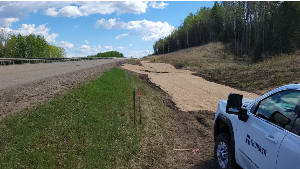
Photo 9. Looking east at the regraded upslope ditch area. Type C erosion control blanket has been placed in the ditch. The inlet to the new 900 mm diameter SWSP culvert is visible near the middle of the photo. |
