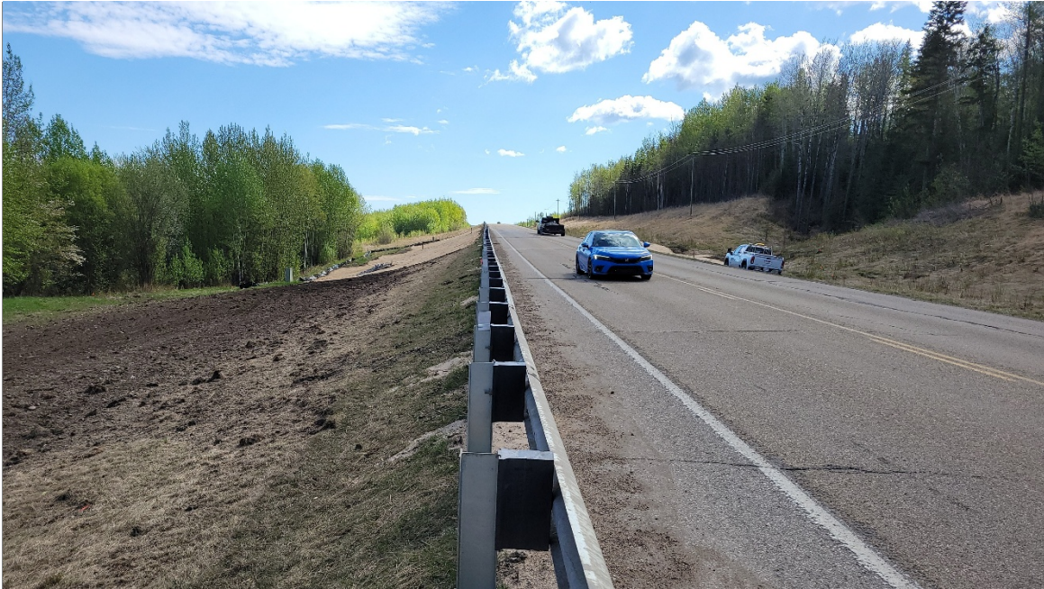
Photo 1. Looking east toward the highway side slope area regraded as part of the 2024-25 pile wall construction.
