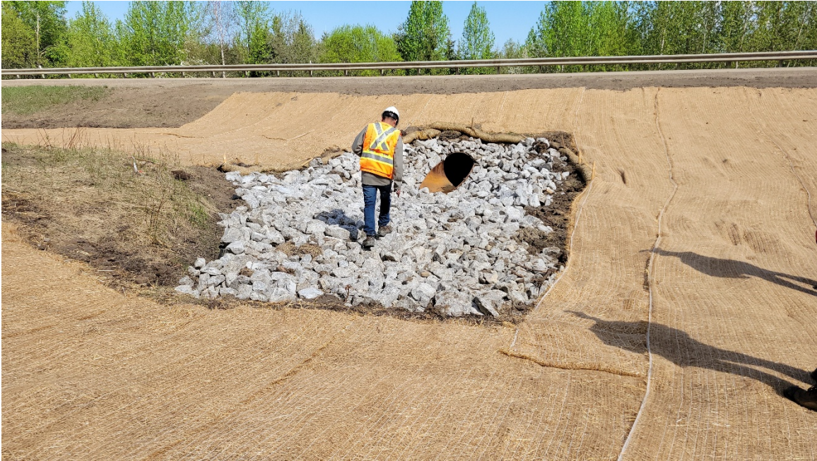
Photo 8. Inlet side of new 900 mm diameter SWSP culvert and riprap bowl.
