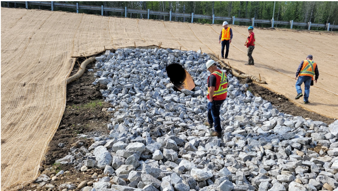
Photo 7. Outlet of new 900 mm diameter SWSP culvert and Class 1M riprap channel.
