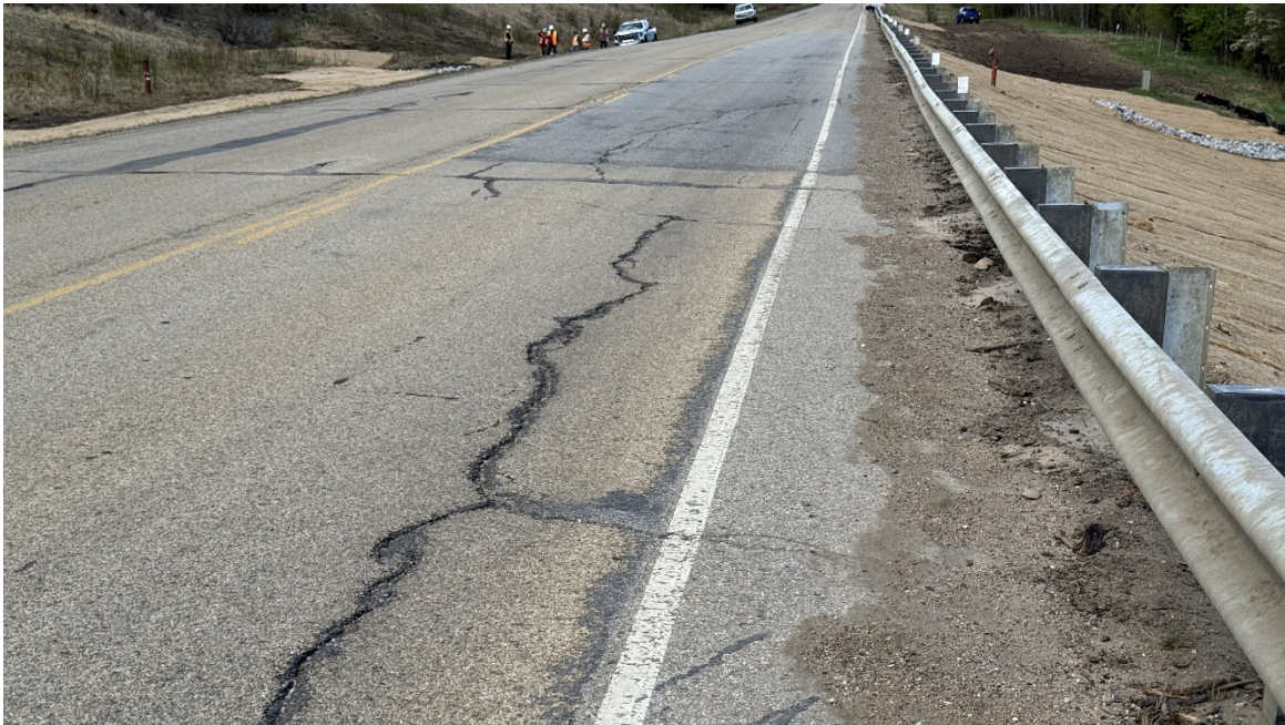
Photo 3B. (Same location as Photo 3A viewed during the current inspection). Note that the guardrail was replaced during the 2024-25 pile wall construction.
