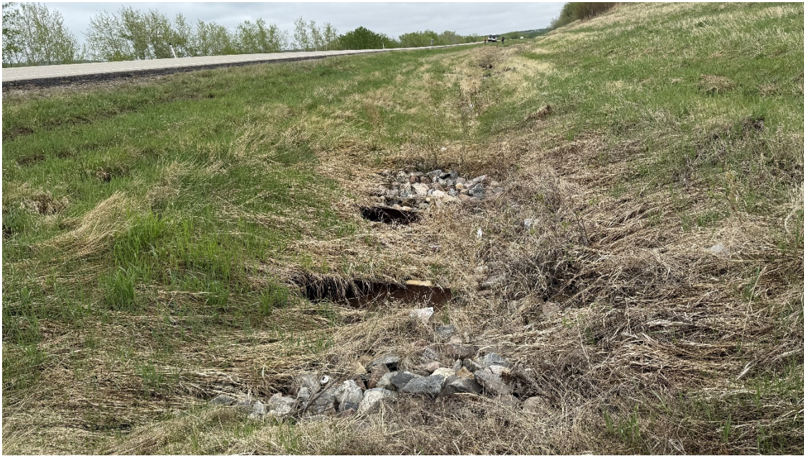
Photo 3. Looking north at the inlets of the twin culverts. No flow noted during current inspection.
