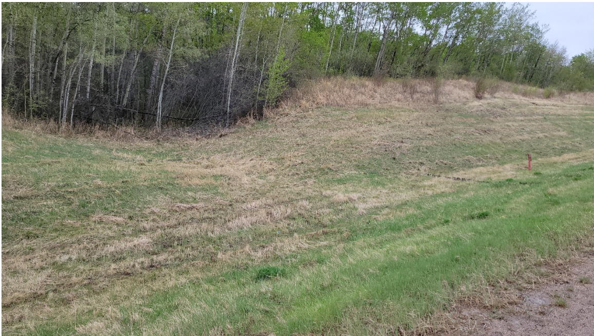
Photo 8. Looking southeast at TRM lined gully and ditch area. No flow was noted in the gully.
