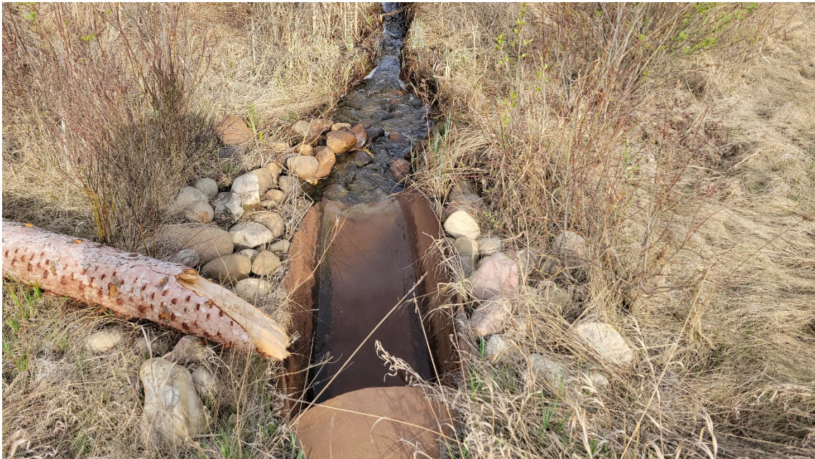
Photo 8. Looking at the outlet of the 900 mm SWSP C2 Culvert outlet. Lighter flow than noted in the 2024 inspection.
