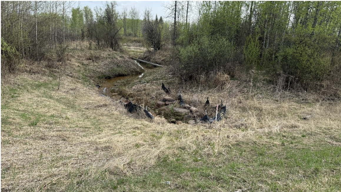
Photo 2. Looking north at Culvert C1 outlet. Water is freely flowing through the culvert and along the channel.
