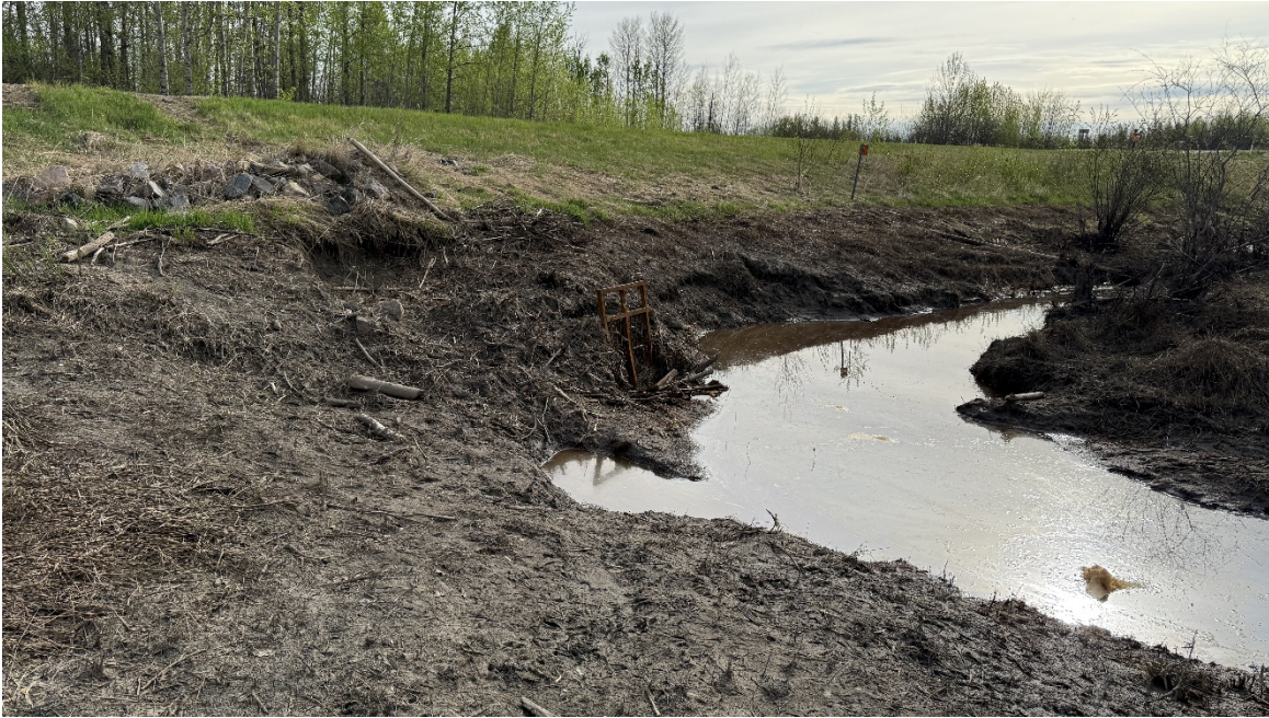
Photo 3. Looking northeast towards the inlet of CSP Culvert C1. Debris has been removed from the culvert inlet since the 2024 inspection.
