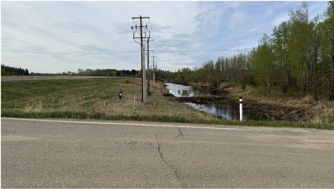
Photo 1. Looking south at Oxbow Lake. Beaver Dam 2 visible towards center of photo. Water levels behind and in front of the dam appear similar to levels noted in the 2024 inspection.
