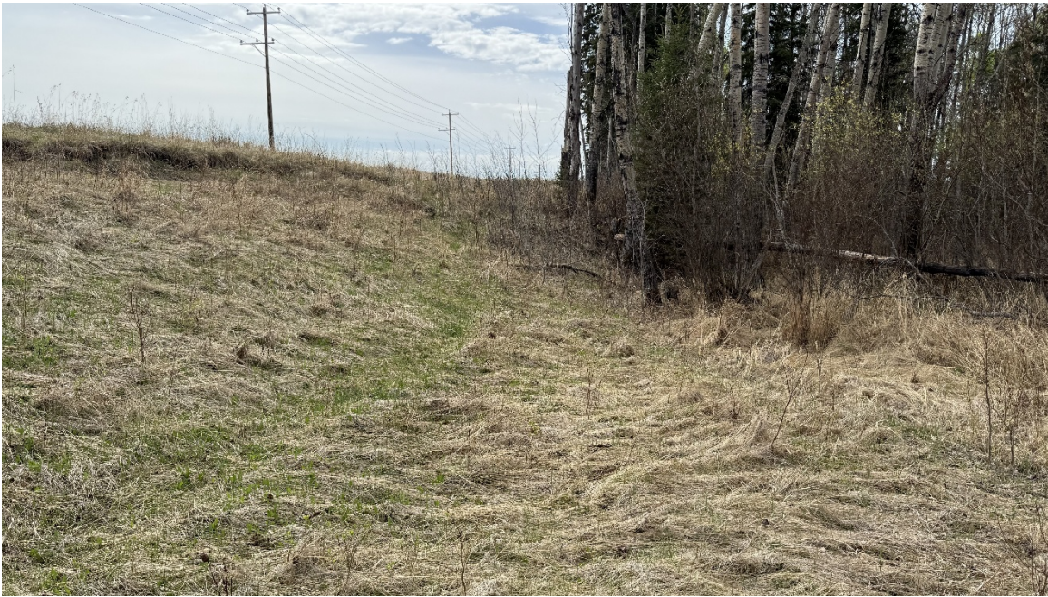
Photo 8. Looking south at the landslide south flank. Backscarp crack is 1.1 m deep and 1.2 m wide.
