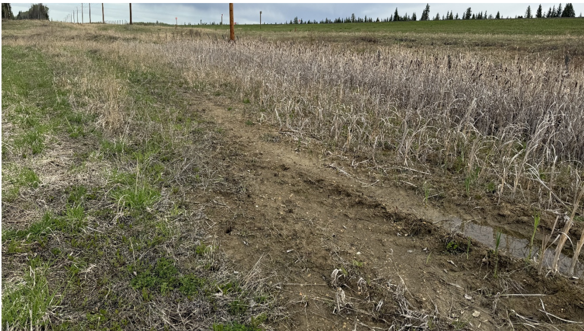
Photo 9. Looking north at the landslide's north flank. Average drop of 1.5 m to 2.0 m within landslide mass.
