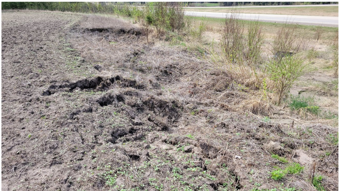
Photo 10. NC091-2: Looking southwest at erosion near the scarp crest which has retrogressed into the farmer's field.
