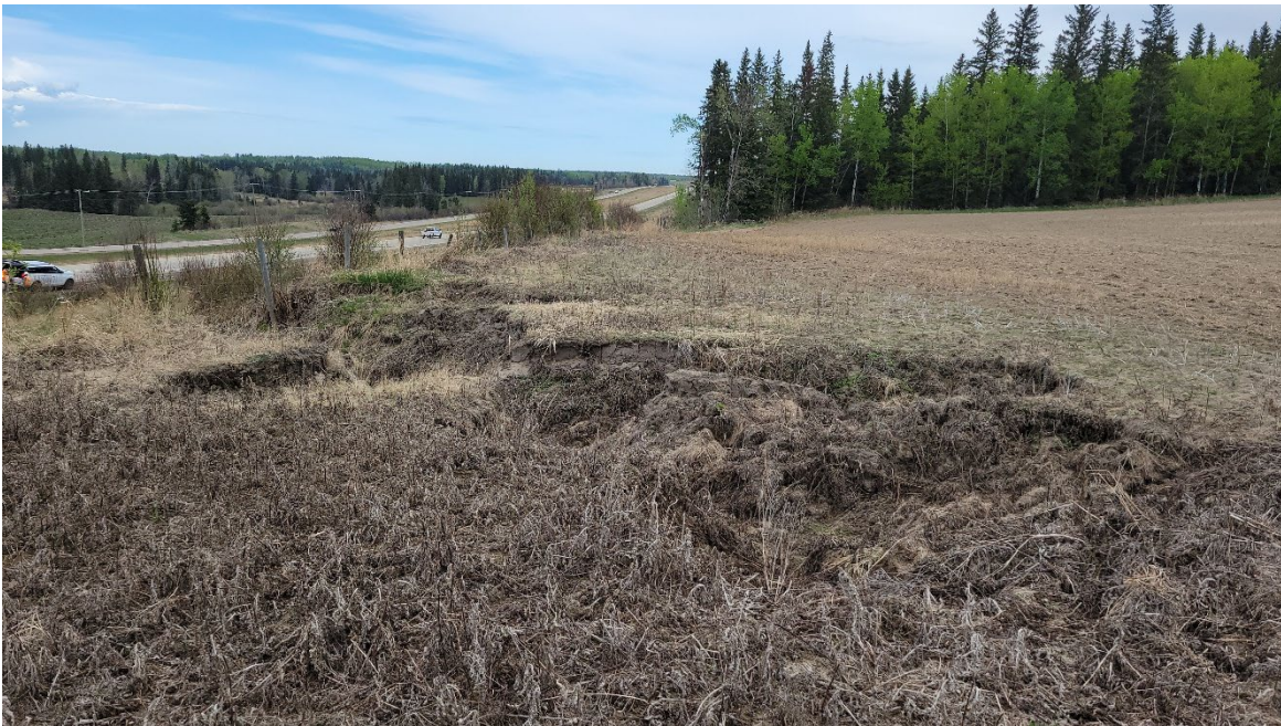
Photo 2. NC091-1: Looking northwest at the erosion gulley developed within the farmer's field. Erosion has worsened since 2024 inspection.
