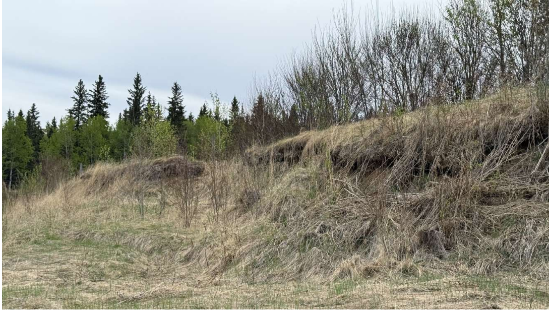
Photo 3. NC091-1: Looking north at landslide backscarp crack showing a 2.4 m drop approximately 5 m west of the upslope ditch.
