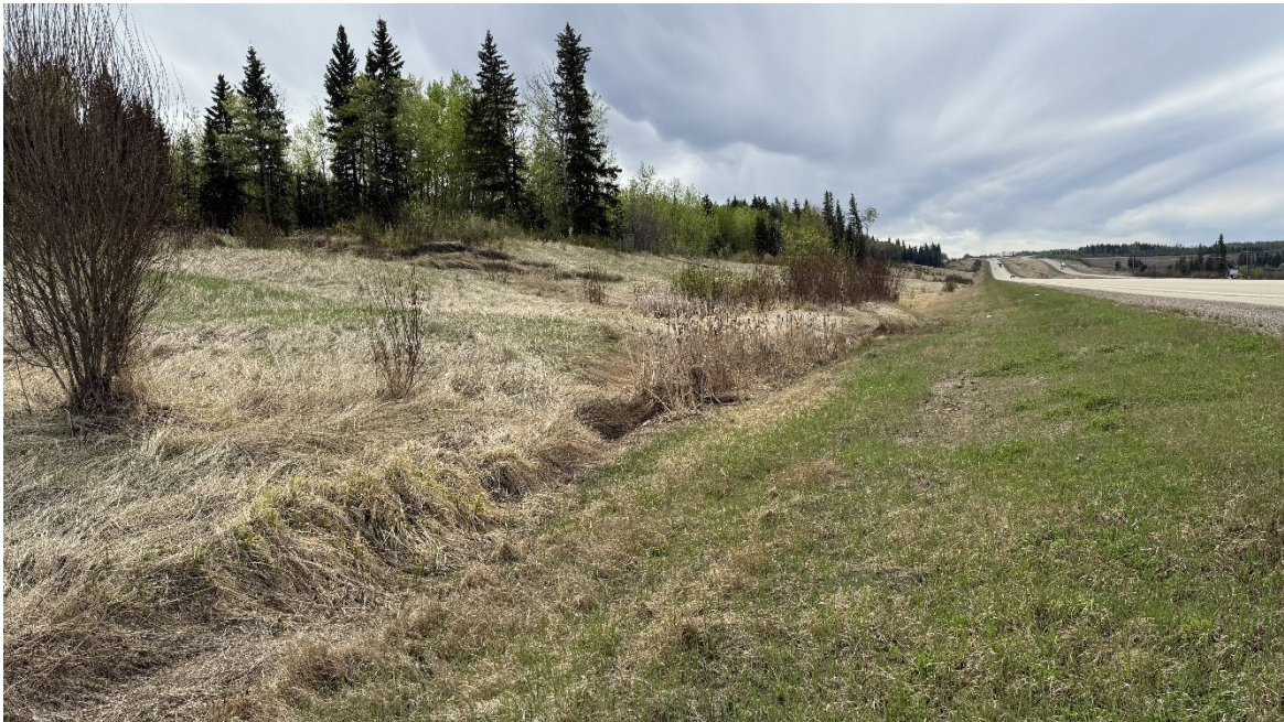
Photo 8. NC091-2: Looking south at the landslide mass; note the distinct toe roll in the ditch and the presence of multiple tension cracks within the backslope.
