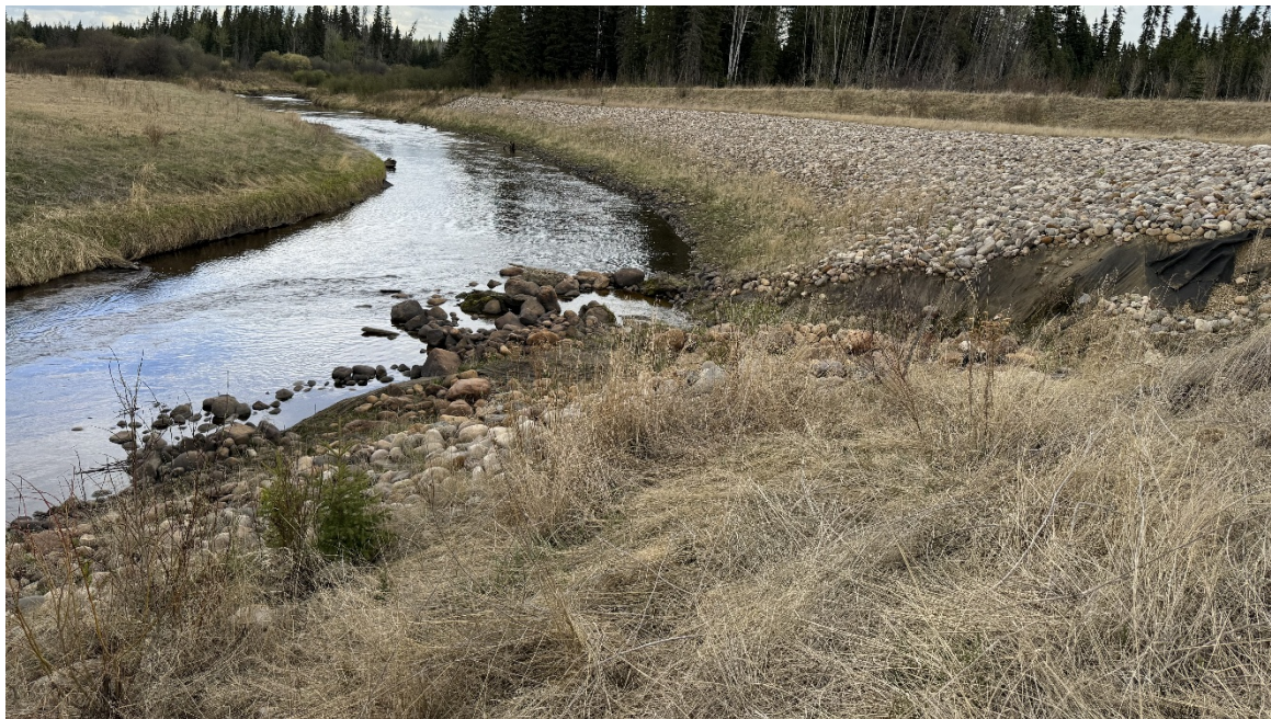
Photo 2. Looking northeast at the north facing riprap channel to the east of the bridge location.
