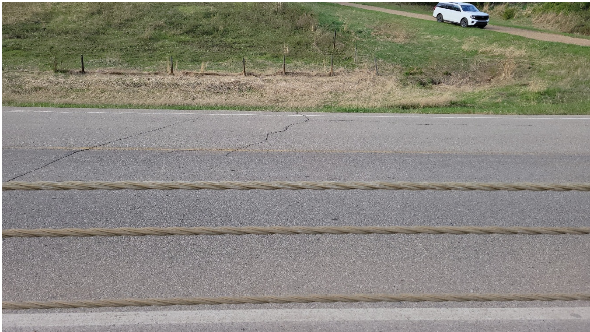
Photo 3. Looking north at a transverse crack (15-20 mm wide with no drop).
