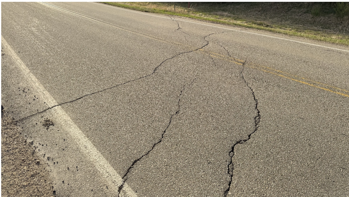
Photo 4. Looking northwest at the eastern flank reflective diagonal cracks (up to 50 mm wide with 20 mm drop).
