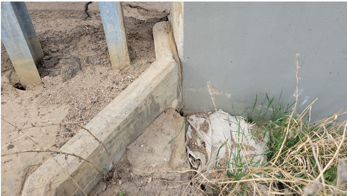
Photo 8. South drain trough. The gap between the drain trough and wing wall was sealed with a flexible filler.
