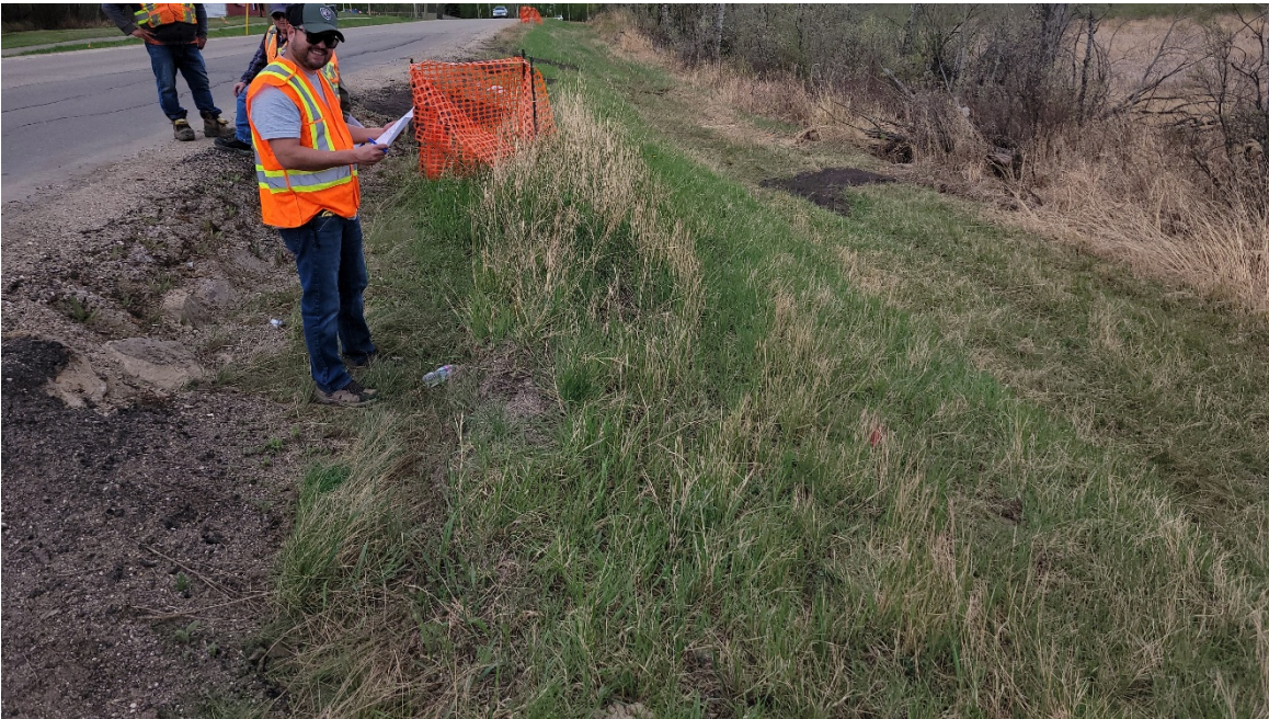
Photo 4. Southern flank of the landslide (looking south); 600 mm drop visible from the highway. Note the topsoil patch at the right-hand side of the photo where Anchor Power Pole No. 3 was removed after the 2024 inspection.
