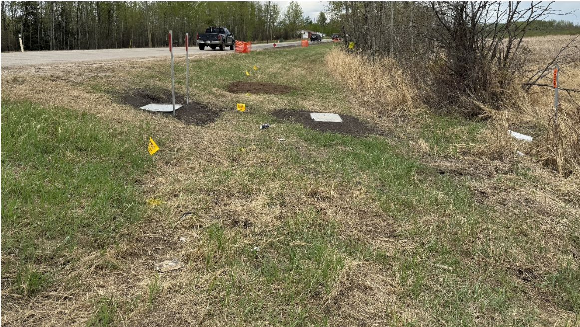
Photo 7. Looking south from the west side of the highway. Two utility boxes are visible where the fibre optic lines have been rerouted to the west side of the highway. The Apex Utilities gas line has also appear to have been rerouted across the highway at this location. |
