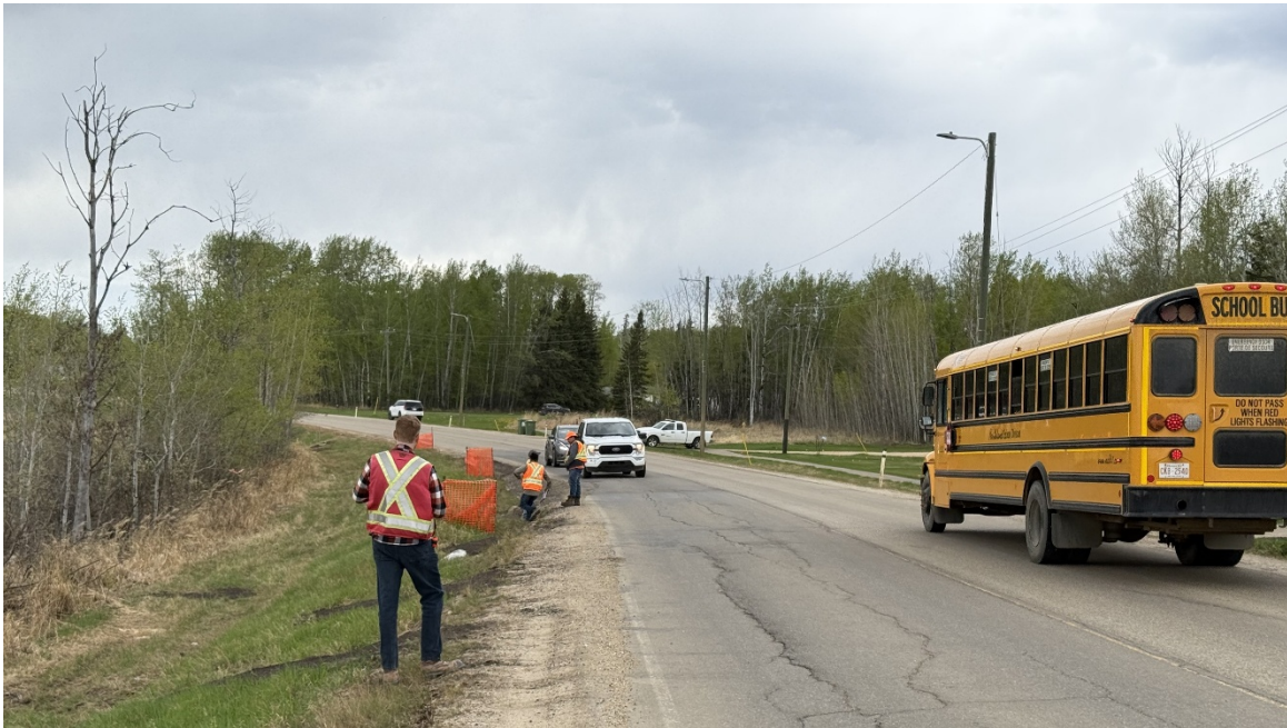
Photo 3. Longitudinal cracks (10-20 mm wide, 60 mm drop) within the previously patched area.
