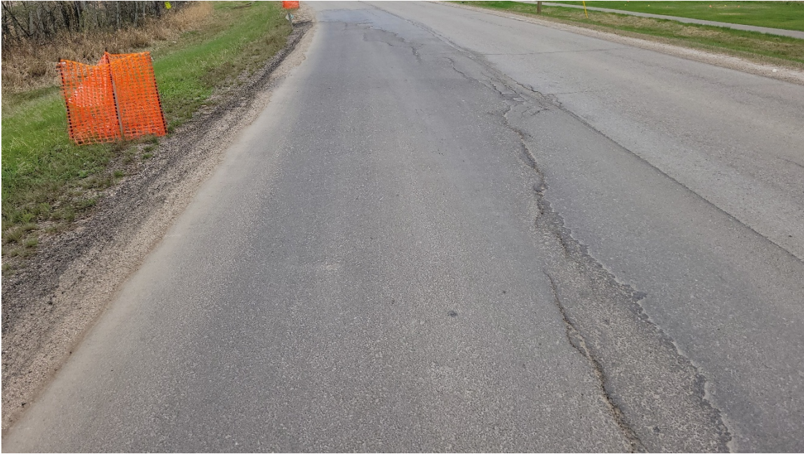
Photo 5. Looking north at the severely impacted section of the highway by the landslide movement. Area was patched after the 2024 inspection.
