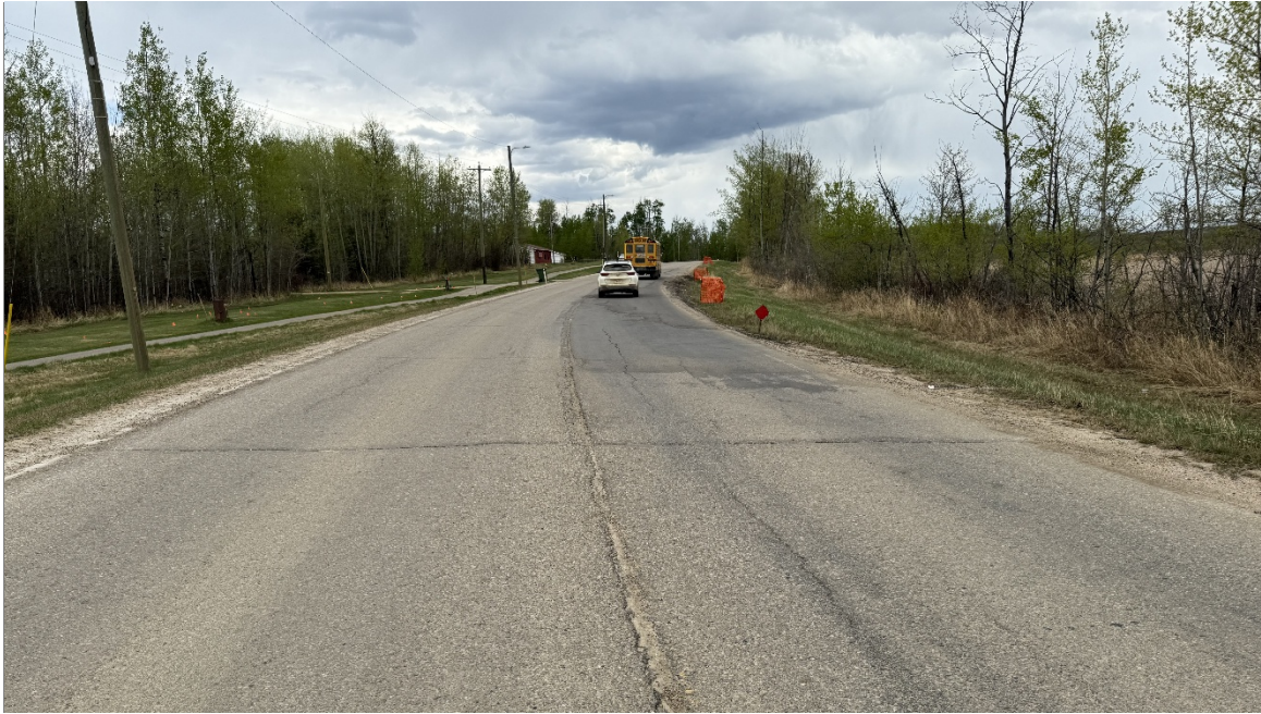
Photo 1. Northern flank of landslide. Head scarp open cracks were filled with ACP in early Spring 2024.
