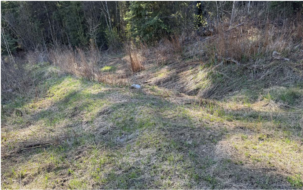
Photo 11. Ditch Runoff Berm – Well vegetated, no flow noted in 2025.
