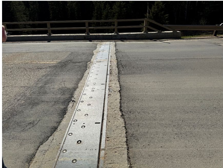
Photo 5. Looking at the north expansion joint. The area of distressed pavement area around the expansion joint has been patched since the 2024 inspection.
