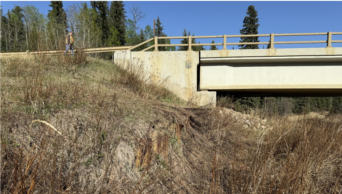
Photo 10. Northwest wingwall: soil staining on the wall face shows original design elevation of fill; approximately 1 m of gravel was placed in 2020 to buttress/cover the gap formed below the wing wall; vegetation has grown within the backfilled area since 2020; erosion up to 500 mm at the top developed within new fill placed against the wing wall (area with erosion had been filled with ACP).
