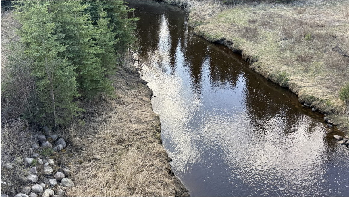
Photo 7. Toe of NW head slope and river channel.
