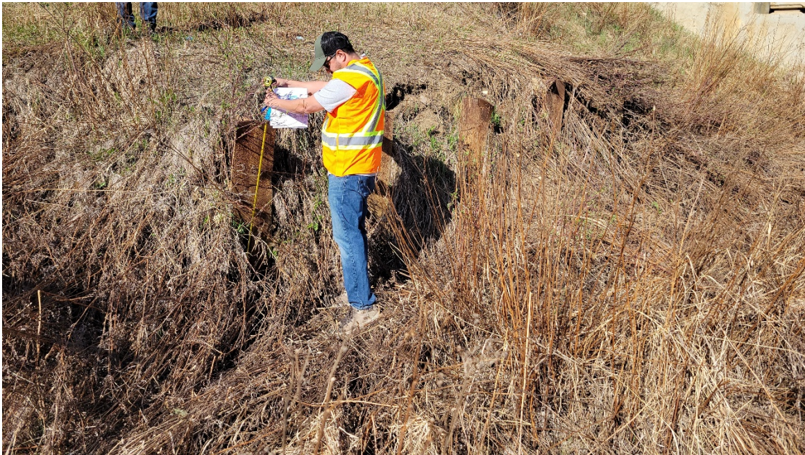
Photo 8. Exposed old bridge H piles within the active landslide mass. The landslide has a 1.8 m drop at this location.
