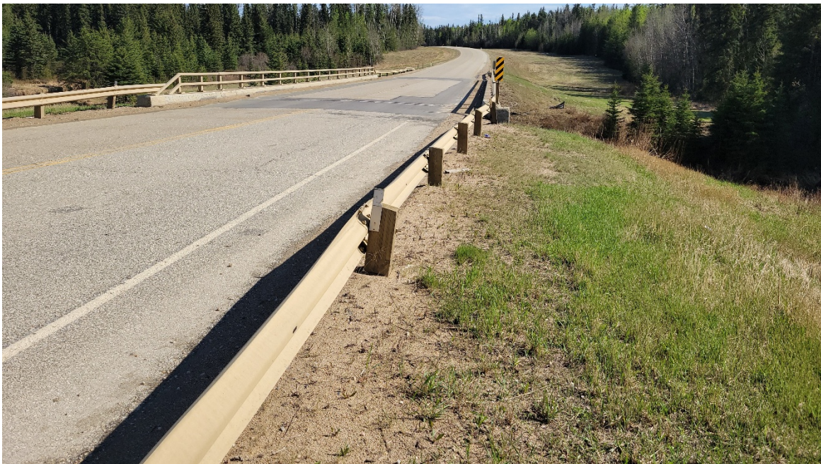
Photo 4. Bridge deck and highway surface condition (looking north at the south expansion joint). The previously distressed pavement area has been patched since the 2024 inspection.
