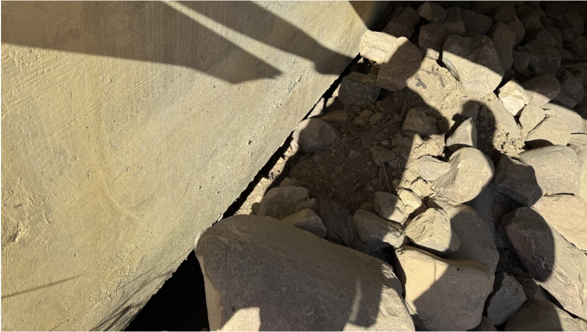
Photo 3. A closer look at the NW corner of the abutment seat. There is a 2.9 m long gap formed along the face of the abutment seat.
