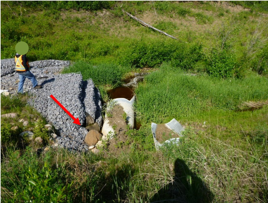
Photo 2 The 1500-mm and 900-mm culverts are being undermined by erosion around the east abutment and wing wall of the gabion wall drop structure (waypoint 482). Photo taken June 12, 2017 looking east.
