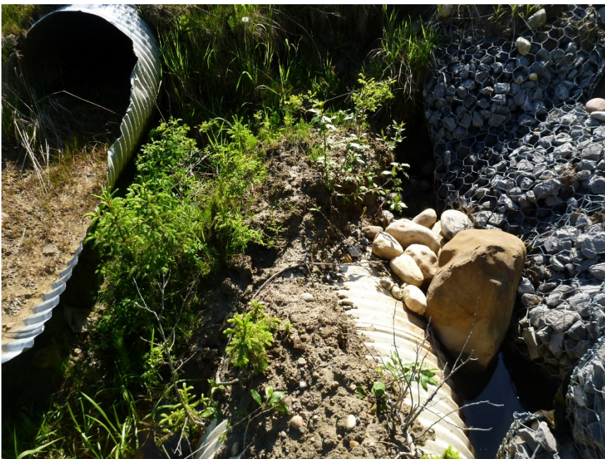
Photo 2 The 1500-mm and 900-mm culverts are being undermined by erosion around the east abutment and wing wall of the gabion wall drop structure (waypoint 482). Photo taken June 12, 2017 looking east.
