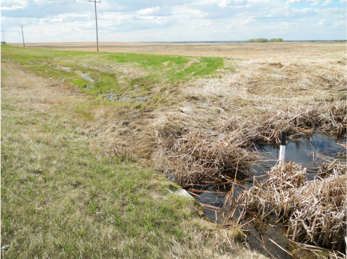
Ponded water north of highway
