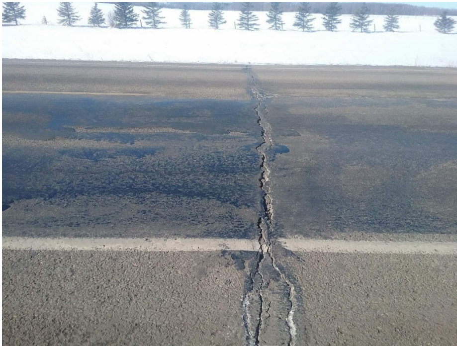
Photo 6 Patched area (3 of 3) at heaved location. Photo taken February 28, 2018 looking north-west.
