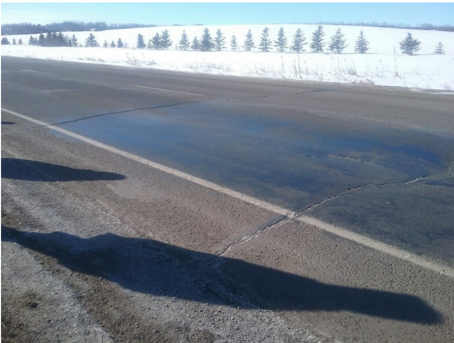
Photo 2 Patched area (1 of 3) at heaved location on northbound lane bounded by transverse cracks (about 7 m apart). Photo taken February 28, 2018 looking south-west.
