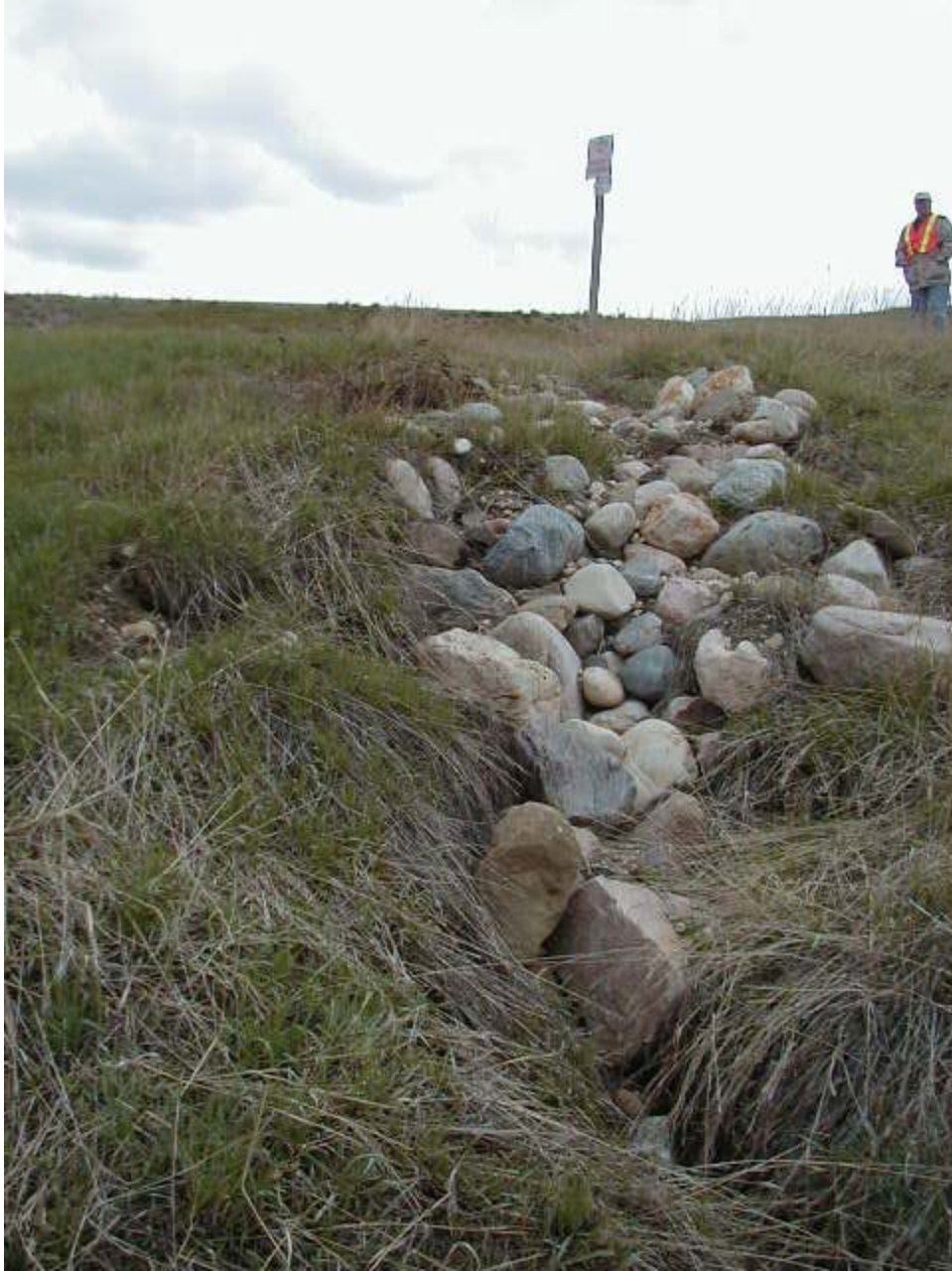
Riprap channel north of fenceline
