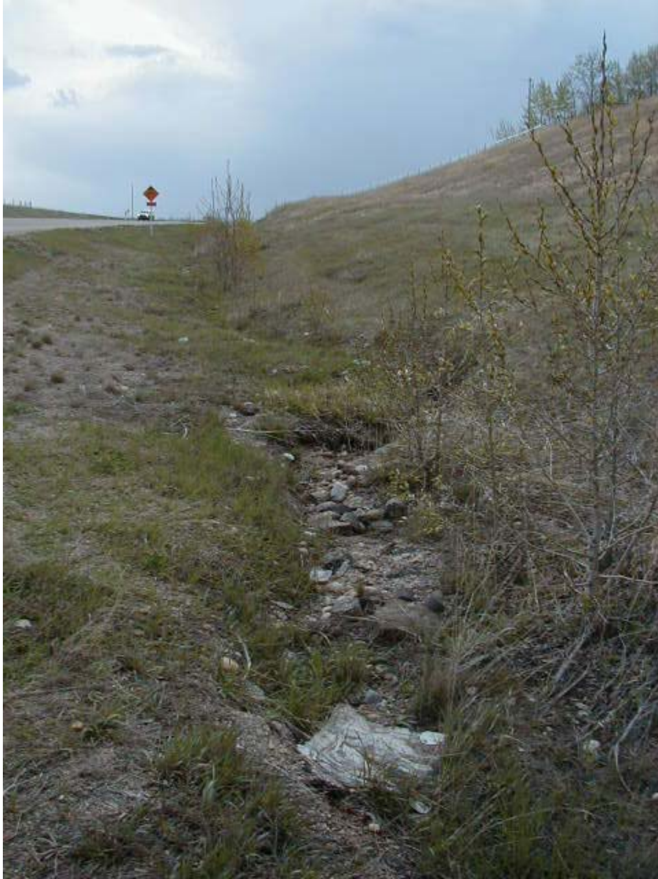
Looking east along south ditch
