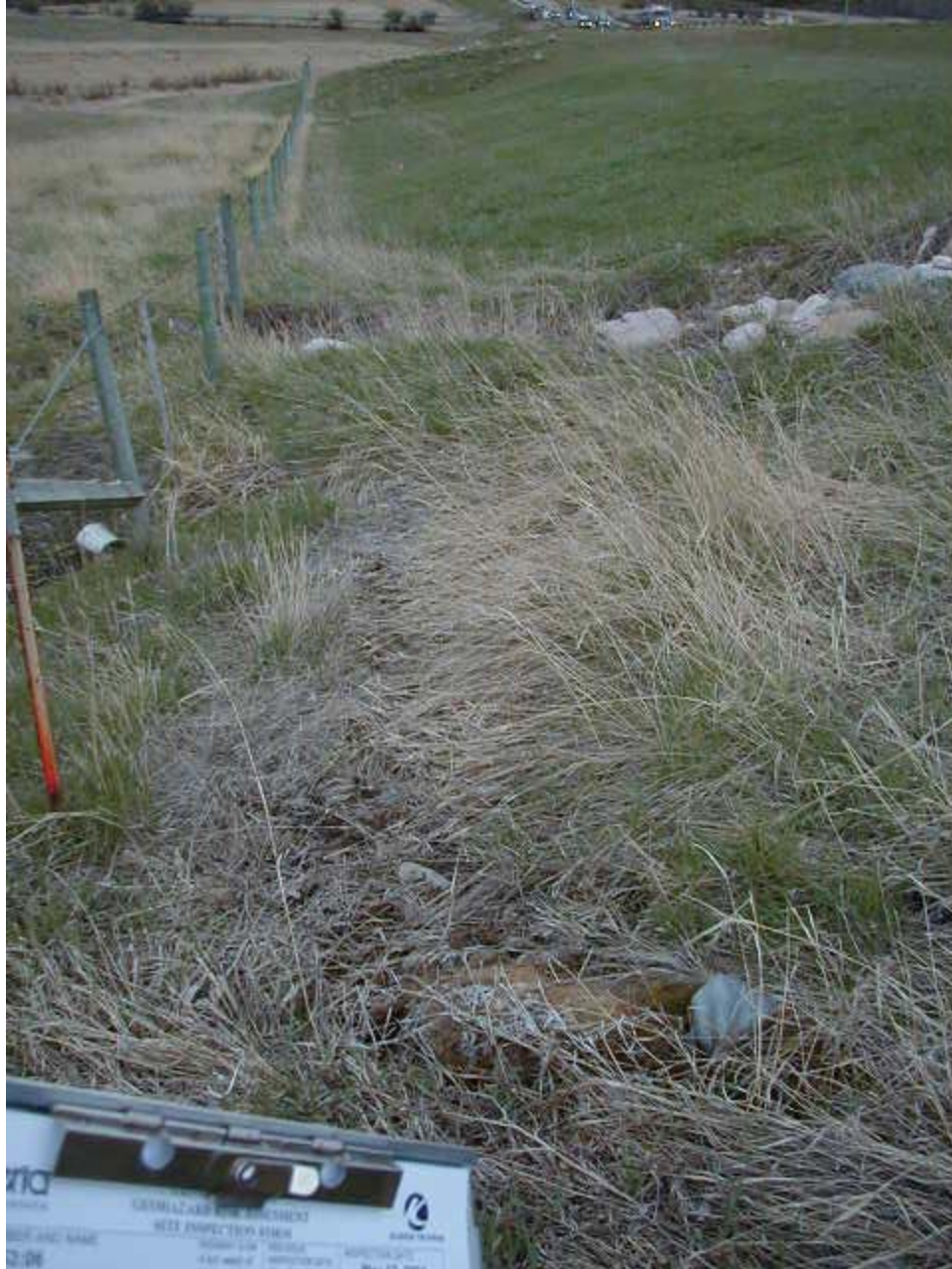
Looking west at end of riprap channel and exposed drain outlet north of fenceline
