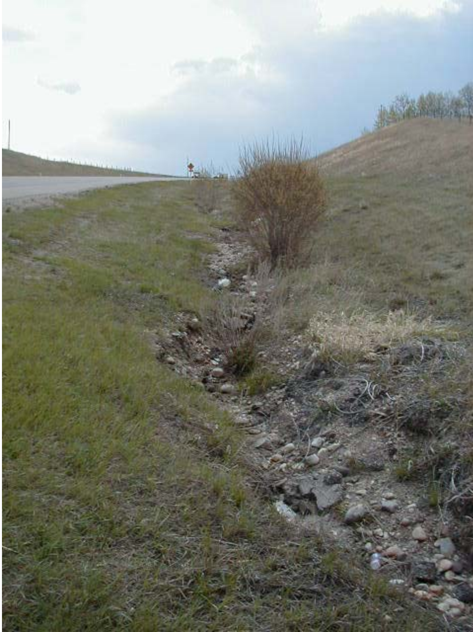
Looking east along south ditch
