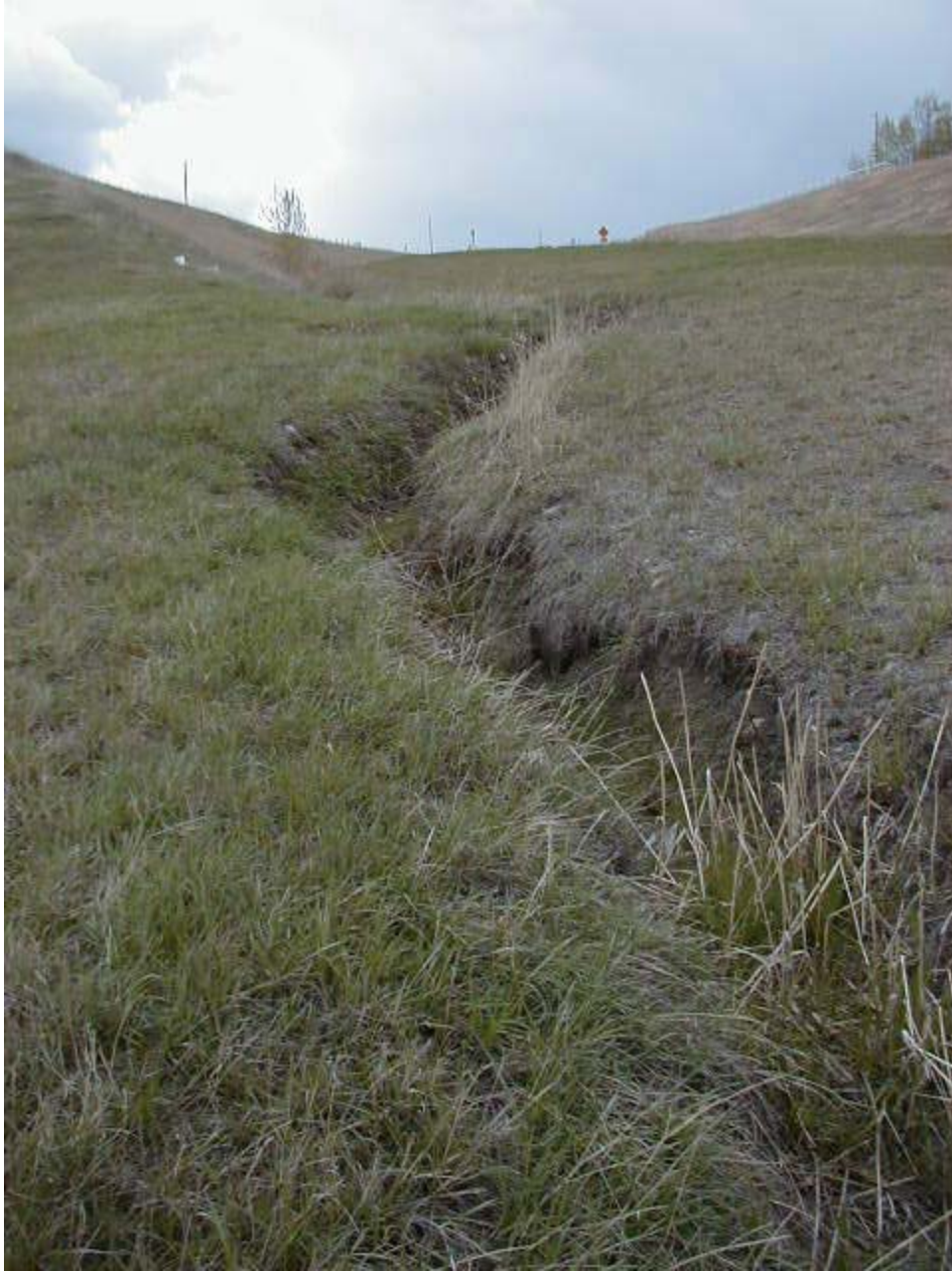
Looking east at west end of north ditch.
