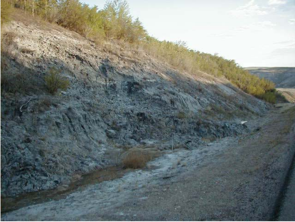
Spring area and slumped material in ditch
