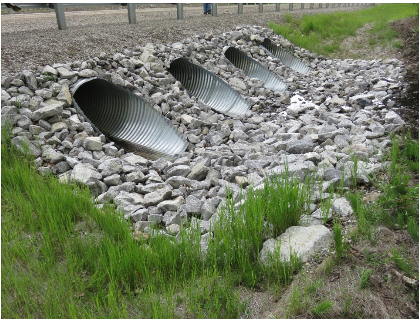
Photo 2 The inlets of the four 1000-mm culverts that were installed in June 2016. Vegetation is growing through the erosion control cloth that was placed around the culverts and in the ditch in June 2016. Photo taken June 12, 2017 looking southwest.
