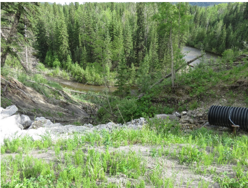
Photo 6 The erosion gully and slide area located on the north slope of the James River Valley, downstream of the drain outfall. The site is the original C030 site that the high-water-mitigation drainage works were designed to divert water away from. Photo taken June 12, 2017 looking southeast.
