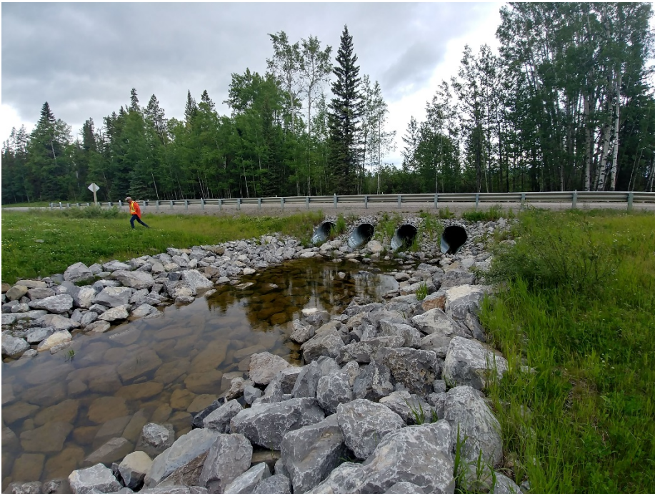
Photo 4 Photo showing the culvert outlets and riprap armoured stilling basin on south side of highway. Photo taken July 9, 2019 looking northwest.
