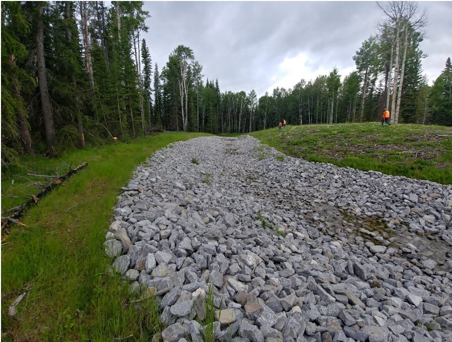
Photo 6 Photo showing the location where water is discharging over the river valley slope from the armoured outlet channel (waypoint 879). Photo taken July 9, 2019.
