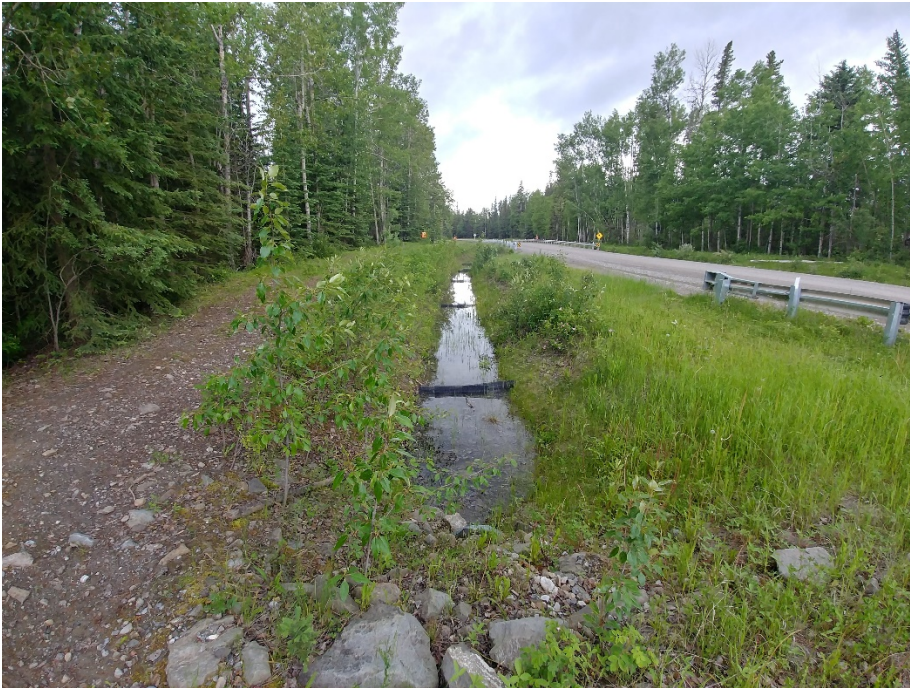
Photo 4 Photo showing the culvert outlets and riprap armoured stilling basin on south side of highway. Photo taken July 9, 2019 looking northwest.
