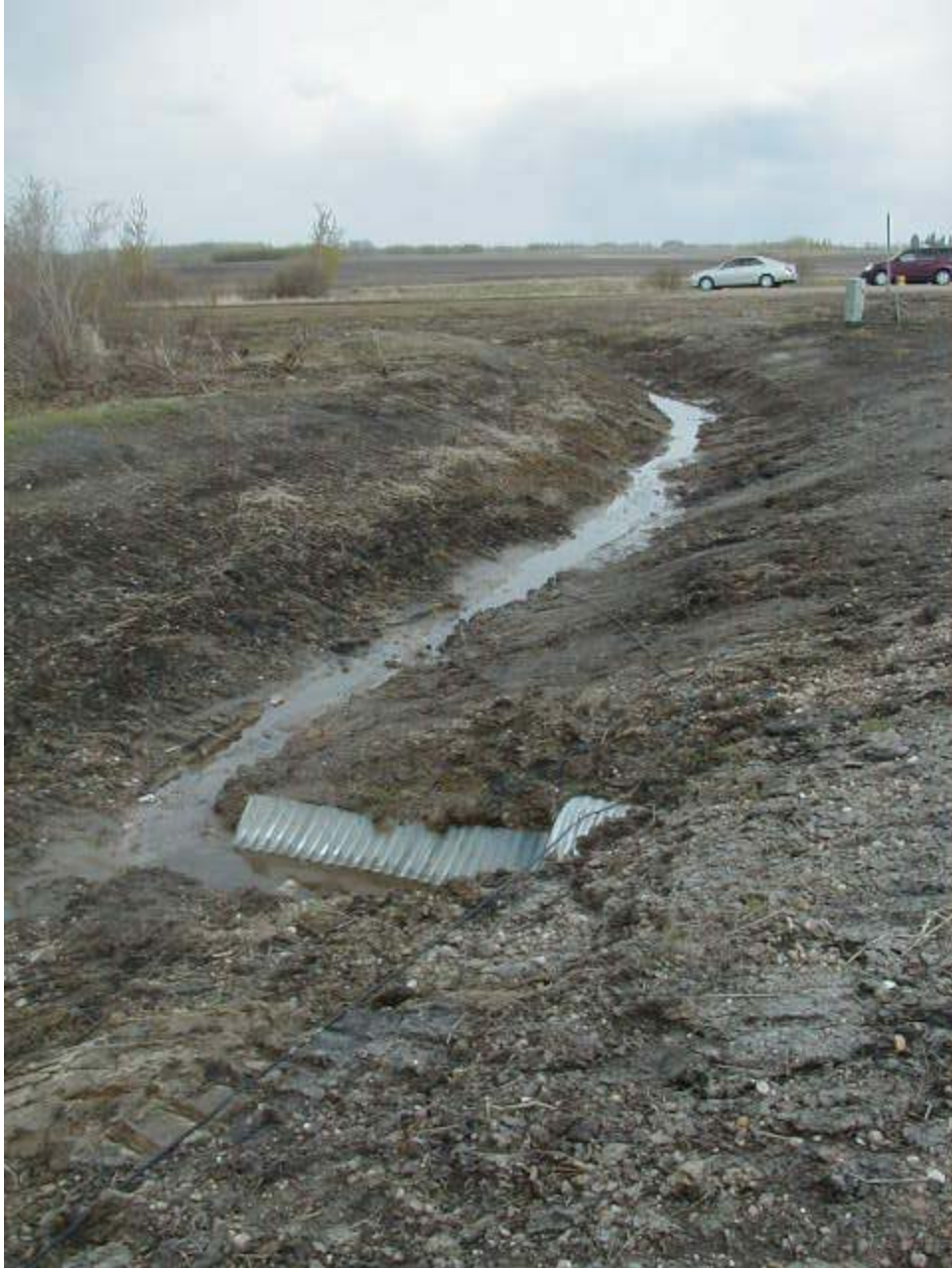
Looking north at culvert outlet in west ditch.
