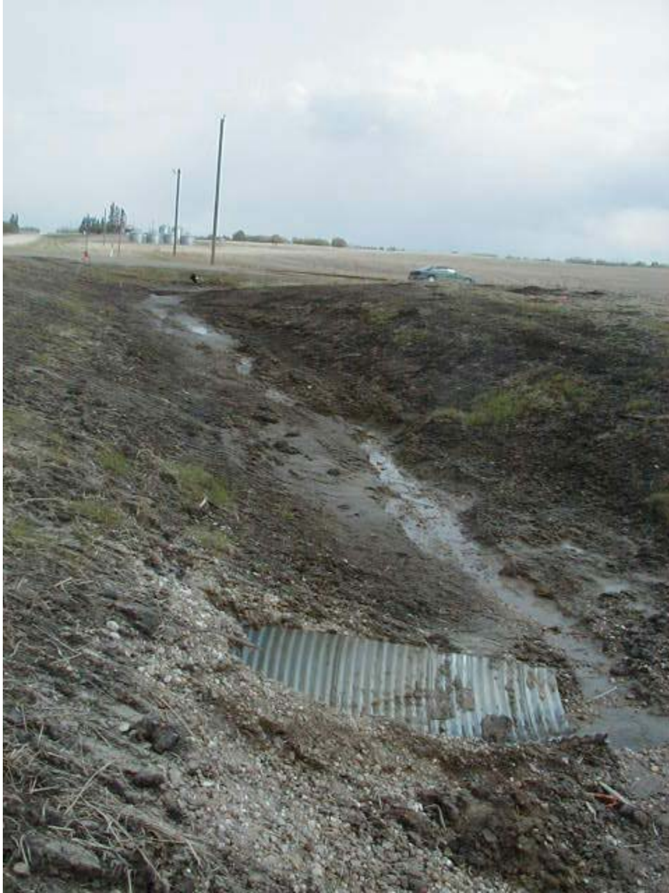
East ditch looking north over new culvert inlet.
