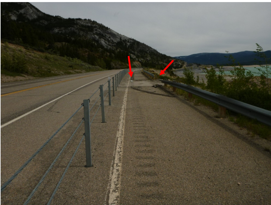
Photo 2 Photo showing the section of asphalt curb and guardrail removed (approx. 5m) during placement of gravel backfill in the western most erosion gully (way. Photo taken June 11, 2018 looking northeast.
