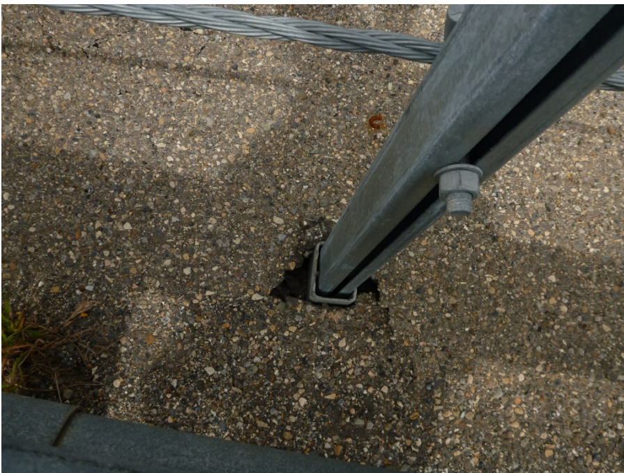
Photo 6 Asphalt collapse due to erosion at the base of one of the high-tension cable barrier (HTCB) posts near western extent of the barrier. Photo taken June 12, 2017 looking north.
