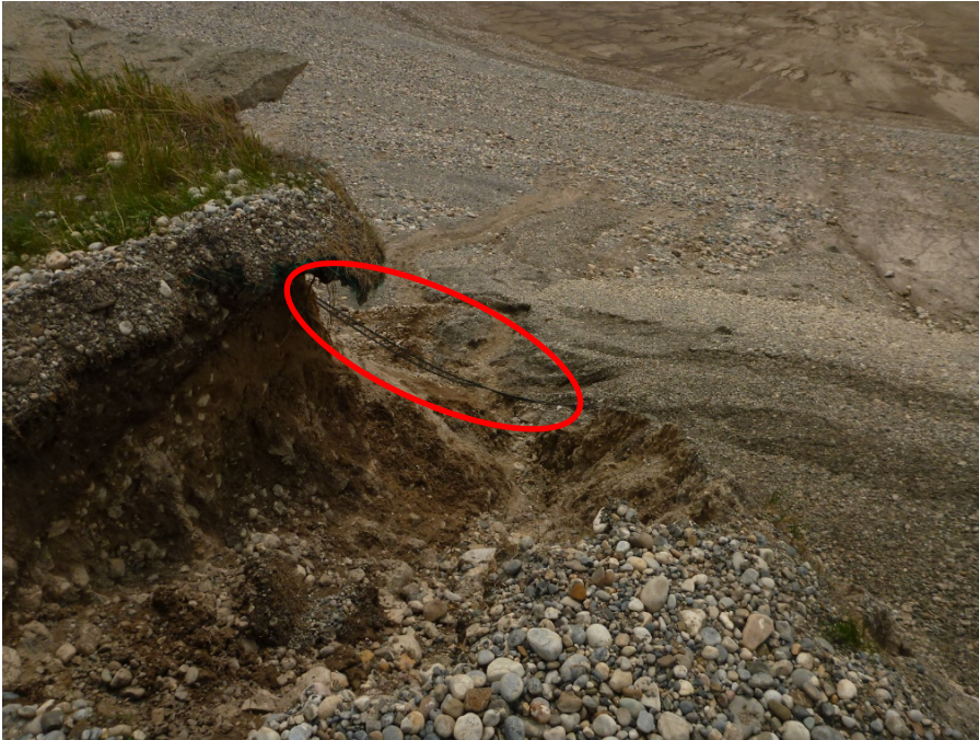
Photo 6 Asphalt collapse due to erosion at the base of one of the high-tension cable barrier (HTCB) posts near western extent of the barrier. Photo taken June 12, 2017 looking north.
