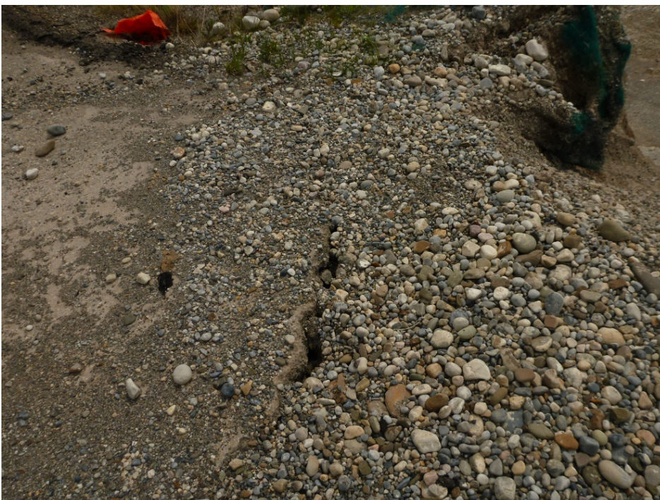
Photo 4 Tension cracks observed in the gravel fill at the crest of the embankment. Photo taken June 11, 2018 looking northeast.
