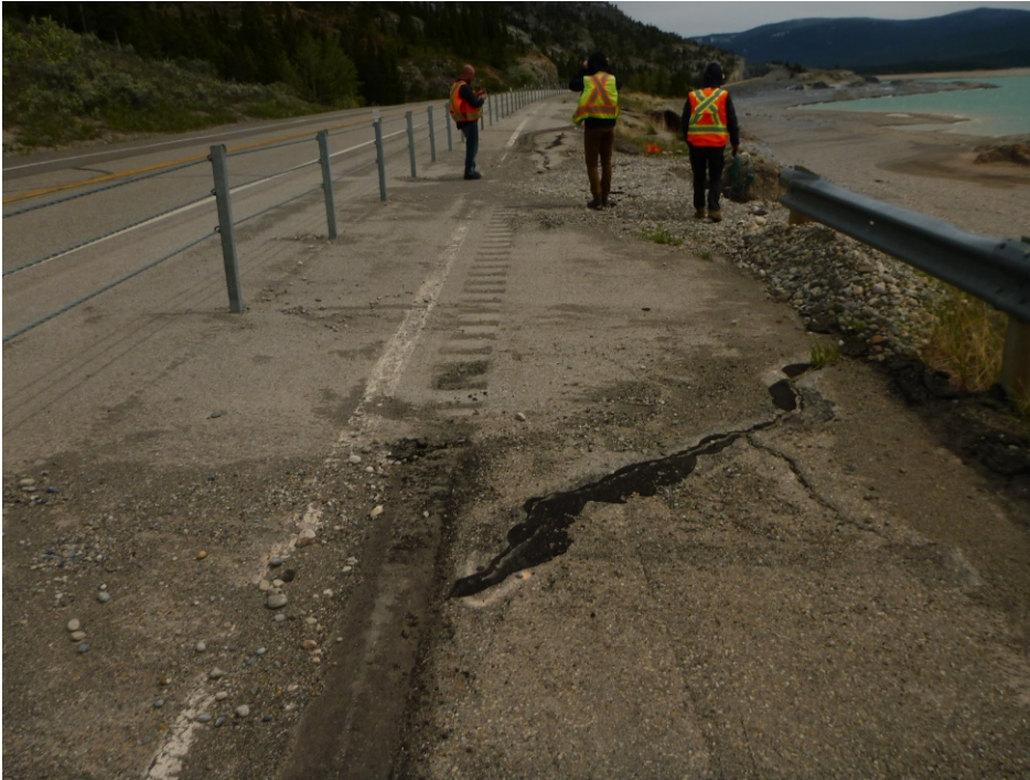
Photo 4 Tension cracks observed in the gravel fill at the crest of the embankment. Photo taken June 11, 2018 looking northeast.
