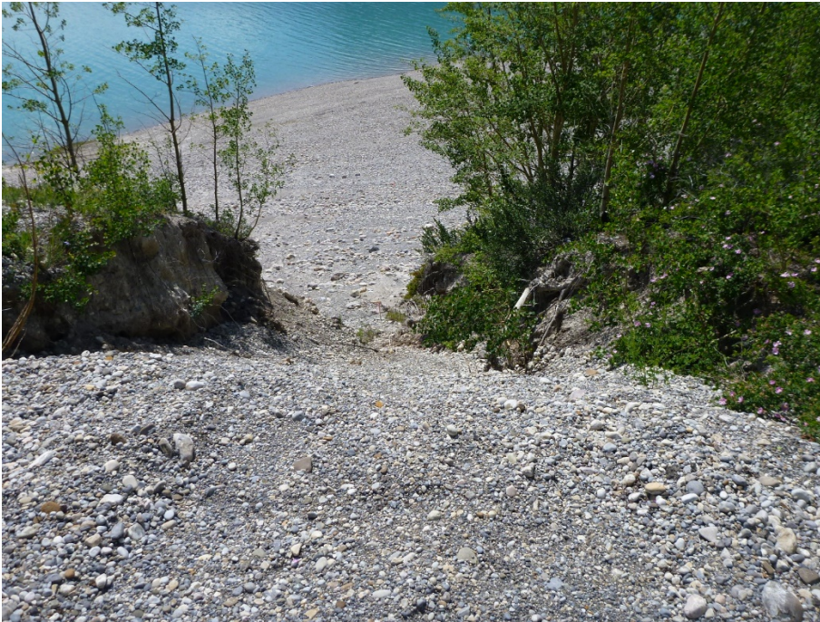
Photo 6 Photo showing the extent of temporary rock-fill berm constructed at the toe of the eroding slope. Berm was constructed by PME as part of the 2019 Temporary Works at the C034 site. Photo taken July 23, 2019 looking north.
