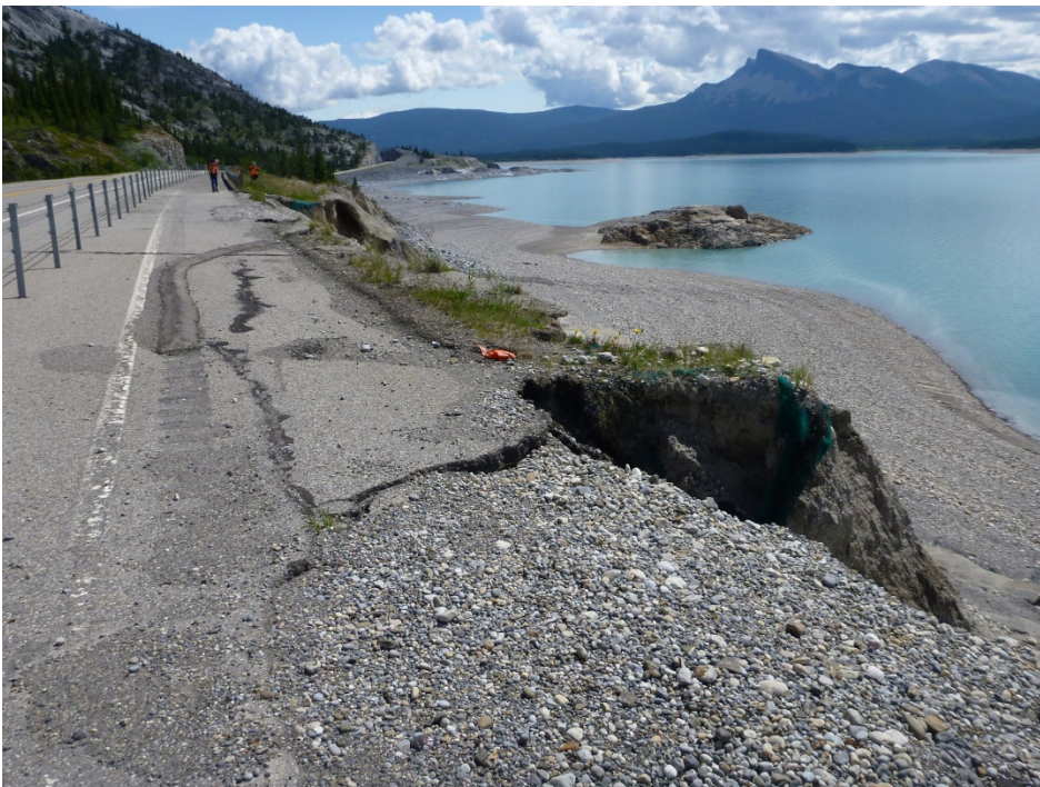
Photo 4 Photo showing the condition of the pavement above the main erosion gullies. Pavement cracks have extended to the white line marking the edge of the old eastbound lane. Photo taken July 9, 2019 looking northeast.
