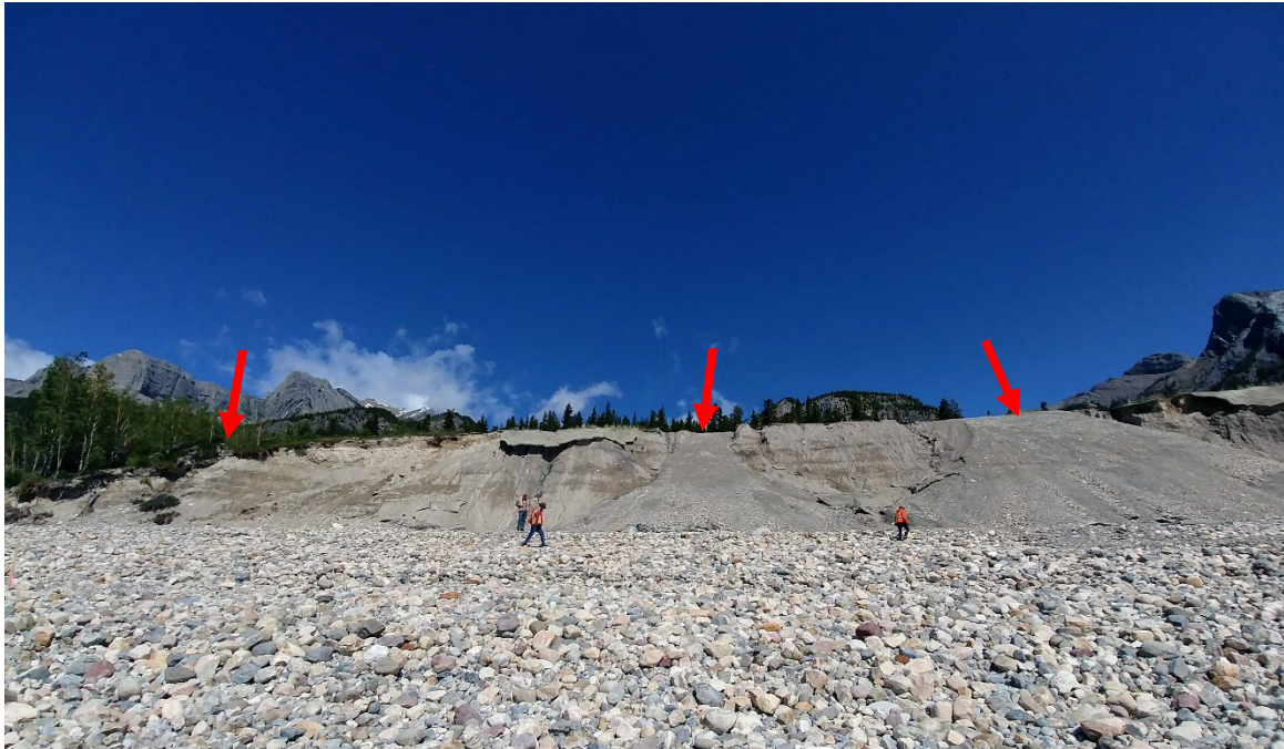
Photo 2 Shotcrete debris and steel mesh accumulating at the toe of the slope. Photo taken July 9, 2019 looking north.
