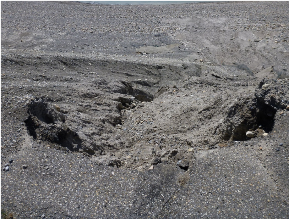
Photo 4 Photo showing the condition of the pavement above the main erosion gullies. Pavement cracks have extended to the white line marking the edge of the old eastbound lane. Photo taken July 9, 2019 looking northeast.
