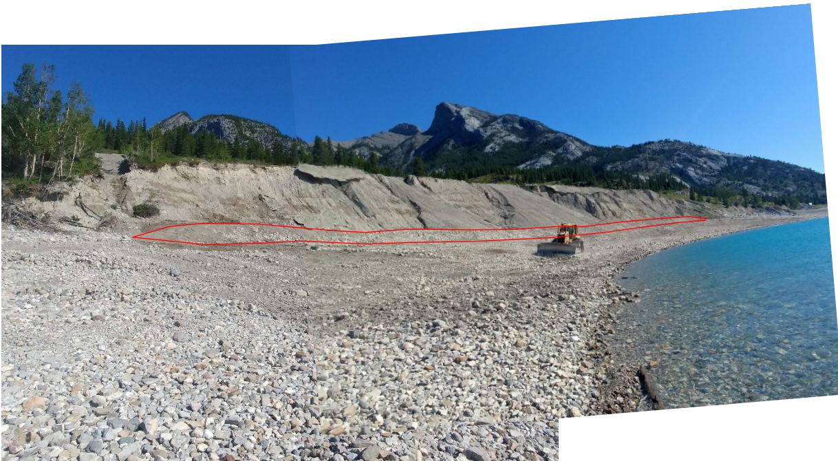
Photo 6 Photo showing the extent of temporary rock-fill berm constructed at the toe of the eroding slope. Berm was constructed by PME as part of the 2019 Temporary Works at the C034 site. Photo taken July 23, 2019 looking north.
