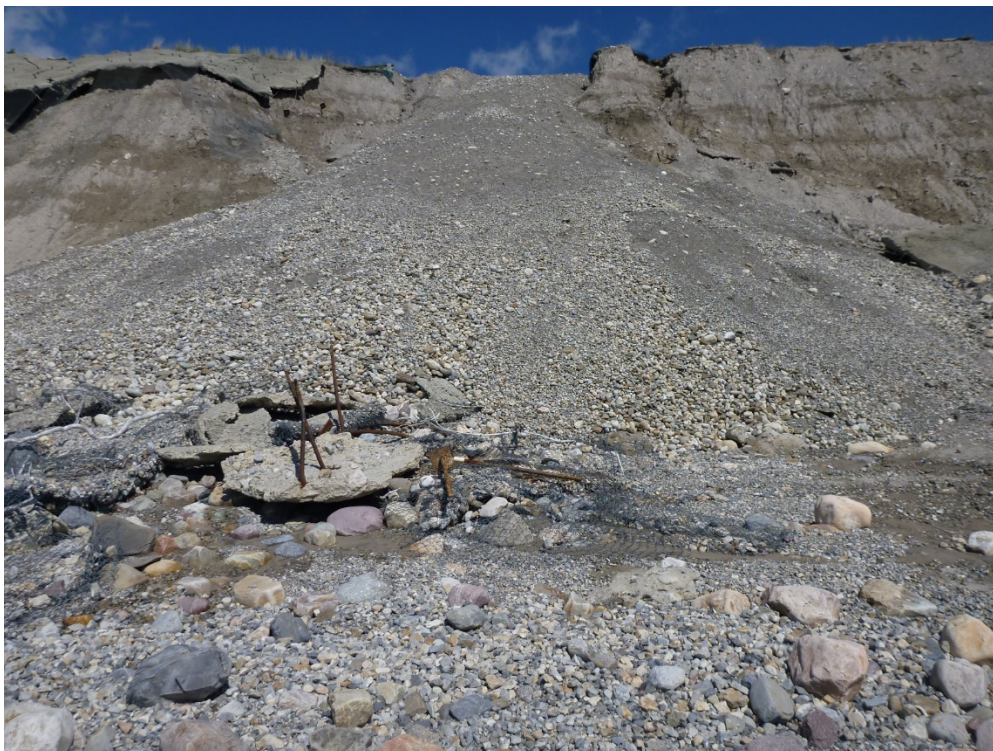
Photo 2 Shotcrete debris and steel mesh accumulating at the toe of the slope. Photo taken July 9, 2019 looking north.
