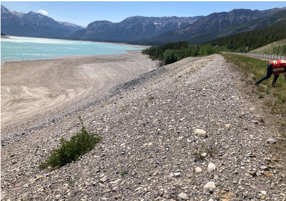
Photo 2 The repaired slope along C034-1 appears to be in good condition and is performing well. Photo taken June 9, 2025 facing west.
