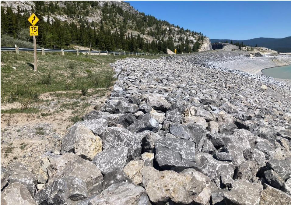
Photo 6 Boulders (indicated by red arrows) placed near the break in the guardrail in an attempt to reduce traffic along the crest of the C034-2 repair. Photo taken June 9, 2025 facing northwest.
