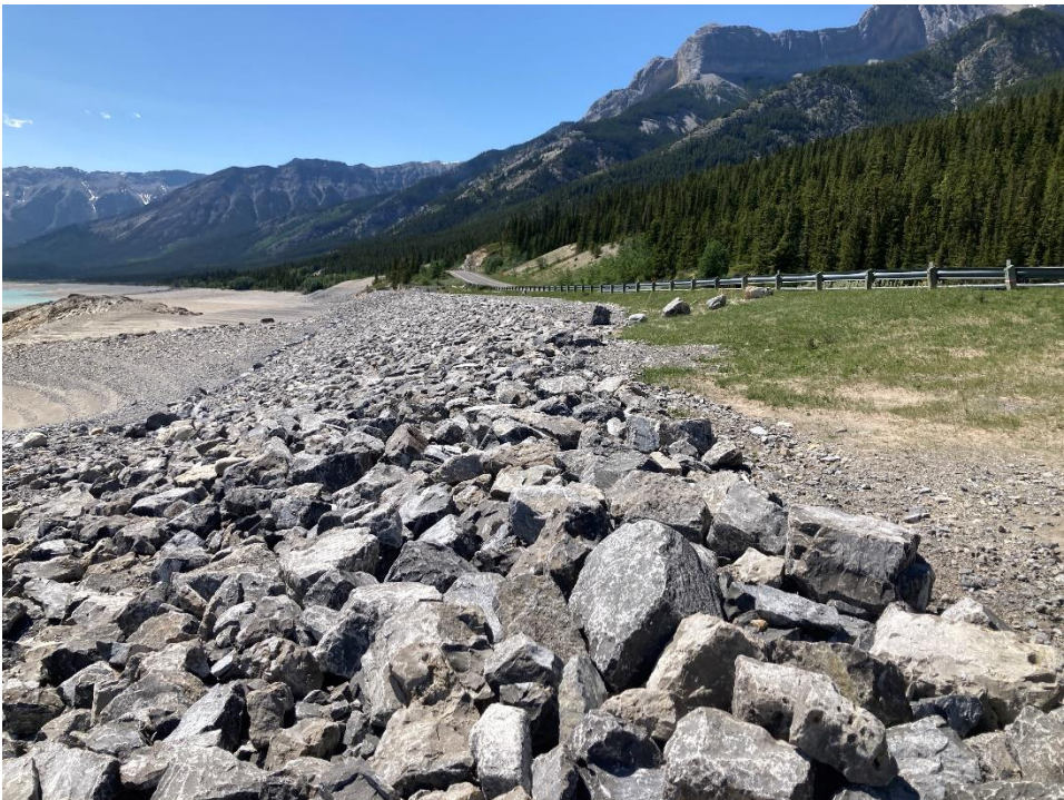
Photo 4 The repaired slope along C034-2 appears to be in good condition and is performing well. Photo taken June 9, 2025 facing west.
