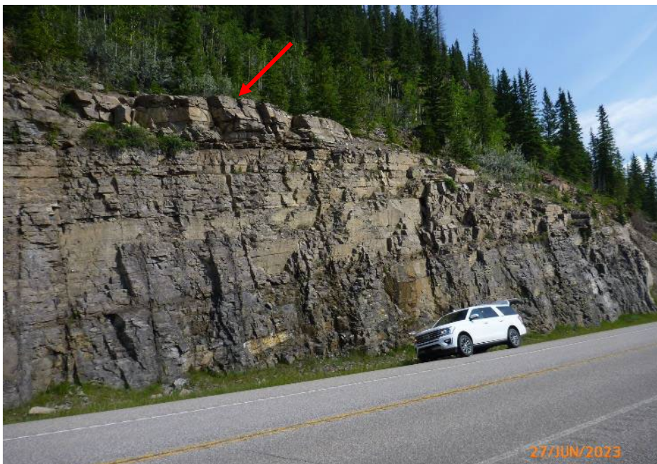
Photo 6 The relatively intact rock slope along the middle and west portion of the site. There is a potentially unstable shelf of rock at the top of the rock slope (indicated by red arrow). Photo taken June 27, 2023, facing north-northeast.
