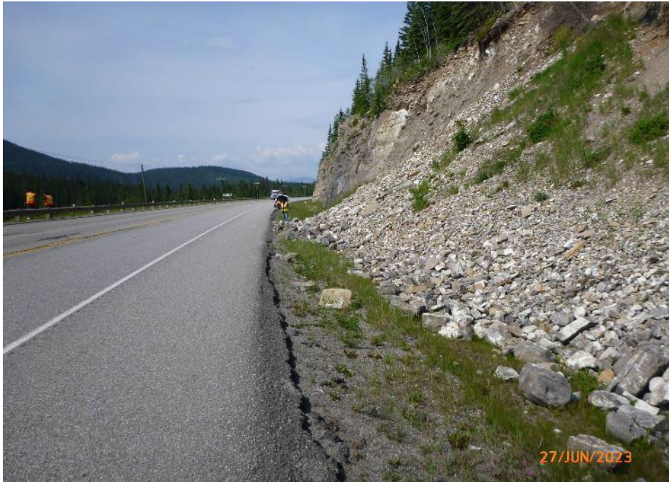
Photo 4 Overburden overhanging the crest of the slope near the east extent of the site. Photo taken June 27, 2023, facing north.
