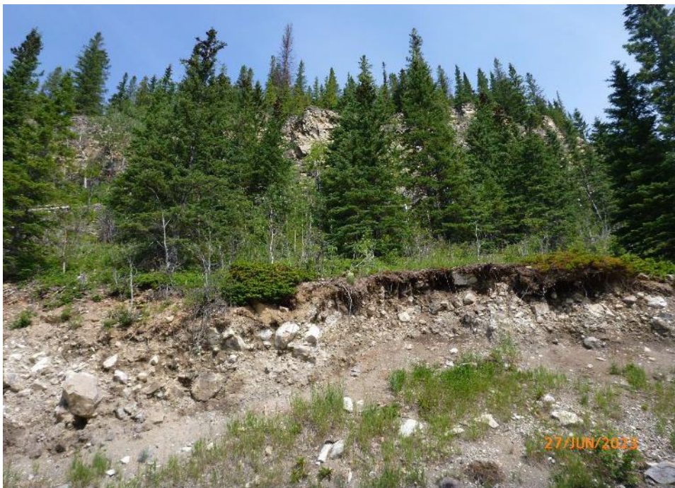
Photo 4 Overburden overhanging the crest of the slope near the east extent of the site. Photo taken June 27, 2023, facing north.
