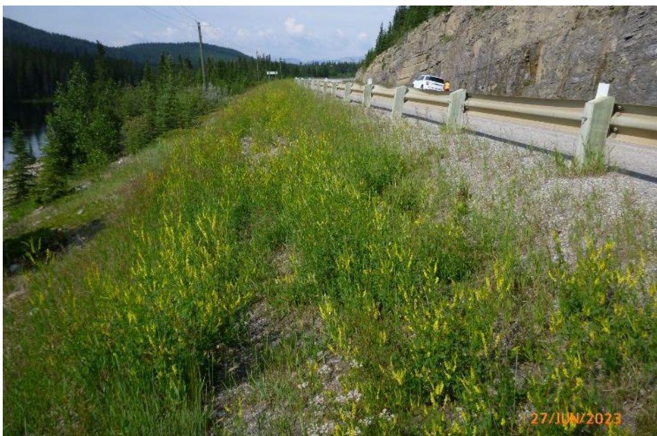
Photo 8 The south (eastbound) highway embankment slope is relatively well vegetated and appears to be in good condition. No rockfall particles were observed on the south side of the highway during the 2023 inspection. Photo taken June 27, 2023, facing west.
