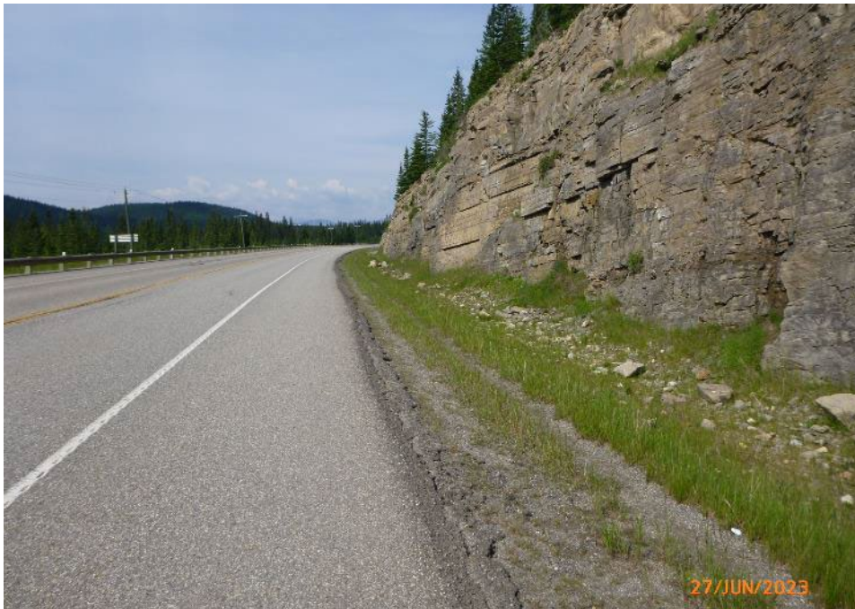
Photo 8 The south (eastbound) highway embankment slope is relatively well vegetated and appears to be in good condition. No rockfall particles were observed on the south side of the highway during the 2023 inspection. Photo taken June 27, 2023, facing west.
