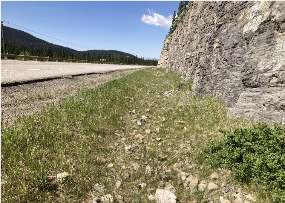
Photo 6 Larger rockfalls up to approximately 1 m long in the north (westbound) ditch at the west extent of the site were deposited between the 2023 and 2025 inspections. Photo taken June 9, 2025 facing east.
