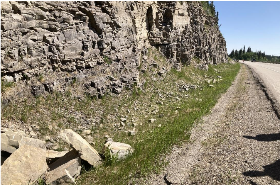
Photo 6 Larger rockfalls up to approximately 1 m long in the north (westbound) ditch at the west extent of the site were deposited between the 2023 and 2025 inspections. Photo taken June 9, 2025 facing east.
