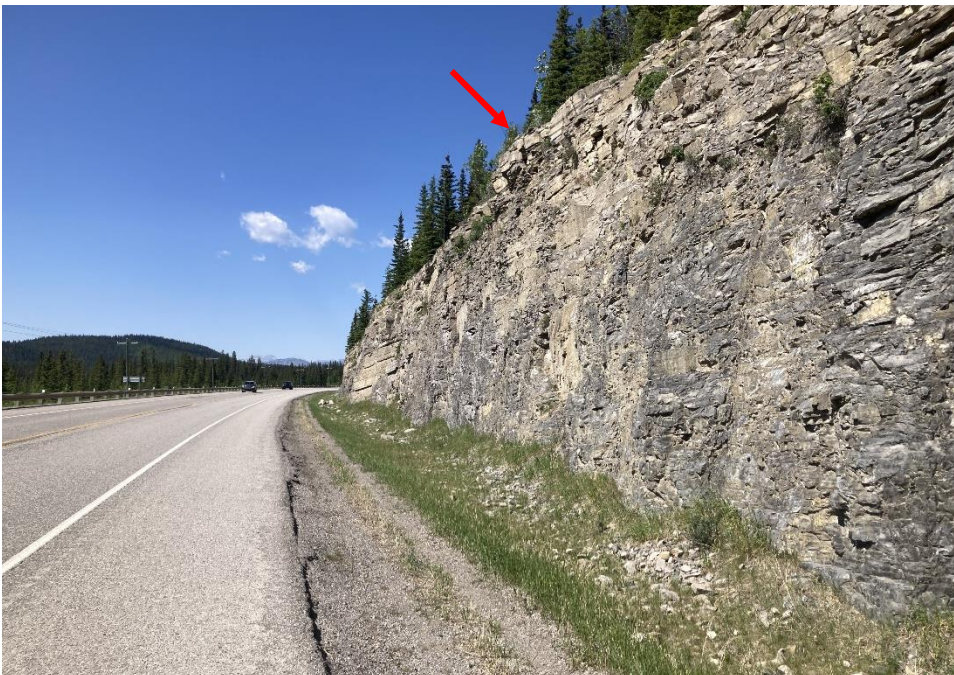
Photo 4 The relatively intact rock slope along the west portion of the site. There is a potentially unstable shelf of rock at the top of the rock slope (indicated by red arrow). Photo taken June 9, 2025 facing west-northwest.
