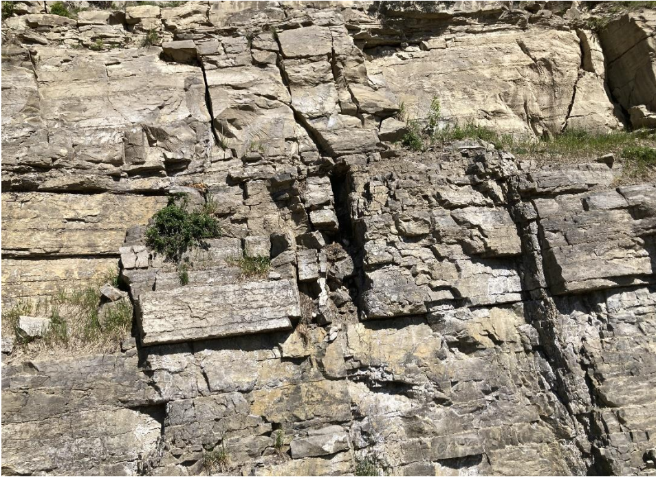
Photo 4 The relatively intact rock slope along the west portion of the site. There is a potentially unstable shelf of rock at the top of the rock slope (indicated by red arrow). Photo taken June 9, 2025 facing west-northwest.
