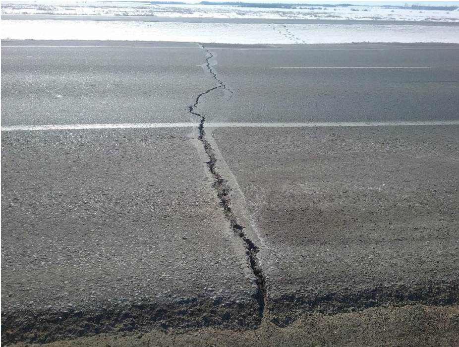
Photo 2 Transverse pavement cracking and depression along westbound lane (east section). Photo taken February 28, 2018 looking south.
