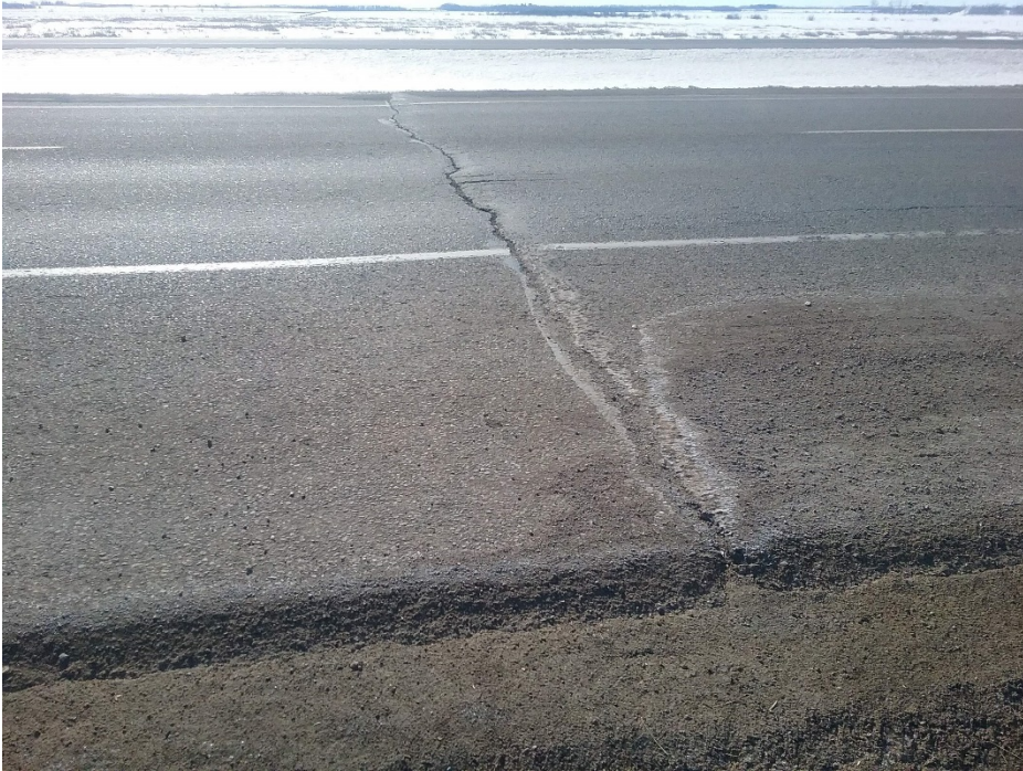
Photo 2 Transverse pavement cracking and depression along westbound lane (east section). Photo taken February 28, 2018 looking south.
