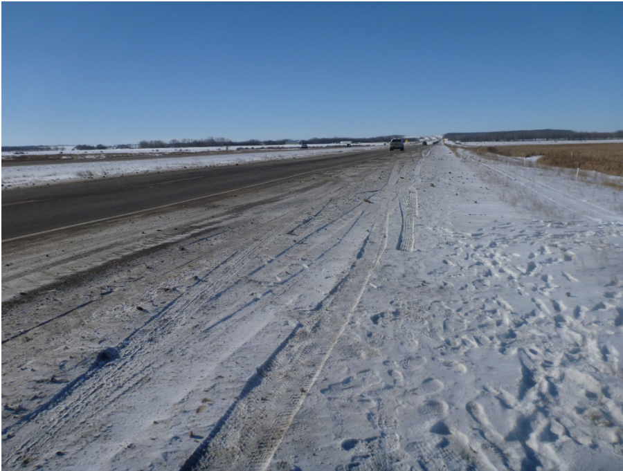
Photo 1 Location of frost heave site (east section). Photo shows the rolling pavement condition. Photo taken on February 21, 2018 looking west.
