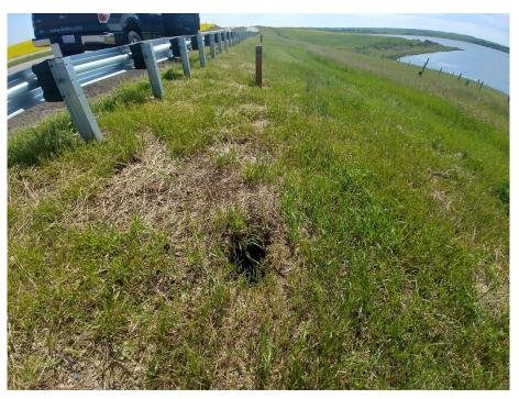
Photo 4 Cracking along south shoulder of east bound lanes, east of H-pile wall. Photo taken July 12, 2019 looking west.
