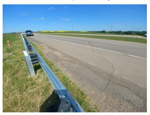
Photo 2 Photo showing settlement and expansion of pavement cracks. Photo taken July 12, 2019.
