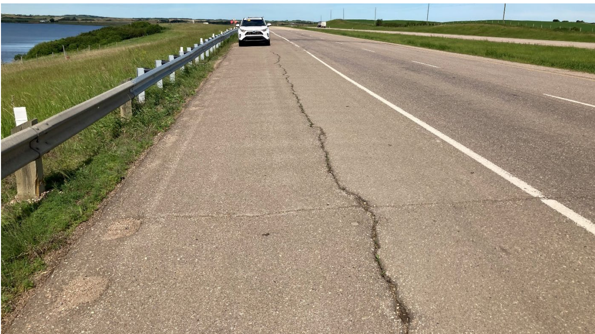
Photo 4 Asphalt cracking in the shoulder of the eastbound lane, east of the existing H-pile wall. Photo taken June 24, 2020 facing west.
