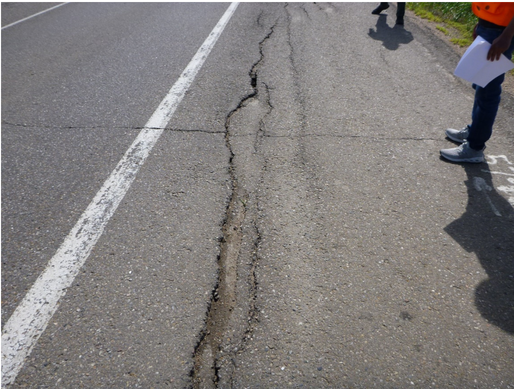
Photo 2 Asphalt cracking and settlement area observed in the eastbound lane. Photo taken June 22, 2020 facing west.
