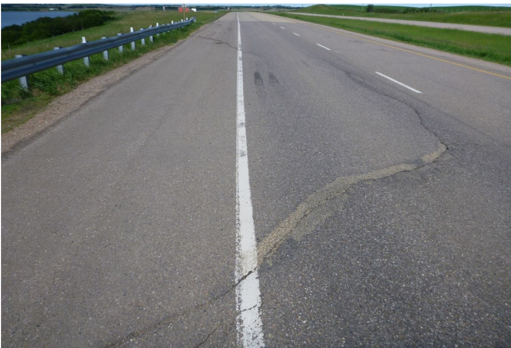
Photo 2 Asphalt cracking and settlement area observed in the eastbound lane. Photo taken June 22, 2020 facing west.
