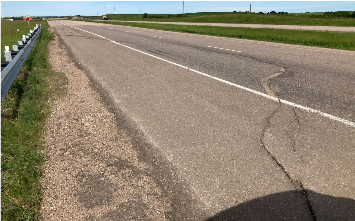
Photo 4 Asphalt cracking in the shoulder of the eastbound lane, east of the existing H-pile wall. Photo taken June 24, 2020 facing west.
