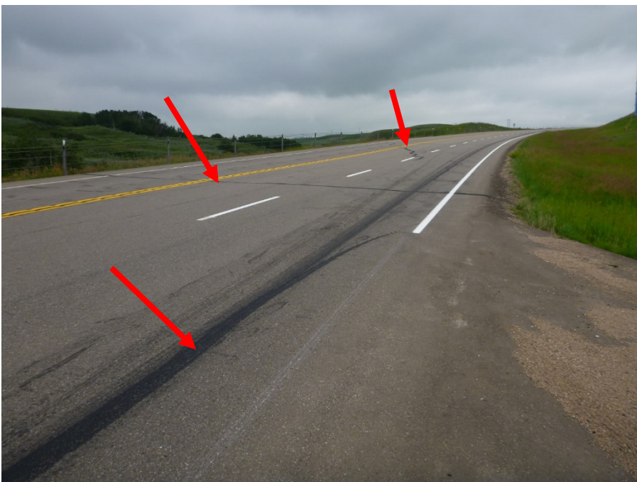
Photo 2 View of pavement surface north at C067 Site B. Sealed pavement cracks (red arrows) do not appear to have gotten worse since 2018. Photo taken July 11, 2019 looking northwest.
