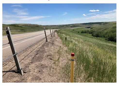
Photo 2 Two voids were observed on the west (southbound) shoulder of Hwy 21. KCB and AT believe they were caused by removing guardrail posts during construction. Photo taken June 23, 2021.
