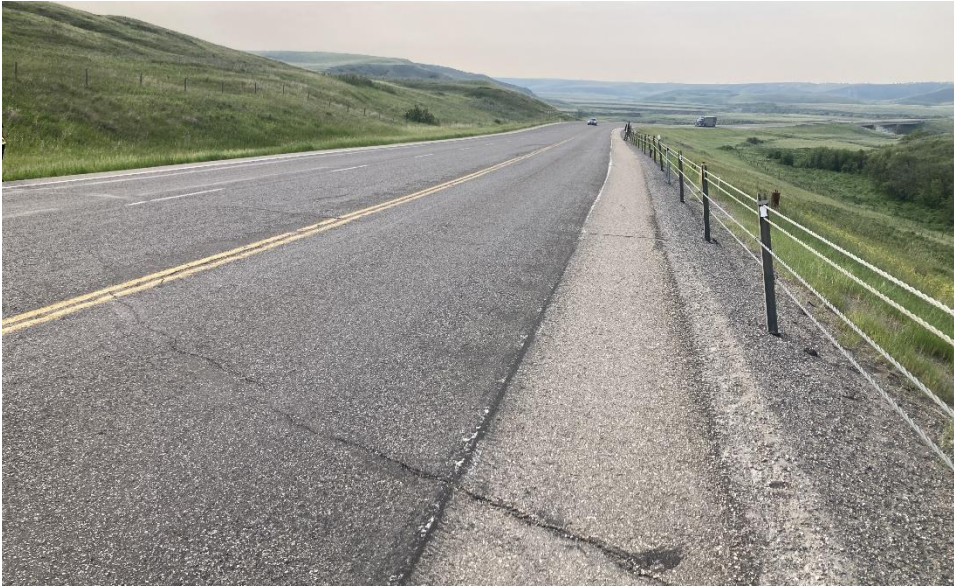
Photo 8 Pavement along Site B was resurfaced (chip sealing) in summer 2024, generally obscuring pavement distress (settlement and cracking) observed during previous inspections. Photo taken June 10, 2025 facing northwest.
