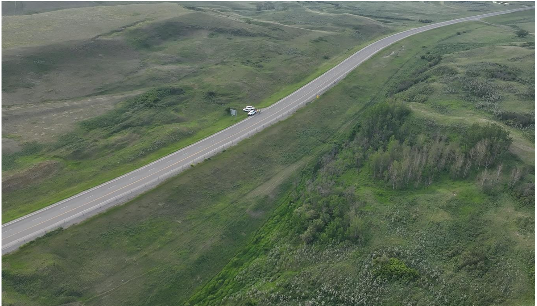
Photo 6 Aerial photo of C067 Site B located downslope (southeast) of Site A. The highway embankment slope is well vegetated and generally even, indicating the H-pile wall is performing well. Photo taken June 10, 2025 facing east.
