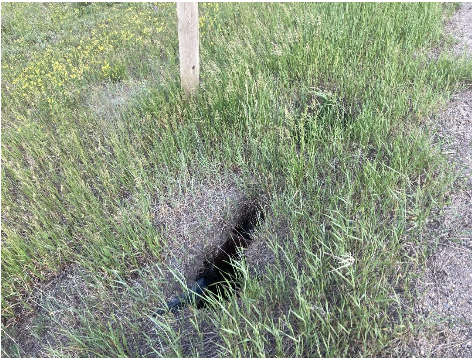
Photo 10 Voids are located along the Site B above the 2017 H-pile wall. Photo taken June 10, 2025 facing west.
