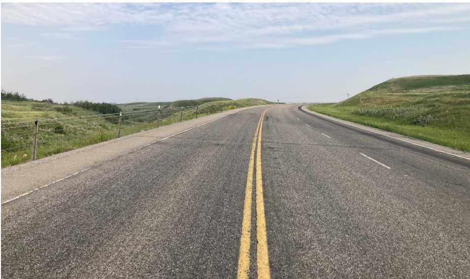
Photo 8 Pavement along Site B was resurfaced (chip sealing) in summer 2024, generally obscuring pavement distress (settlement and cracking) observed during previous inspections. Photo taken June 10, 2025 facing northwest.
