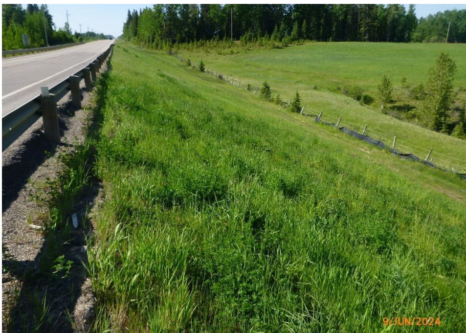
Photo 4 The repair of the highway embankment slope is well vegetated and appears to be performing well. Photo taken June 9, 2025 facing south-southwest.
