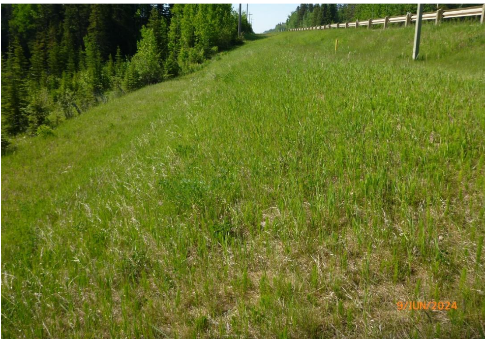
Photo 8 East highway embankment slope above culvert inlet is well vegetated and appears to be performing satisfactorily. Minor evidence of movement (ground cracks) observed near the embankment toe. Photo taken June 9, 2025 facing south.
