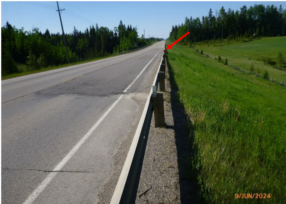
Photo 4 The repair of the highway embankment slope is well vegetated and appears to be performing well. Photo taken June 9, 2025 facing south-southwest.
