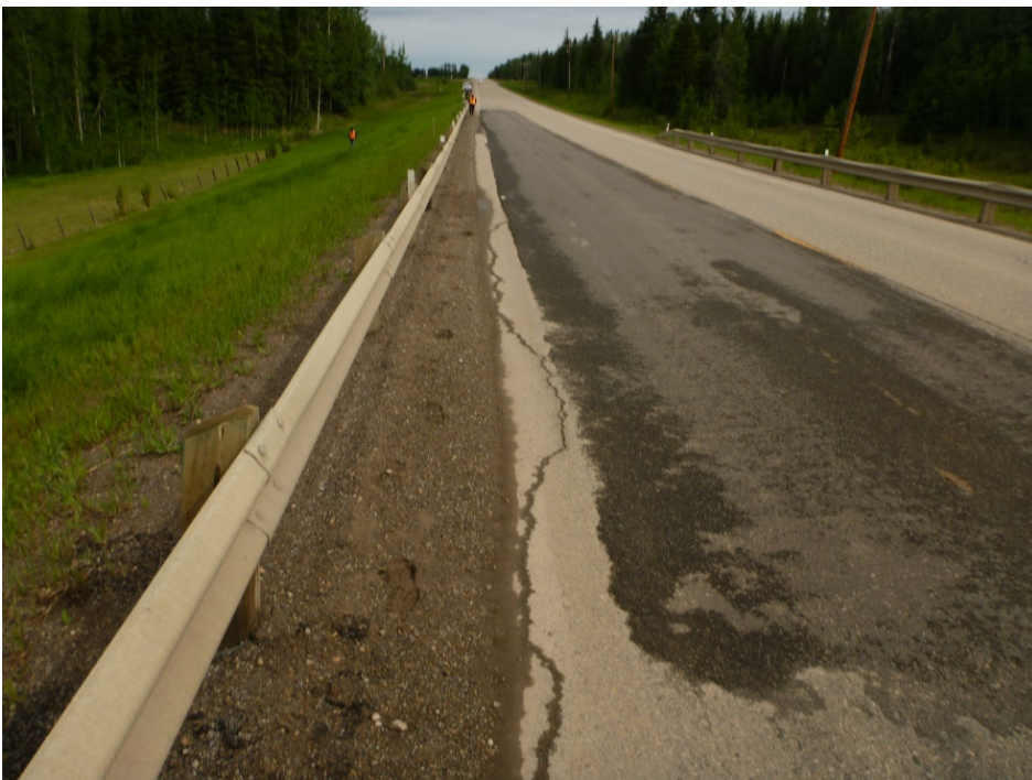
Photo 2 New pavement cracking (approximately 8 m in length) at the south end of the asphalt patch. Photo taken June 11, 2018 looking north.
