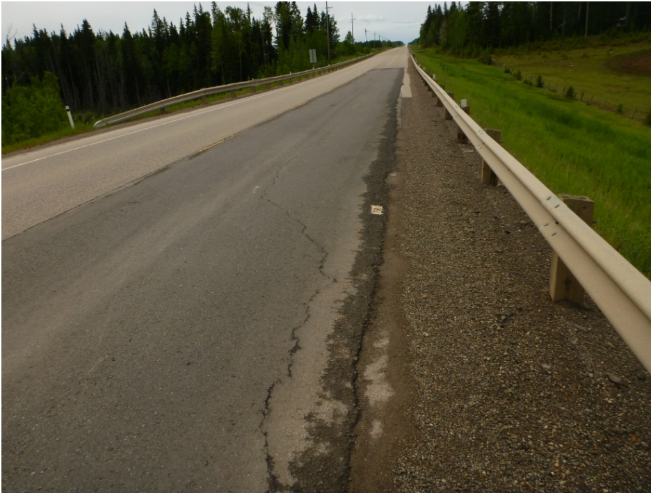
Photo 2 New pavement cracking (approximately 8 m in length) at the south end of the asphalt patch. Photo taken June 11, 2018 looking north.
