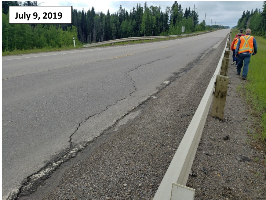
Photo 1 Pavement cracking in asphalt patch appears to have expanded. Photo taken July 9, 2019 looking south. (Photo from 2018 inspection included for comparison)
