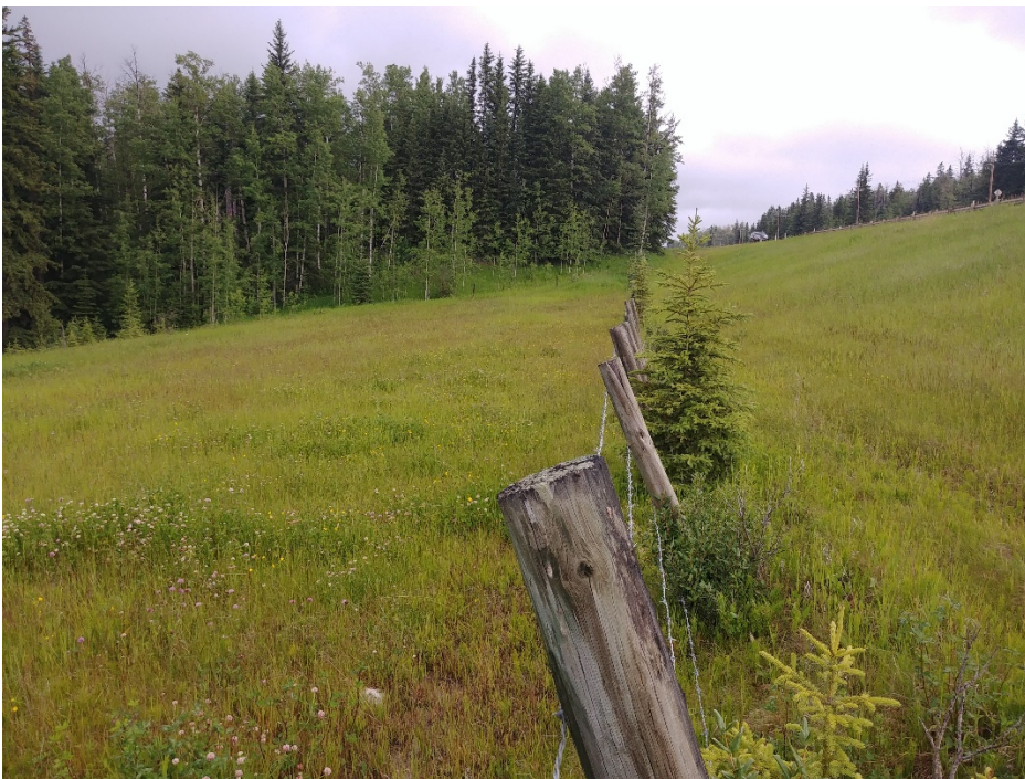
Photo 3 The fence line at the toe of the slide is deflected but shows little change since 2018 inspection. Photo taken July 9, 2019 looking north.
