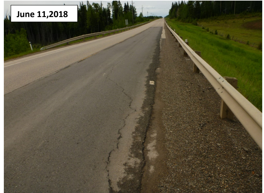
Photo 1 Pavement cracking in asphalt patch appears to have expanded. Photo taken July 9, 2019 looking south. (Photo from 2018 inspection included for comparison)
