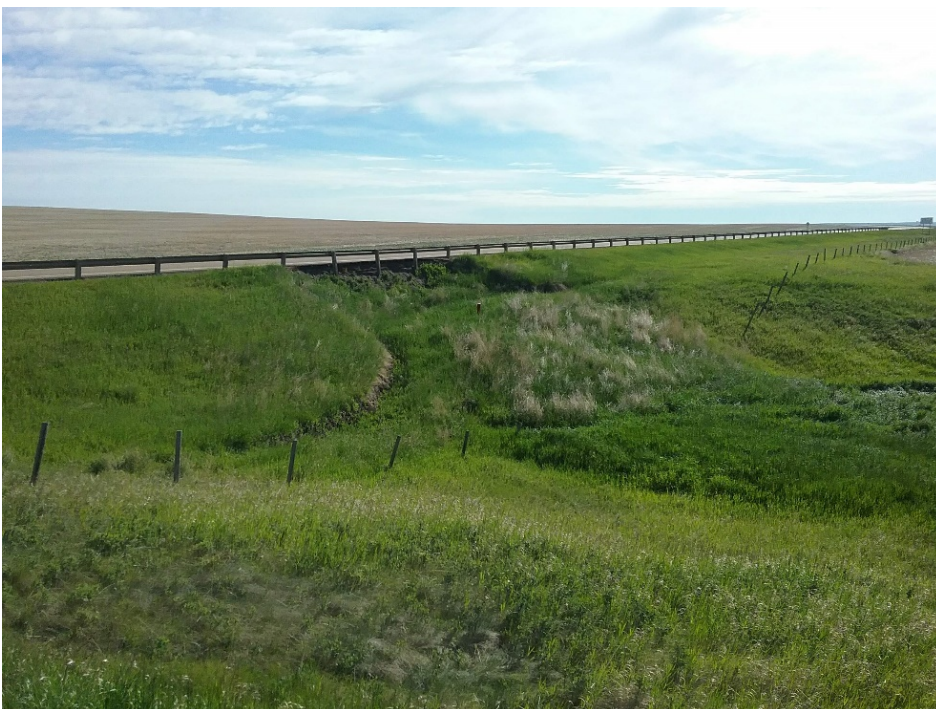
Photo 4 View of the C070W slide area. No discernible movement of the backscarp was observed. Three guardrail posts remain unsupported. Photo taken June 13, 2018 looking northeast.
